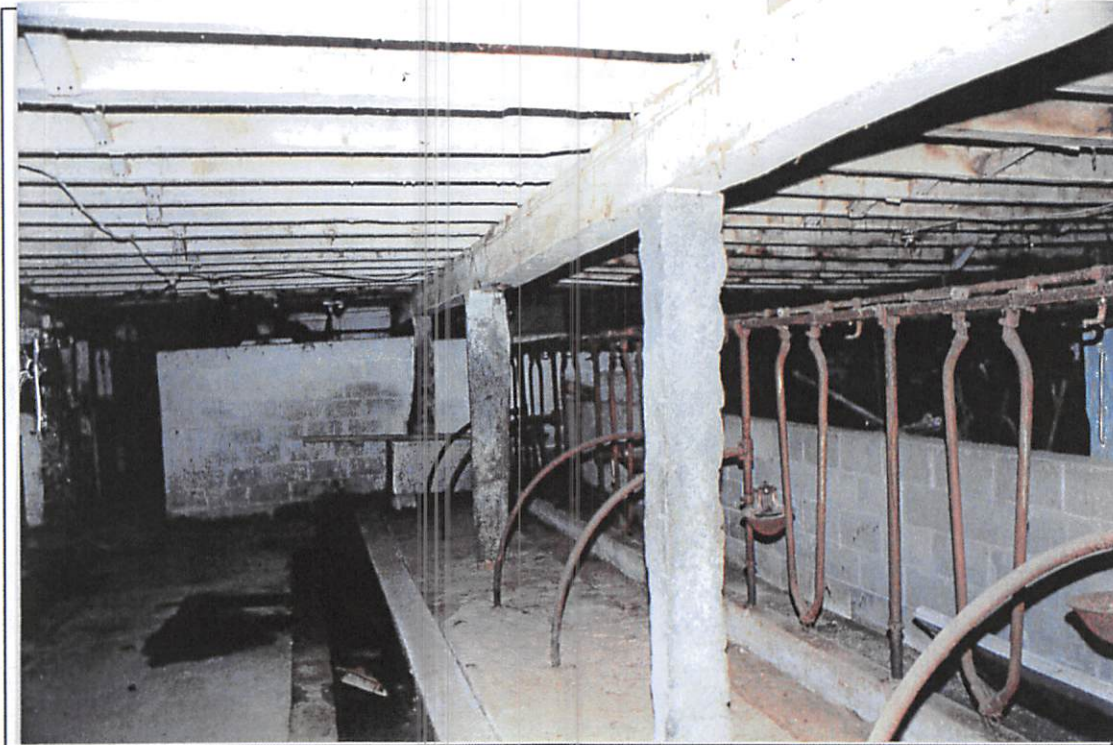
Photo # 7 Description: Replaced Columns (Before) Photo 7 Baseline 100
