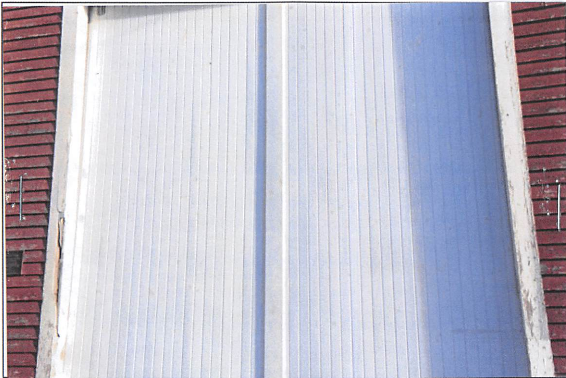
Photo # 14 Description: West Entrance Barn Door (After) Photo 14 Replacement Door:
