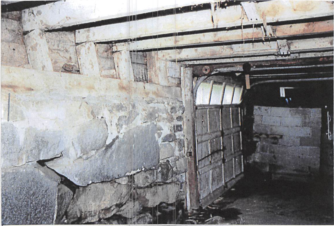
Photo # 3 Description: Northwest Wall (Before) Reference Photo 3 Baseline 62:
