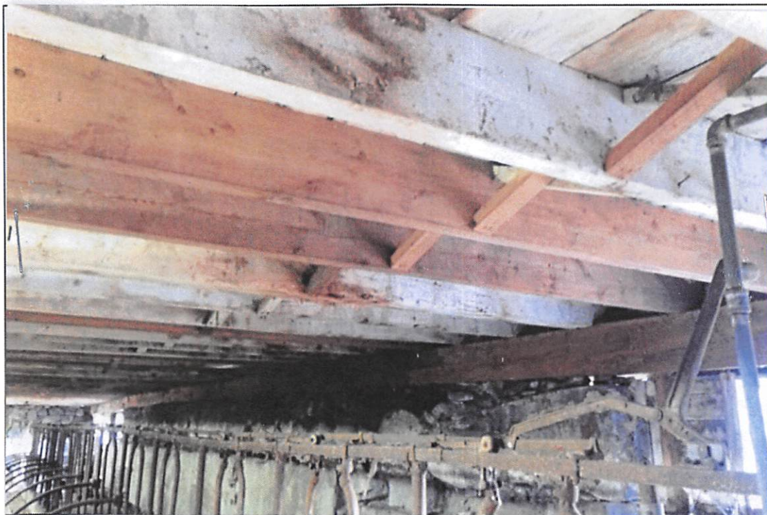
Photo # 6 Description: South Wall Sill Replacement (After) Photo 6 Sill Replacement:
