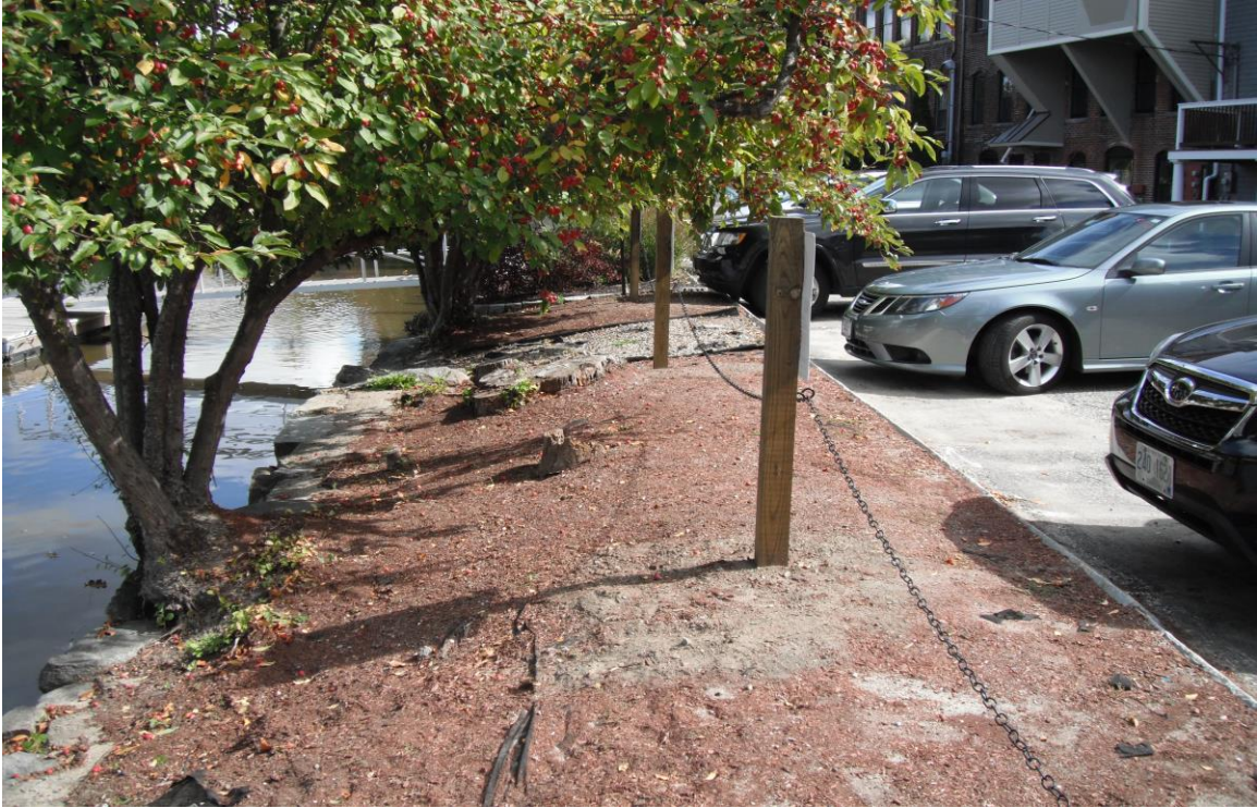
Photo 7: Facing easterly along existing retaining wall and adjacent parking lot.
