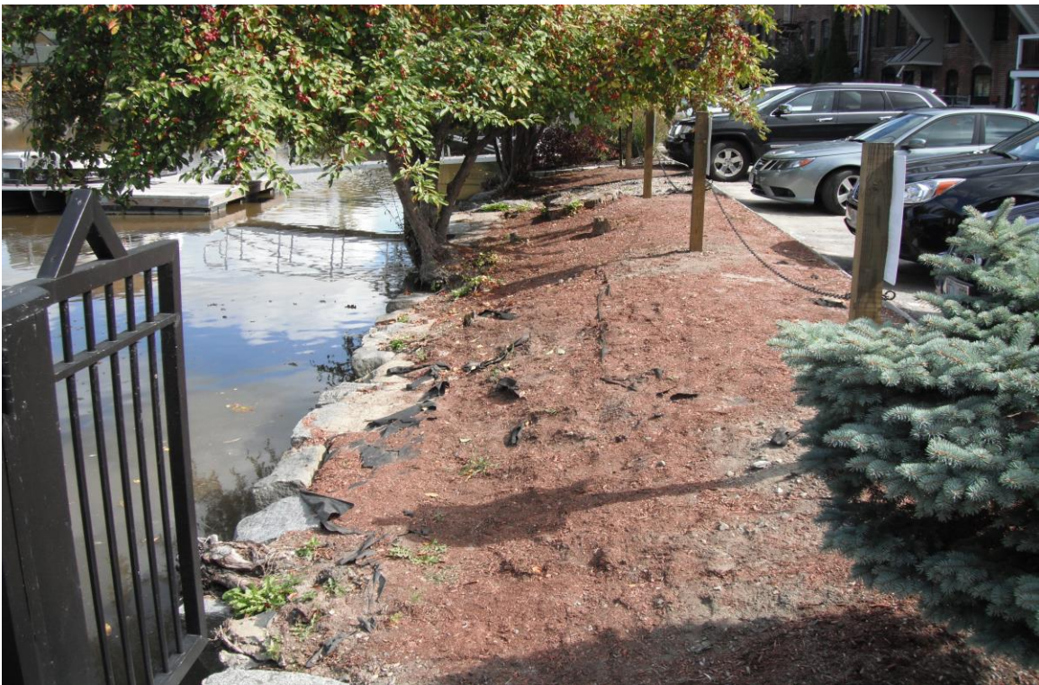
Photo 2: Facing easterly along existing retaining wall.
