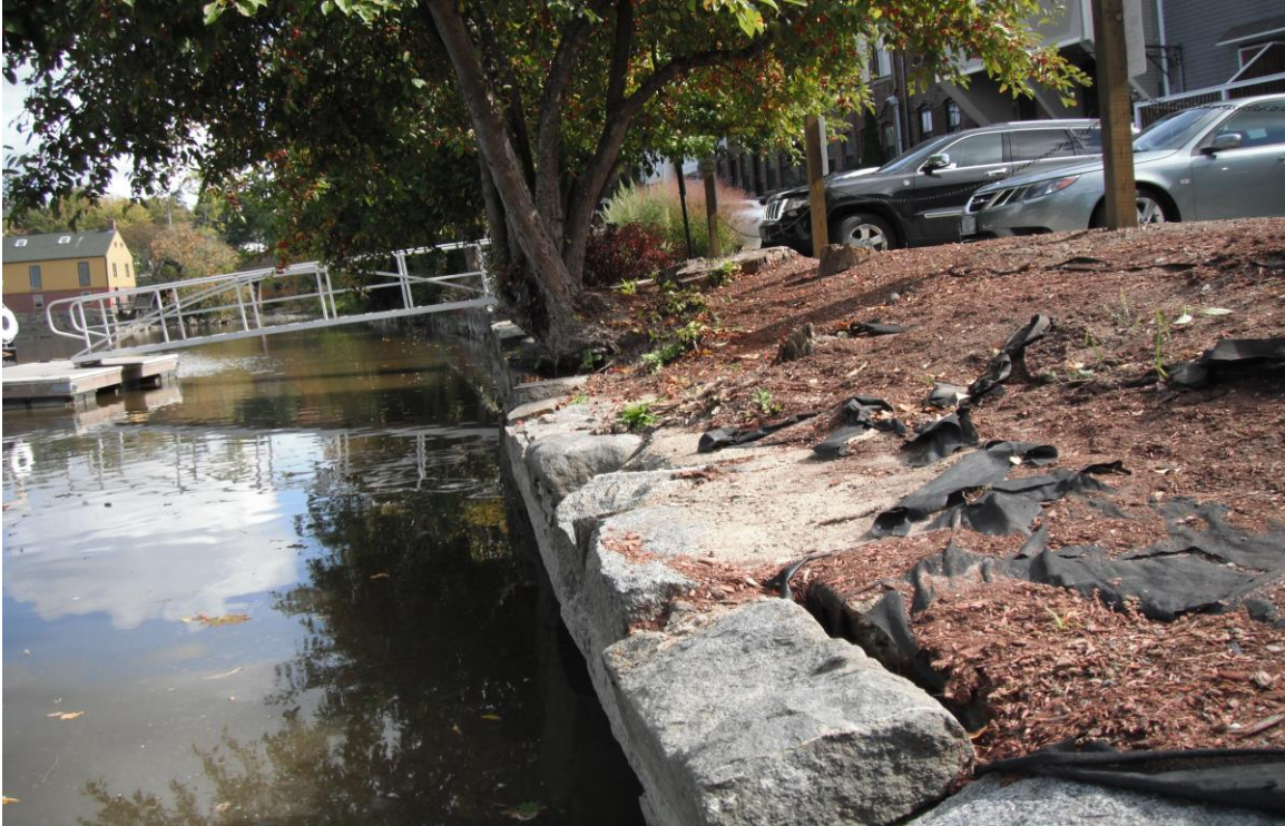
Photo 3: Facing easterly along existing retaining wall.
