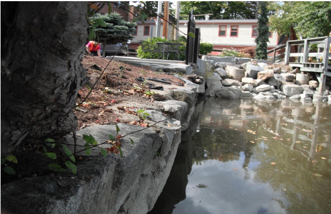
Photo 4: Facing westerly along existing retaining wall.
