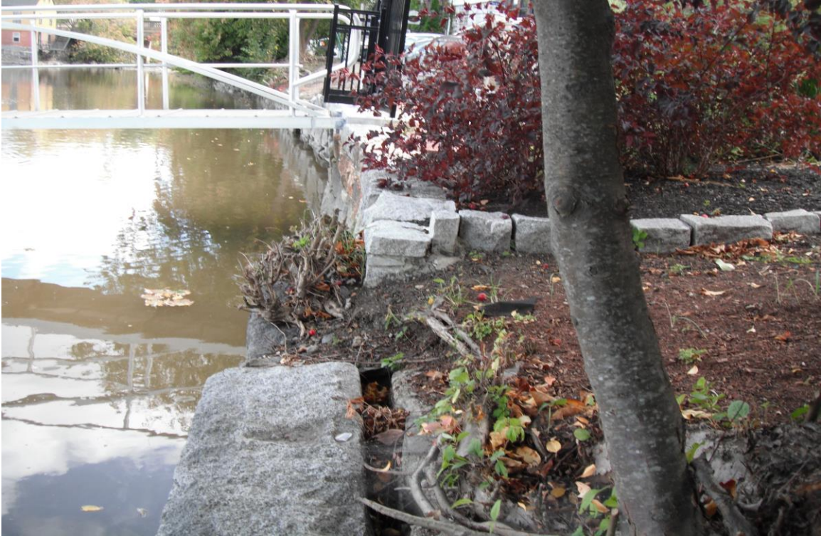
Photo 5: Facing easterly along existing retaining wall toward abutting parcel.
