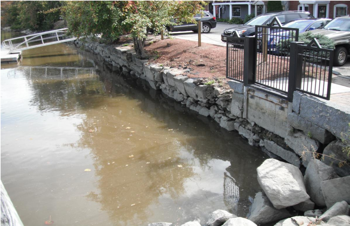
Photo 1: Facing easterly toward existing retaining wall.
