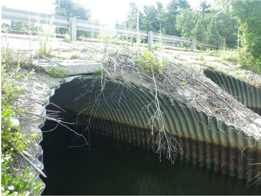
Photo 3: Linden Street Culvert (from upstream)
