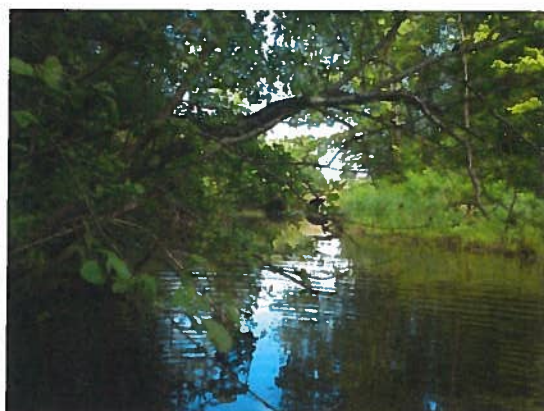
View looking westerly toward the Court Street culverts.
