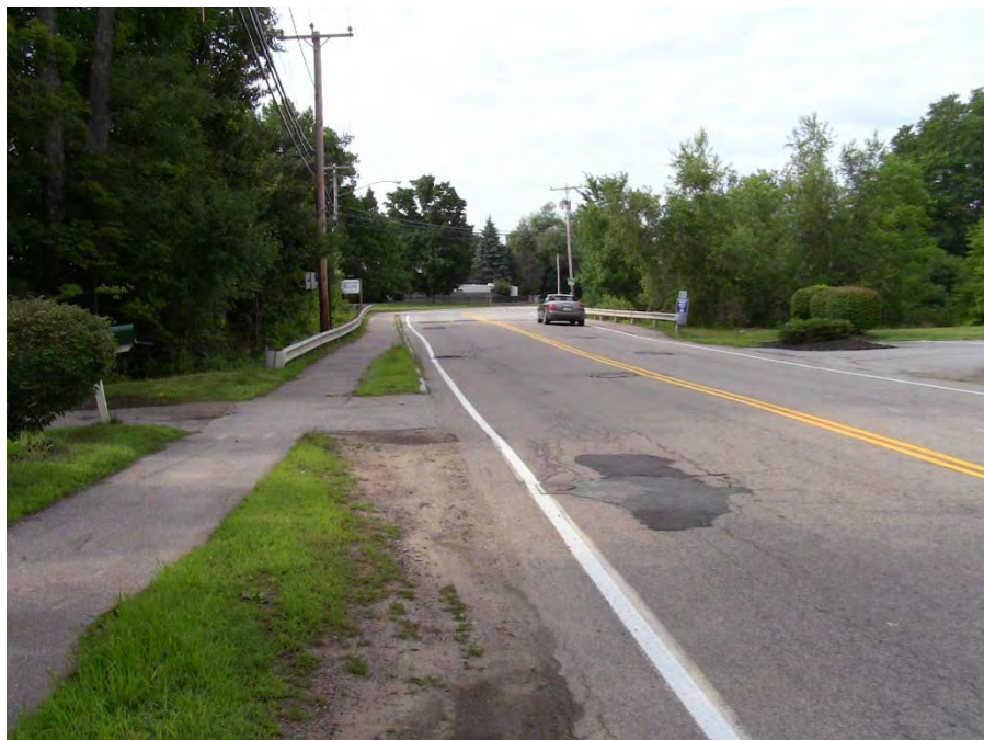
Photo 6: Court Street Culvert Approach (from north)
