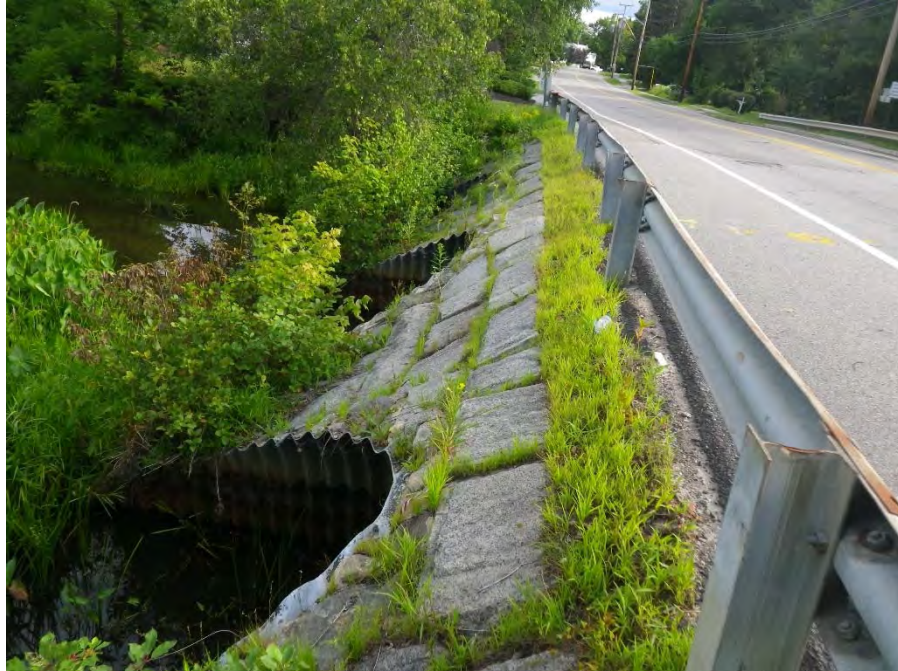
Photo 7: Court Street Culvert (upstream inlet)
