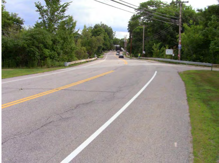
Photo 5: Court Street Culvert approach (from south)
