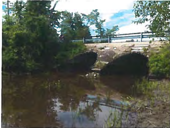
View of Linden Street culverts looking westerly.
