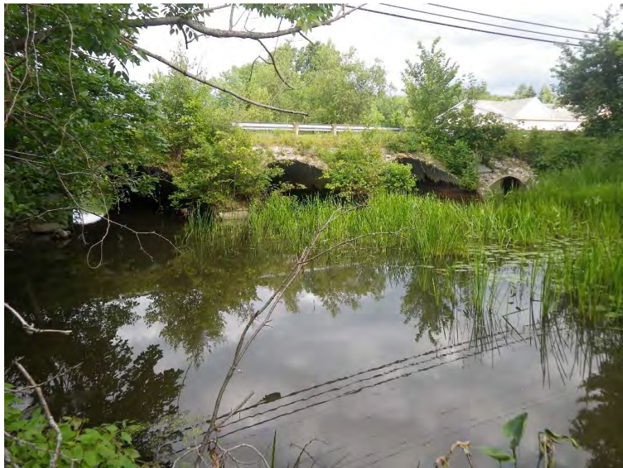
Photo 8: Court Street Culvert (from downstream)
