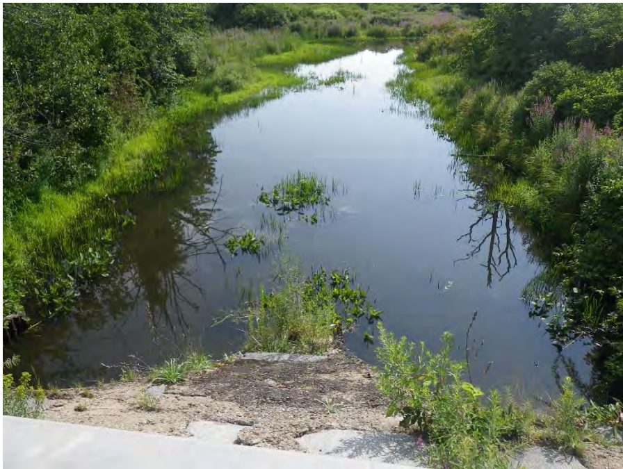
Photo 4: Linden Street Culvert (looking downstream)
