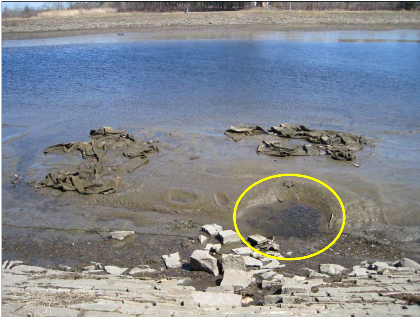
Picture 2. View from Swasey Parkway looking east across the Squamscott River. The buried stormwater outfall/ plunge pool is highlighted in yellow. The absorbent mats at the site are also visible.
