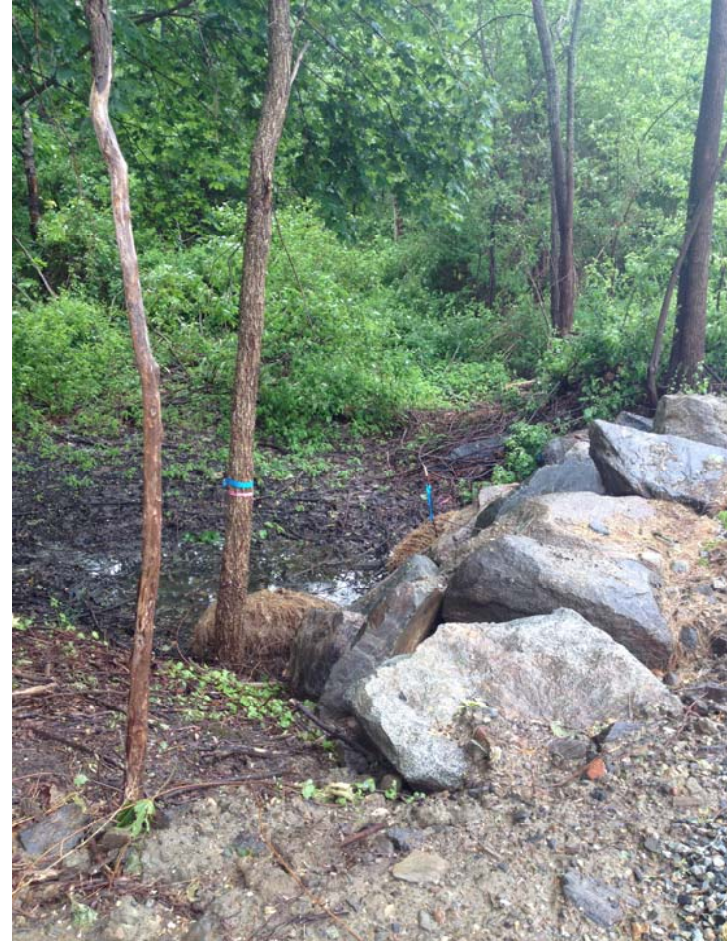
Photograph 2. View looking southwest at boulder wall in foreground and small Palustrine Forested Wetland in background; hay bales at toe of slope for erosion control.
