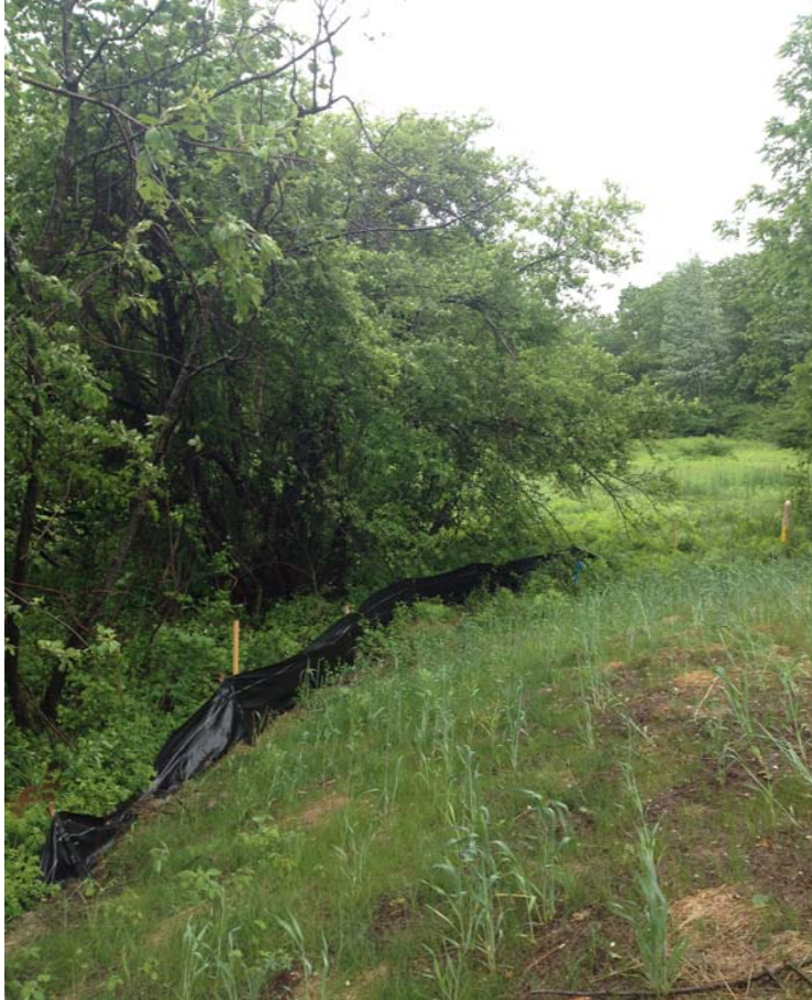
Photograph 3. View looking southwest at silt fence in buffer area adjacent to large wet meadow in background.
