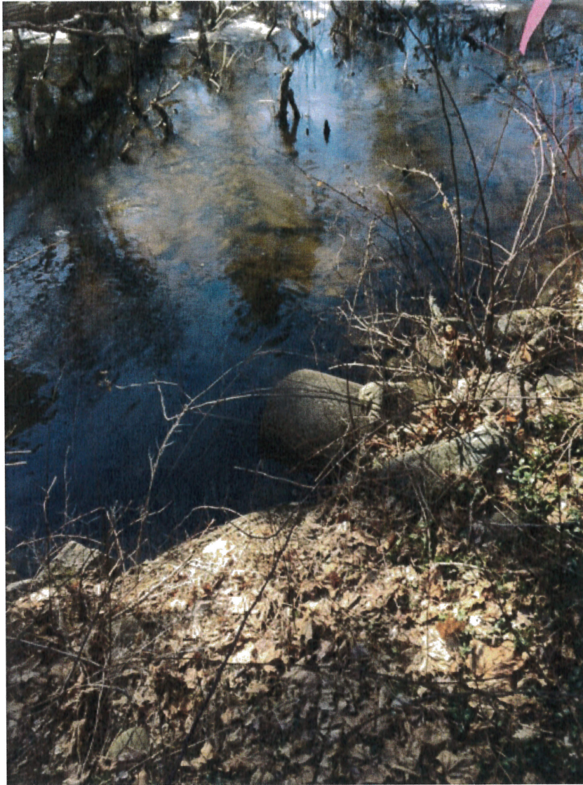
Photo #10 - Looking at the pipe outfall (February 2016).
