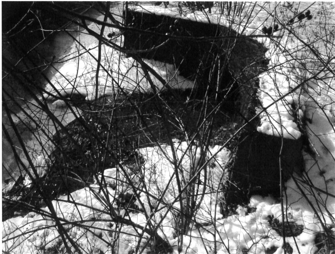
Photo #9 – Looking at existing outfall (January 2016).
