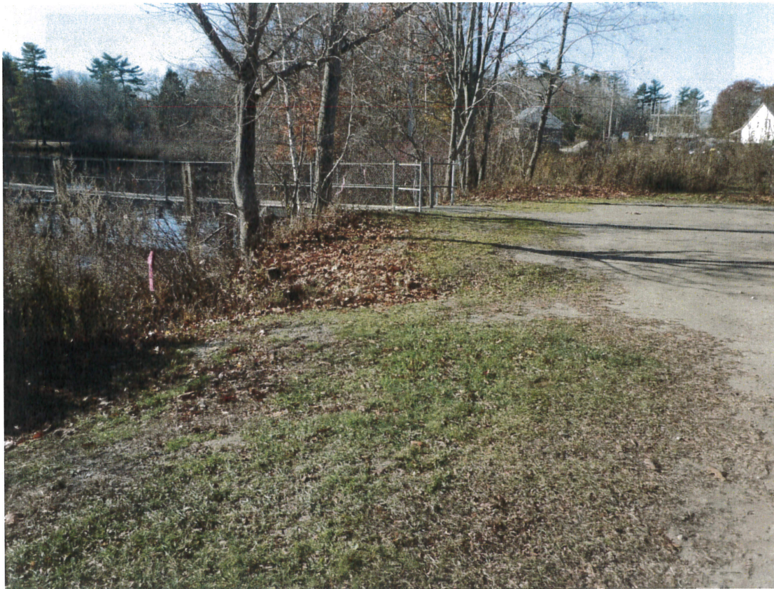
Photo #6 – Looking southwest at existing outfall (November 2015).
