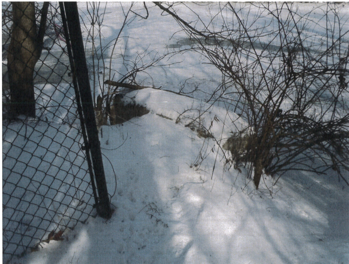
Photo #2 - Looking northeast at headwall of existing outfall (January 2016).
