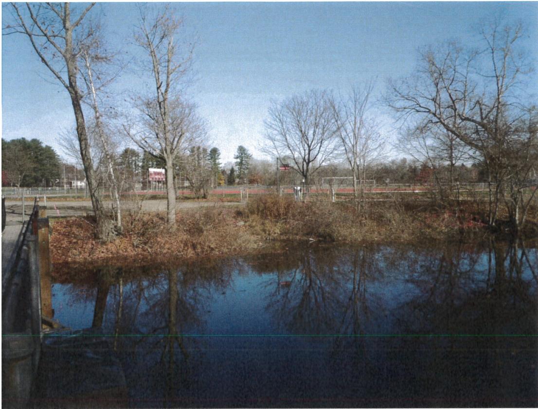
Photo #4 - Looking northwest at existing outfall (November 2015).
