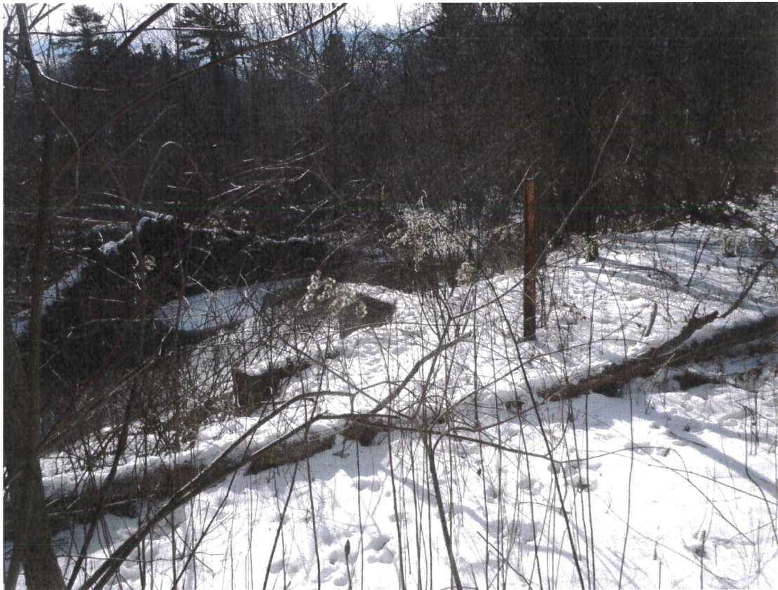
Photo #7 – At river edge, looking south at headwall of existing outfall (January 2016).
