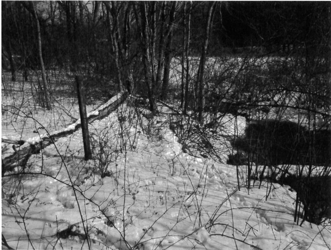
Photo #8 – At river edge, looking northeast at existing outfall (January 2016).
