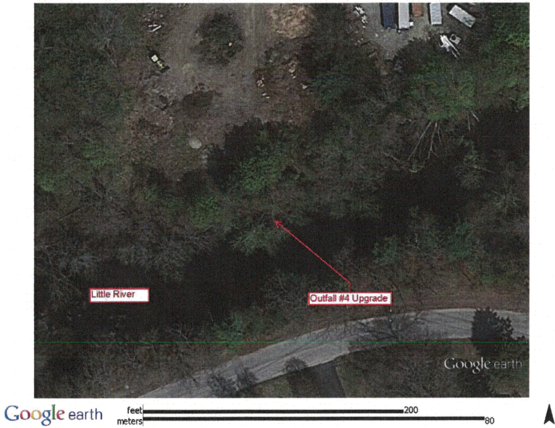
Aerial View of Outfall #4
