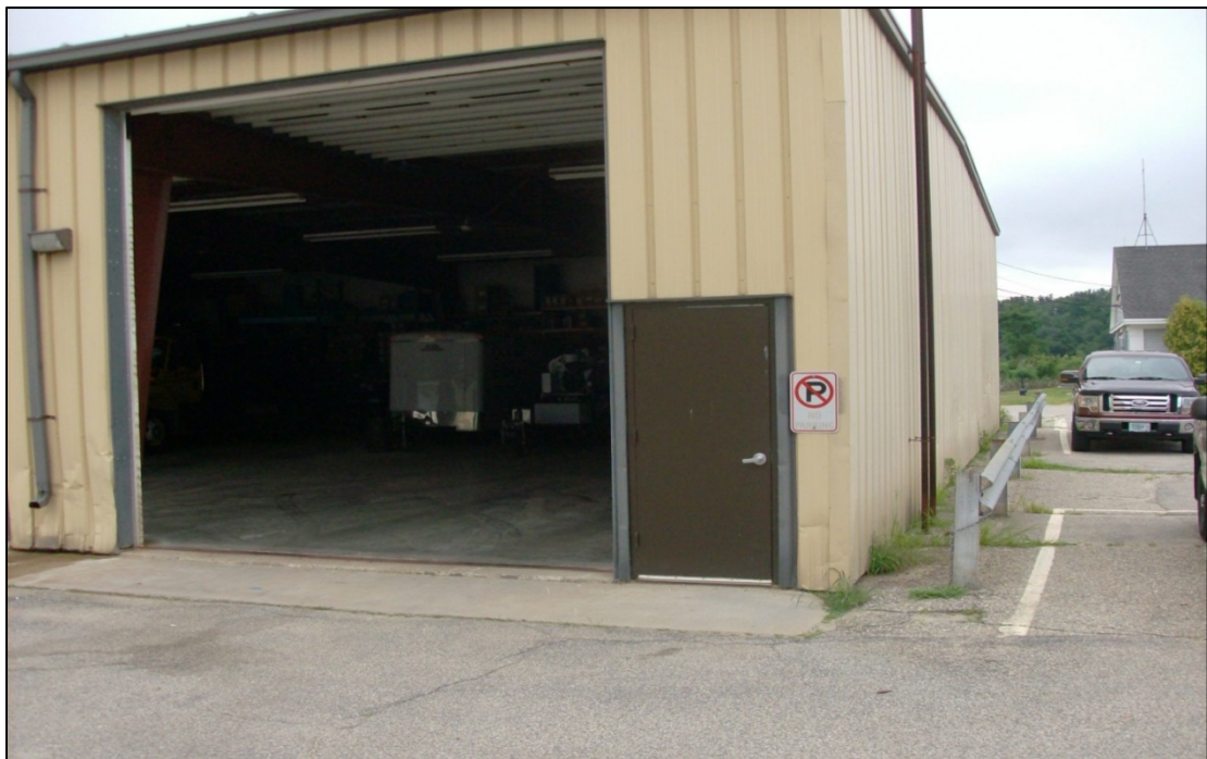
Pass door on west side of building.
