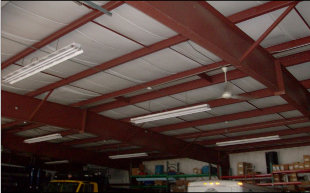
Typical metal framing.
