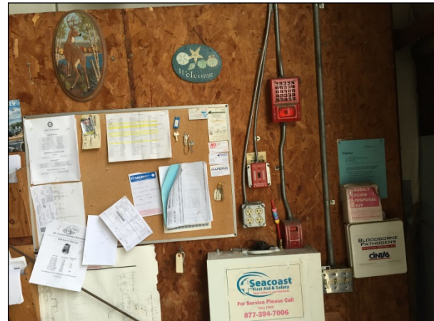
General Surface Mounted Outlet
