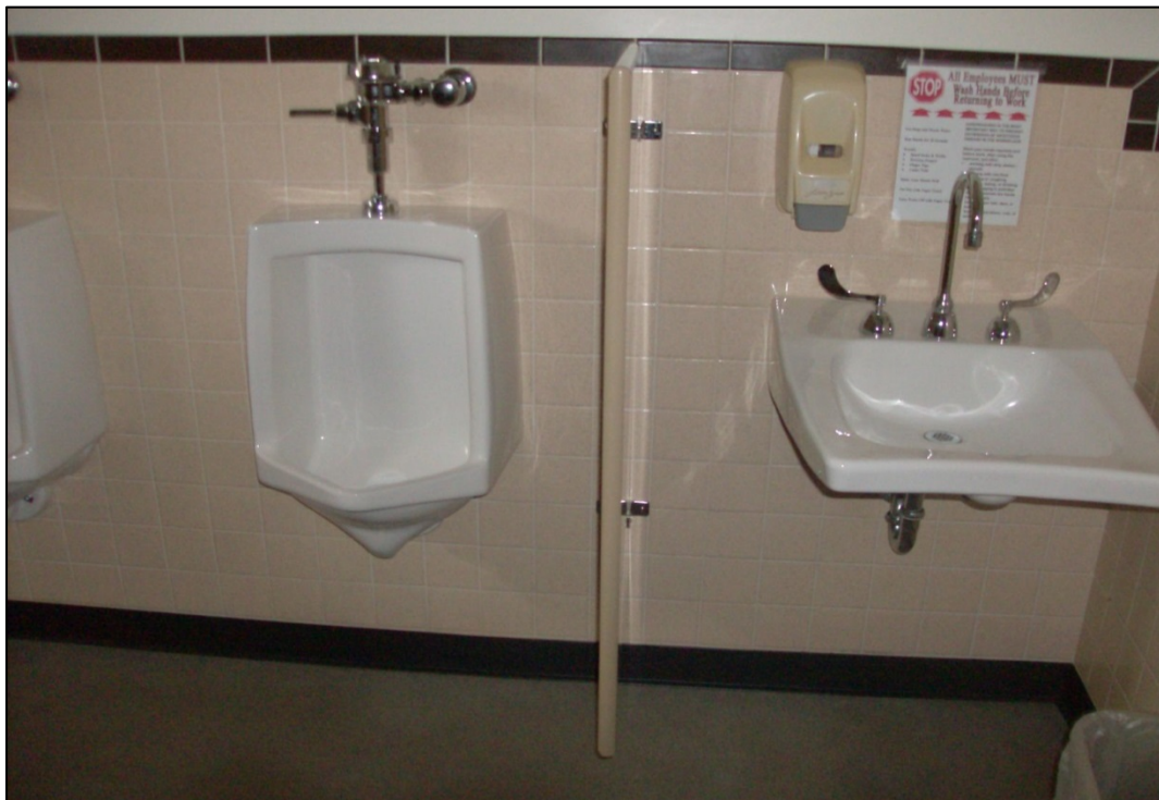
Men's Room with ADA accessible sink.
