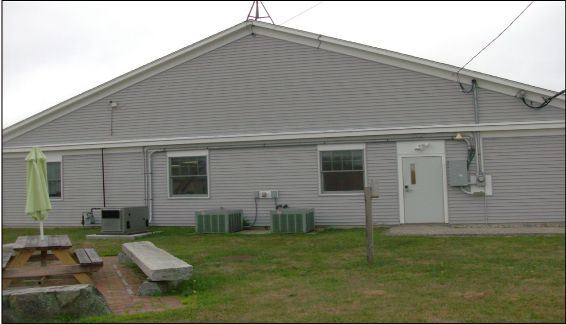
South side of building.
