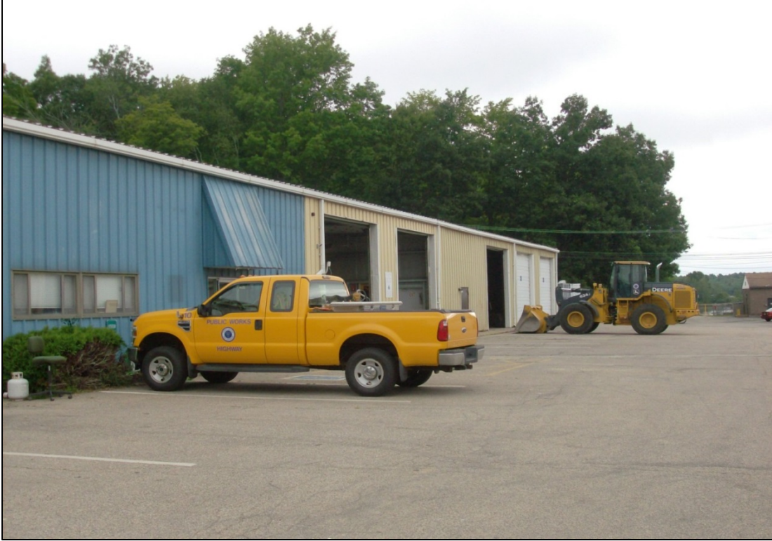
DPW Maintenance and Storage Garage looking east.
