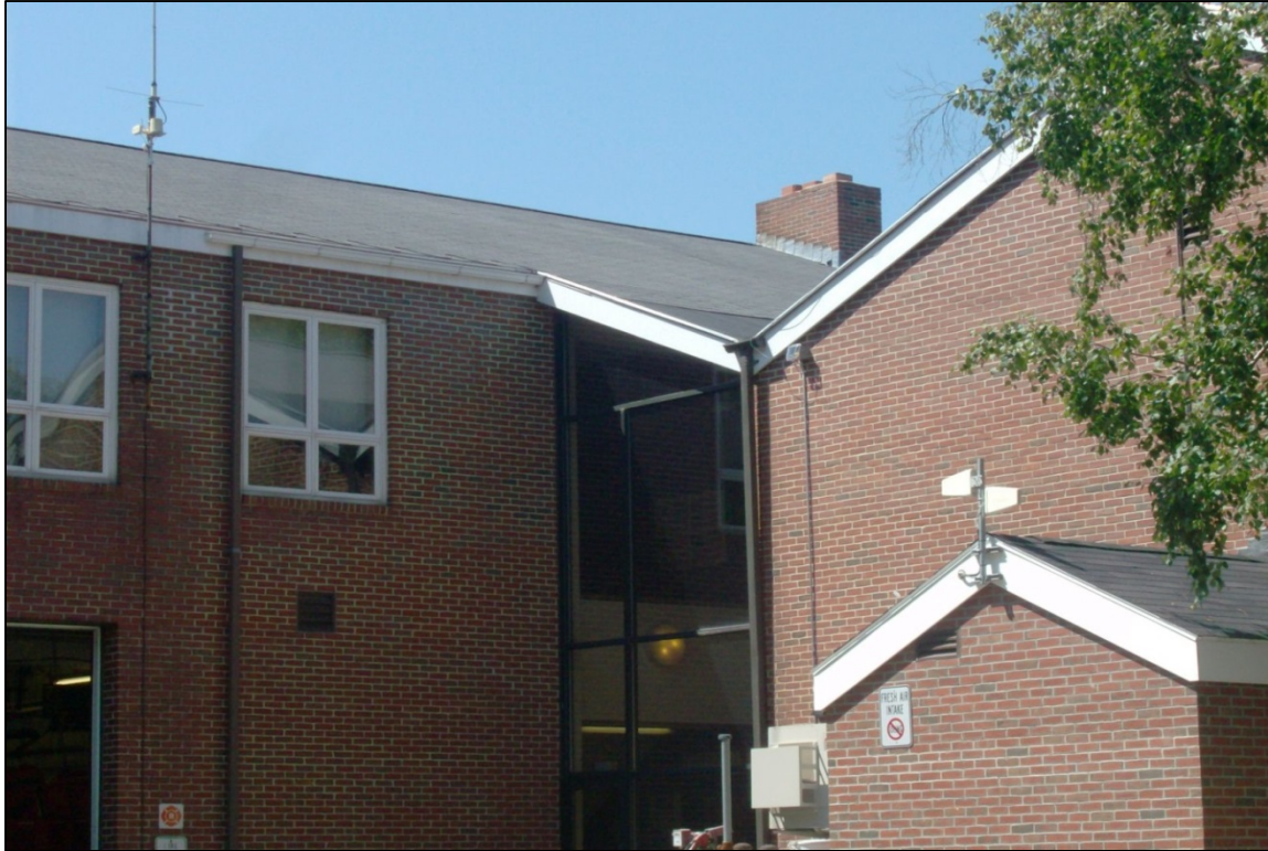
South edge of roof valley over central portion of building.
