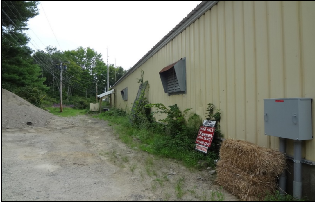
View along the rear of the DPW Garage and Storage Building.
