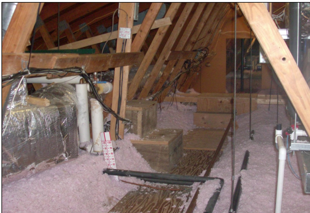
Attic area with ample blown-in insulation.
