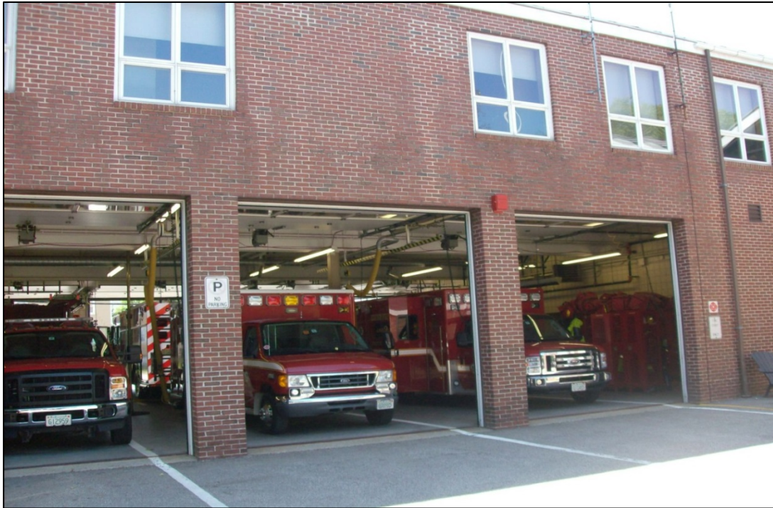
East side apparatus bays facing the rear parking lot.
