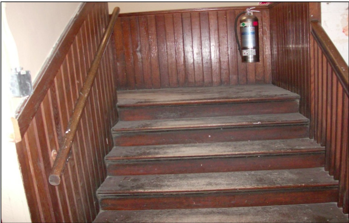
Wood stairs to second floor.
