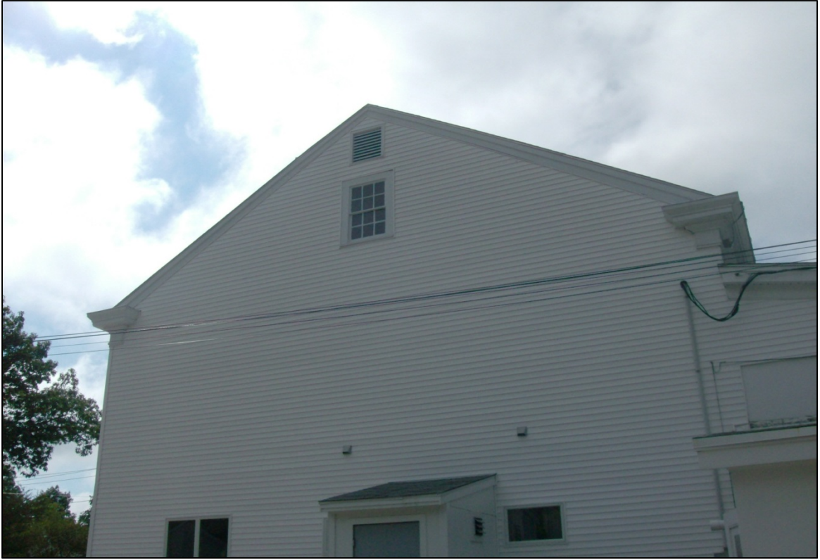
Back wall of the Senior Center.
