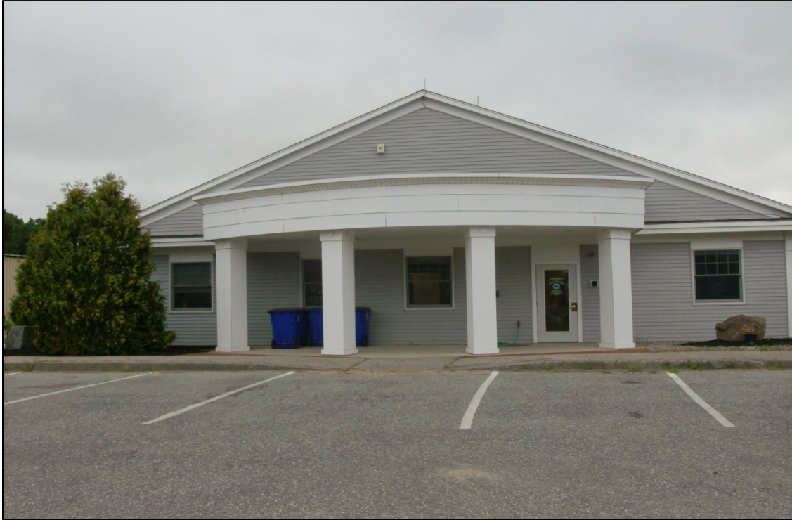
DPW Administration Office main entrance.
