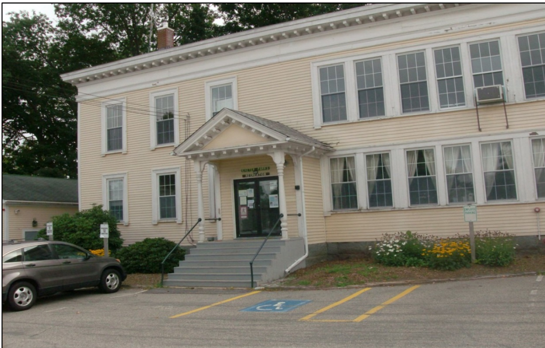
Main entrance from parking lot. Note handicap parking, but entrance is not accessible.
