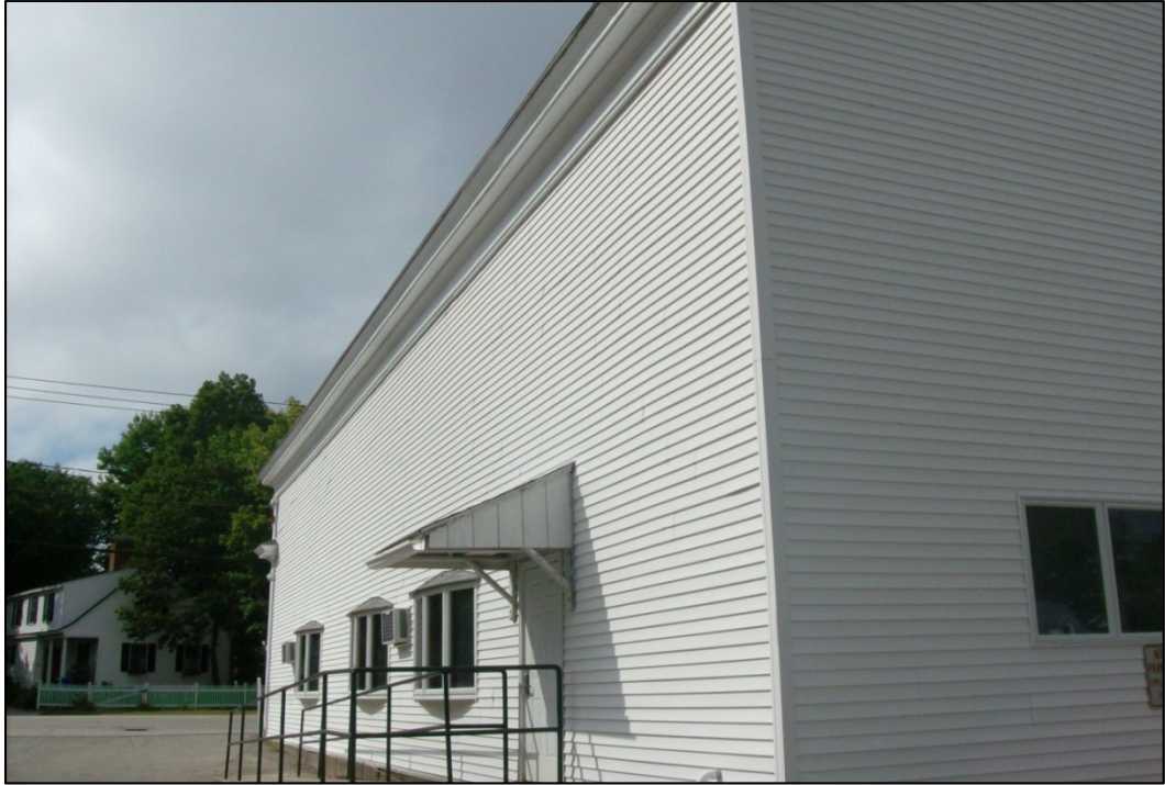
South wall of the Senior Center with ADA accessible ramp.
