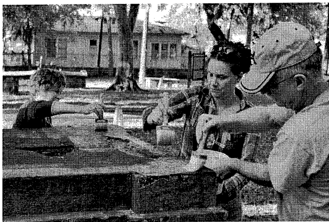
Figure 23. Limewash is a breathable coating sometimes used to protect the surface of the grave marker and provide a decorative finish. Limewash is applied by brush in five to eight thin coats (with each coat about the consistency of skim milk). The surface is allowed to slowly dry between coats. Sometimes the surface is covered by damp burlap to slow the drying process. Photo: Sarah Jackson.
