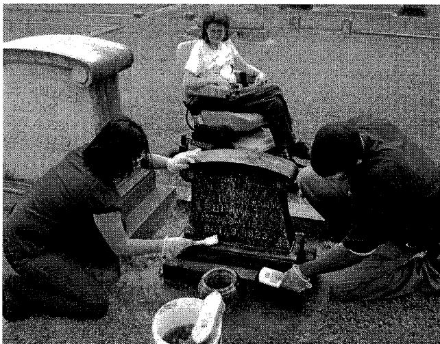
Figure 17. Volunteers can undertake cleaning of grave markers once they have received initial training. Cleaning methods may include wetting the stone, using a mild chemical cleaner, gently agitating the surface with a soft bristle brush, and thoroughly rinsing the marker with clean water. Photo: Jason Church.
