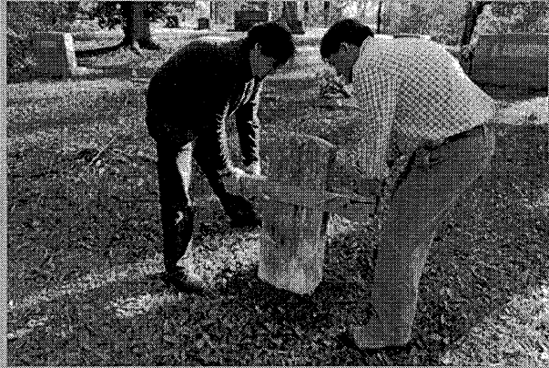
Figure E1. The simple wooden clamp system allows two people to safely lift a marble grave marker. Photo: Sarah Jackson.
