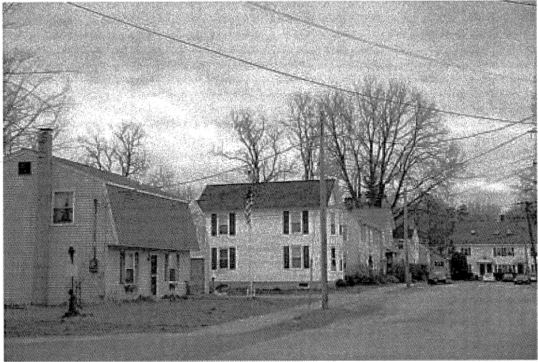
Photo 56) 17 South St., 15 and 11-13 South
