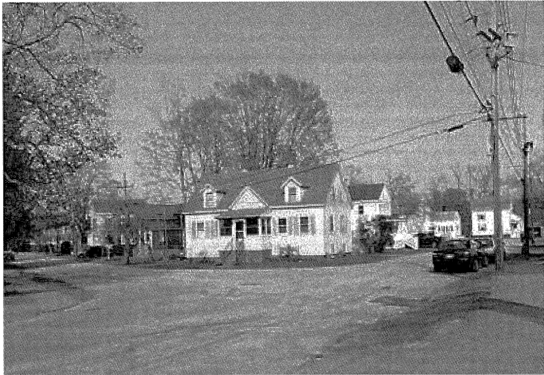
Photo 68) South St. and River St. Ext., 34-36 South center, River St. right rear
