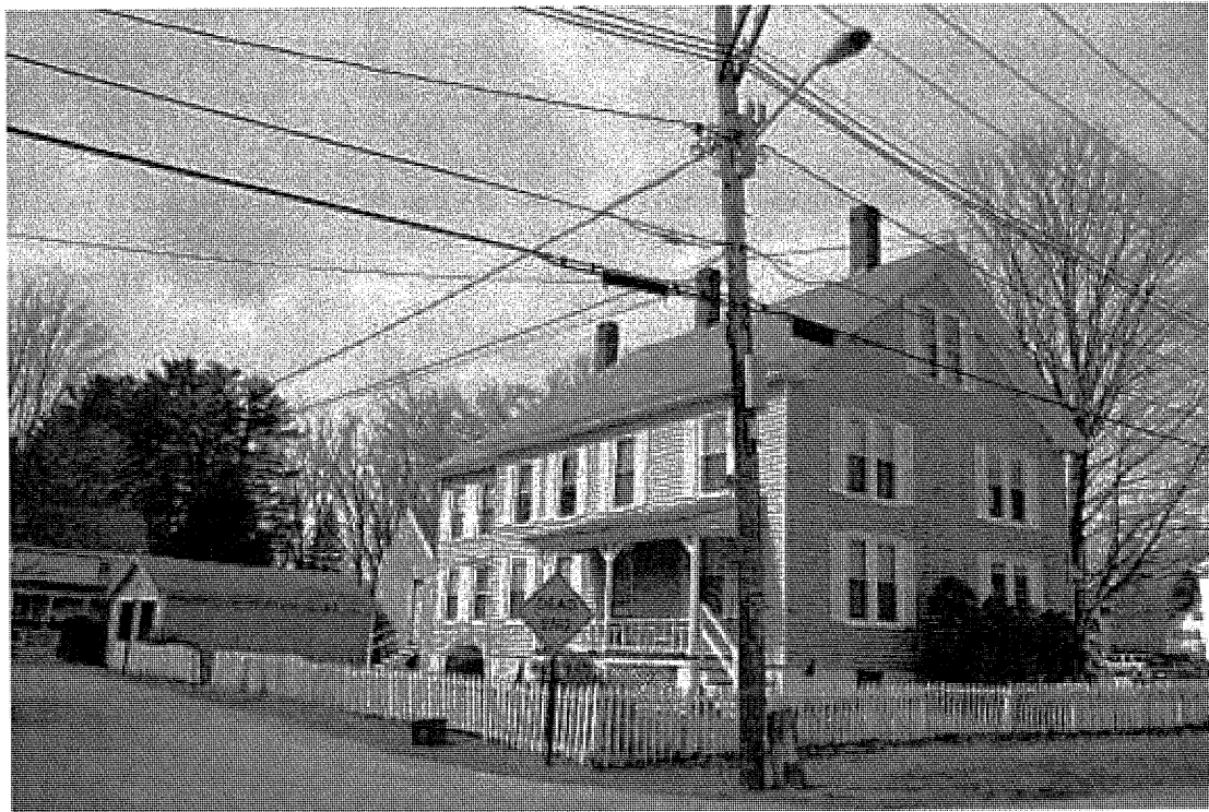
Photo 76) 38-40 South St. side elevation and garage
