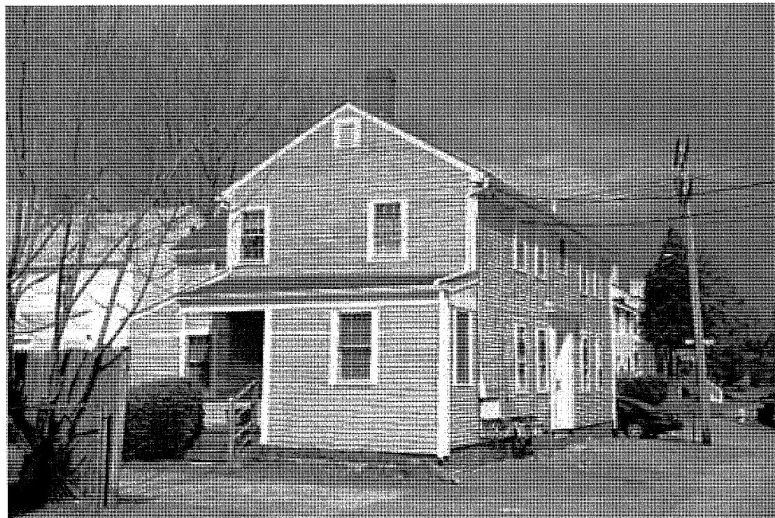
Photo 25) 39 Franklin St., rear and gable end
