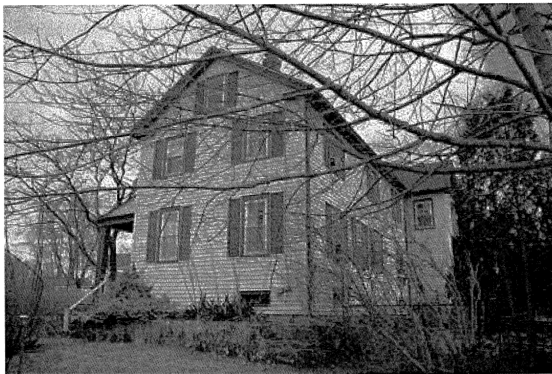
Photo 92) 12 River St. end and rear elevations
