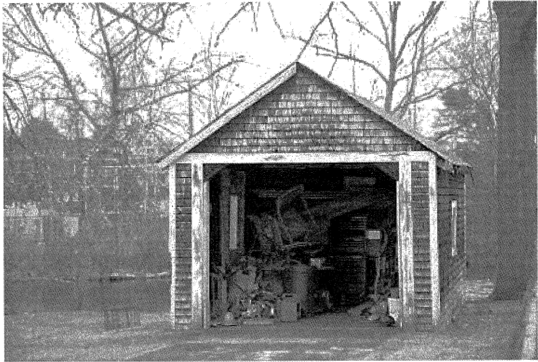
Photo 101) 22 River St. garage
