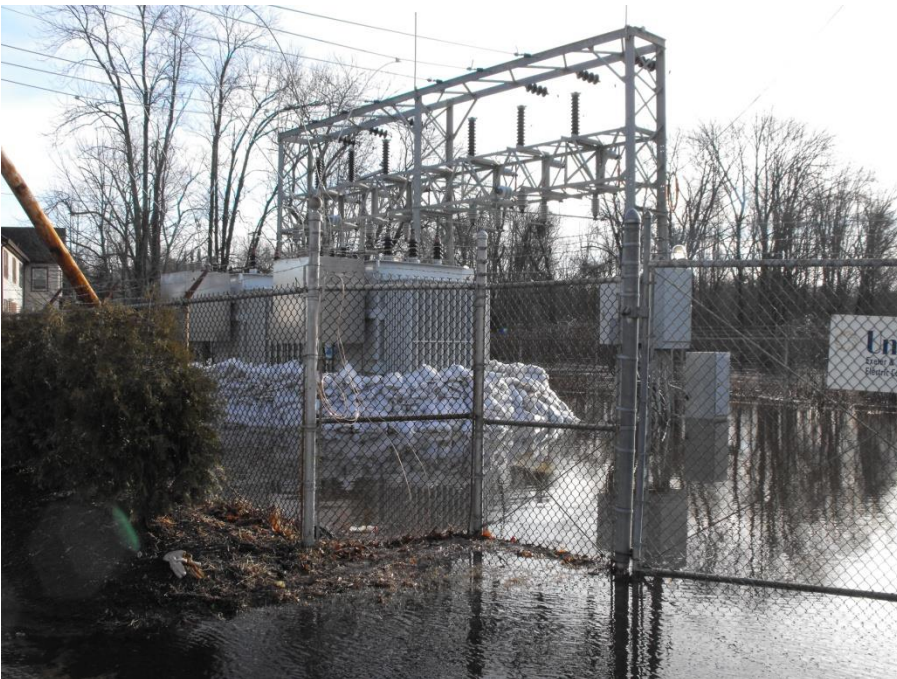
3-16-2010: Utilil Sub-Station on the Exeter River
