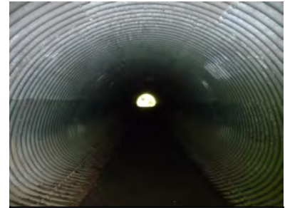
Trail to The Oaklands through the Route 101 underpass culvert.
