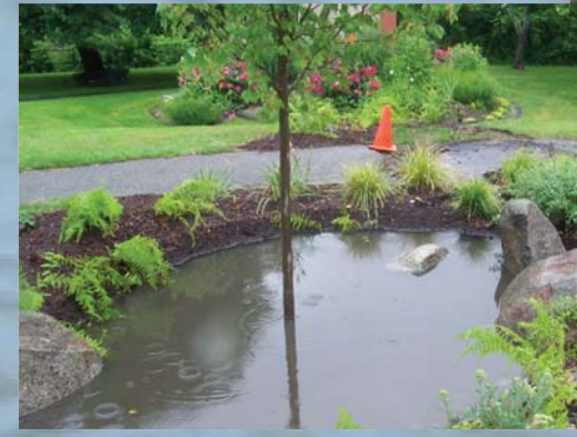
Images of the first rain after the curb cut and installation of the rain garden. Stormwater flowing down Chestnut Street is diverted to the rain garden. Before, stormwater flowed to a nearby catch basin and discharged untreated, directly into the Exeter River.
