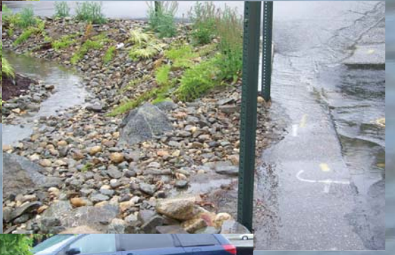
Images of the first rain after the curb cut and installation of the rain garden. Stormwater flowing down Chestnut Street is diverted to the rain garden. Before, stormwater flowed to a nearby catch basin and discharged untreated, directly into the Exeter River.
