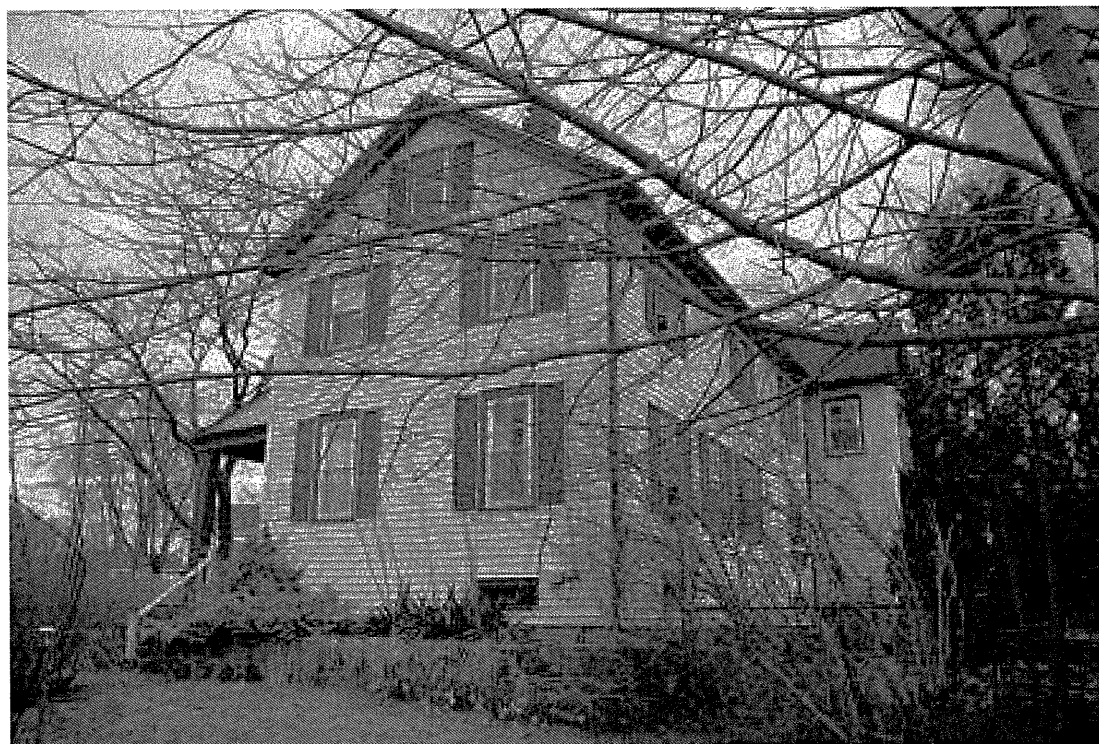
Photo 92) 12 River St. end and rear elevations
