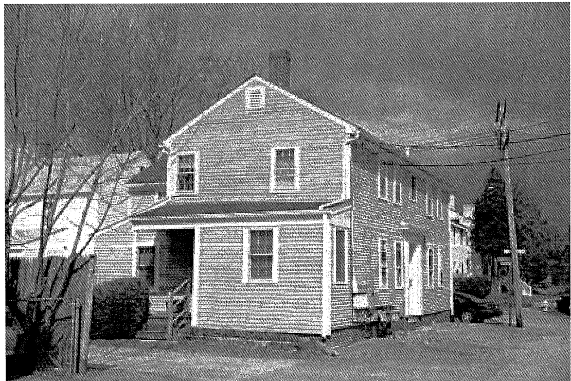
Photo 25) 39 Franklin St., rear and gable end
