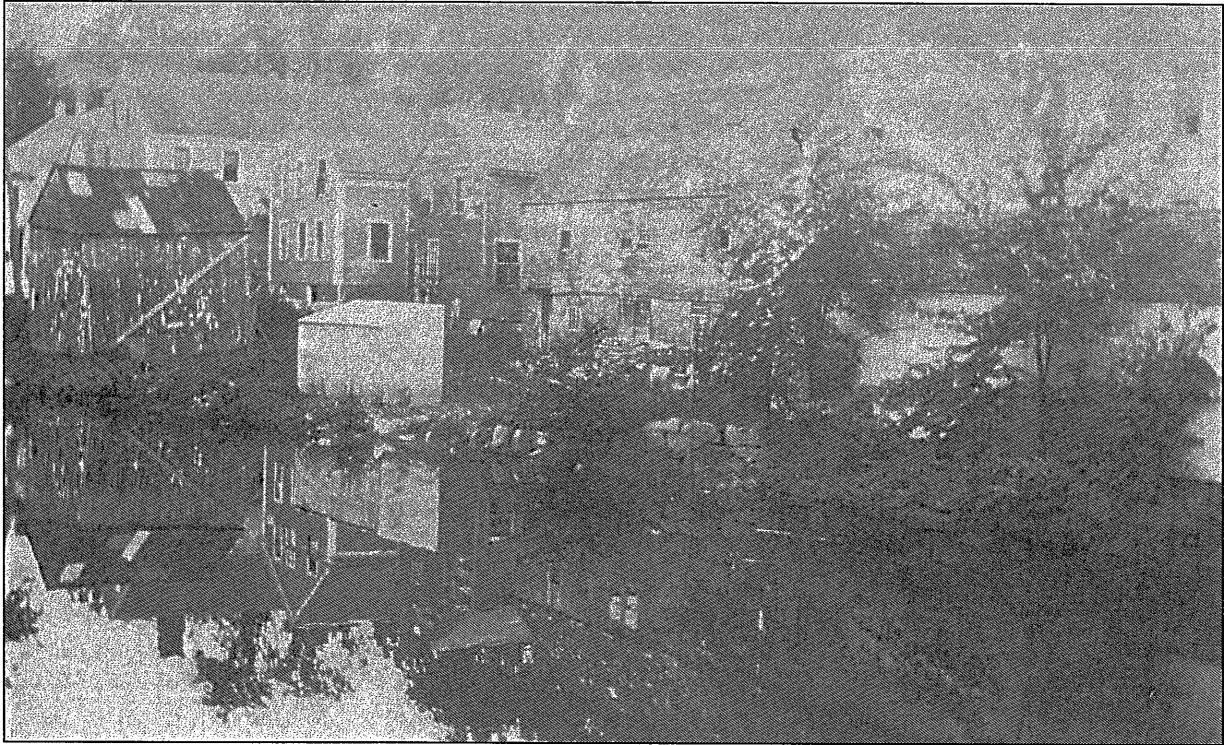
Franklin Street riverfront. Rear of 24-26 Franklin left rear. Three houses site of 20 Franklin not extant.
