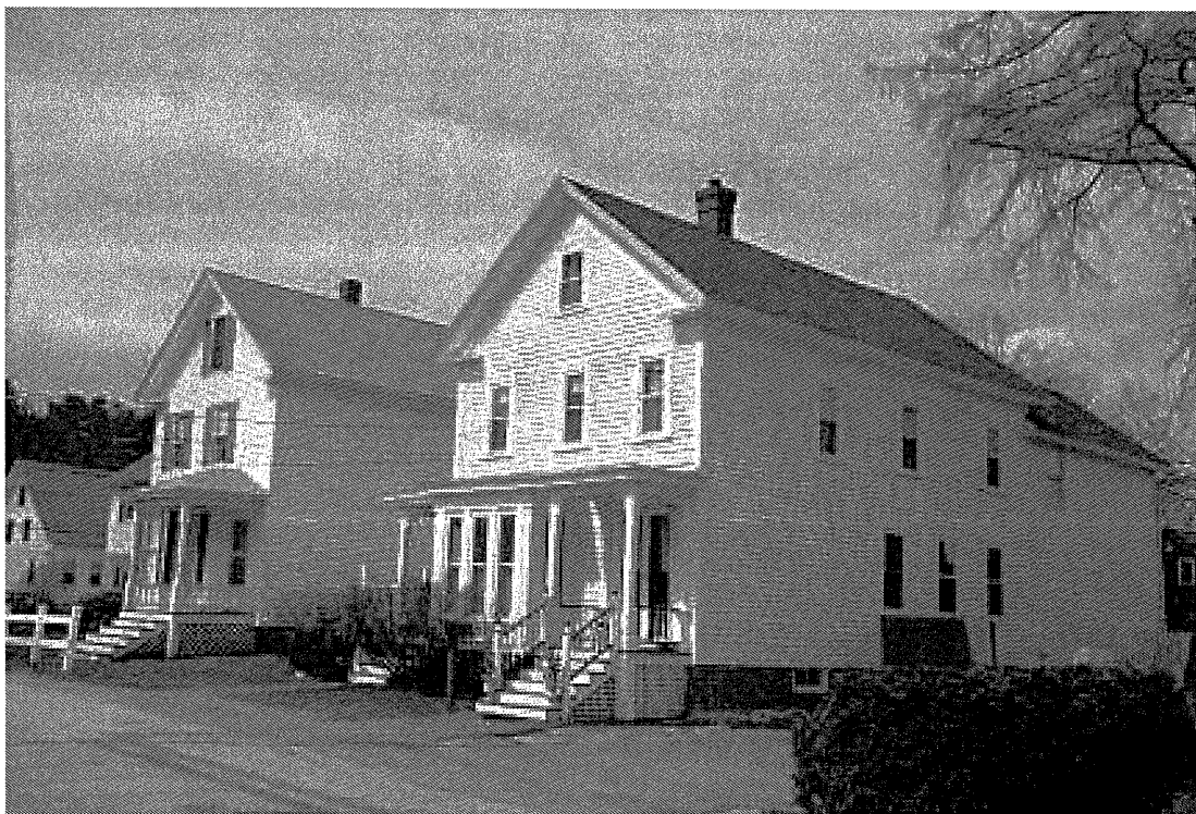
Photo 94) River St., 17 River right, 19 River left
