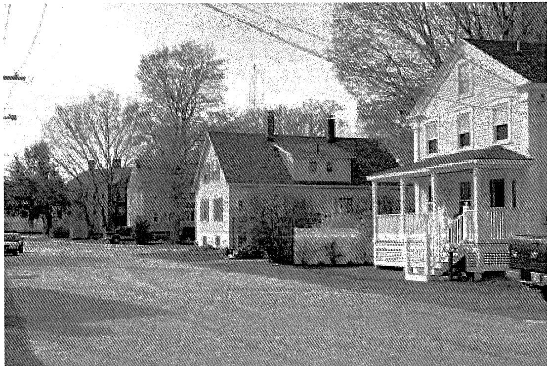
Photo 69) South St. from River St. Extension, 8 River Street Ext. at right, 41-43, 34-36 South left
