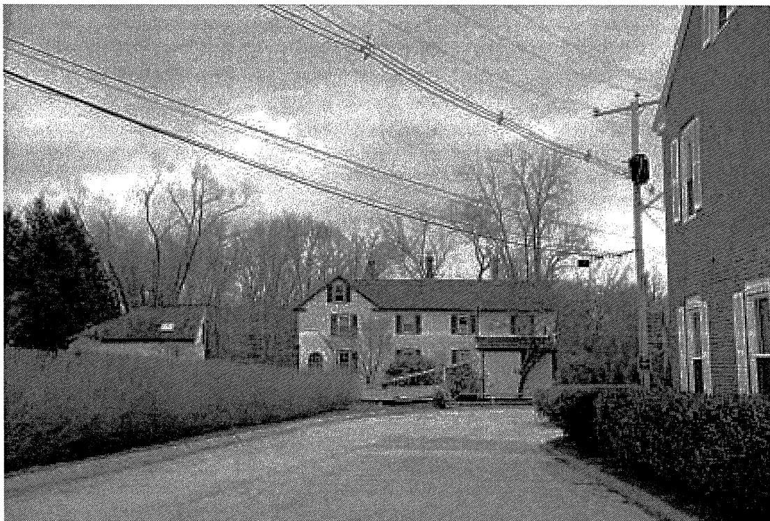
Photo 90) 12 River St., from South St.
