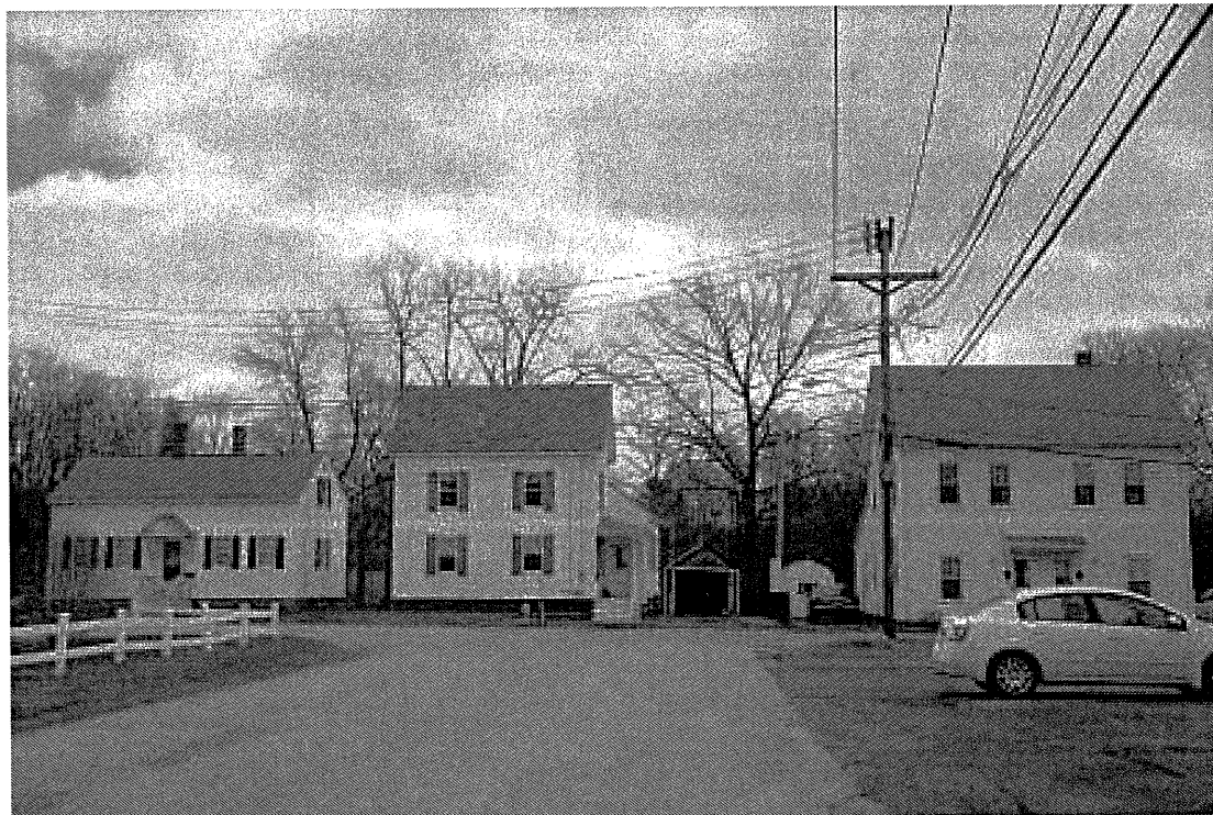
Photo 98) River St. opposite River St. Ext. 20, 22 and 24-26 River
