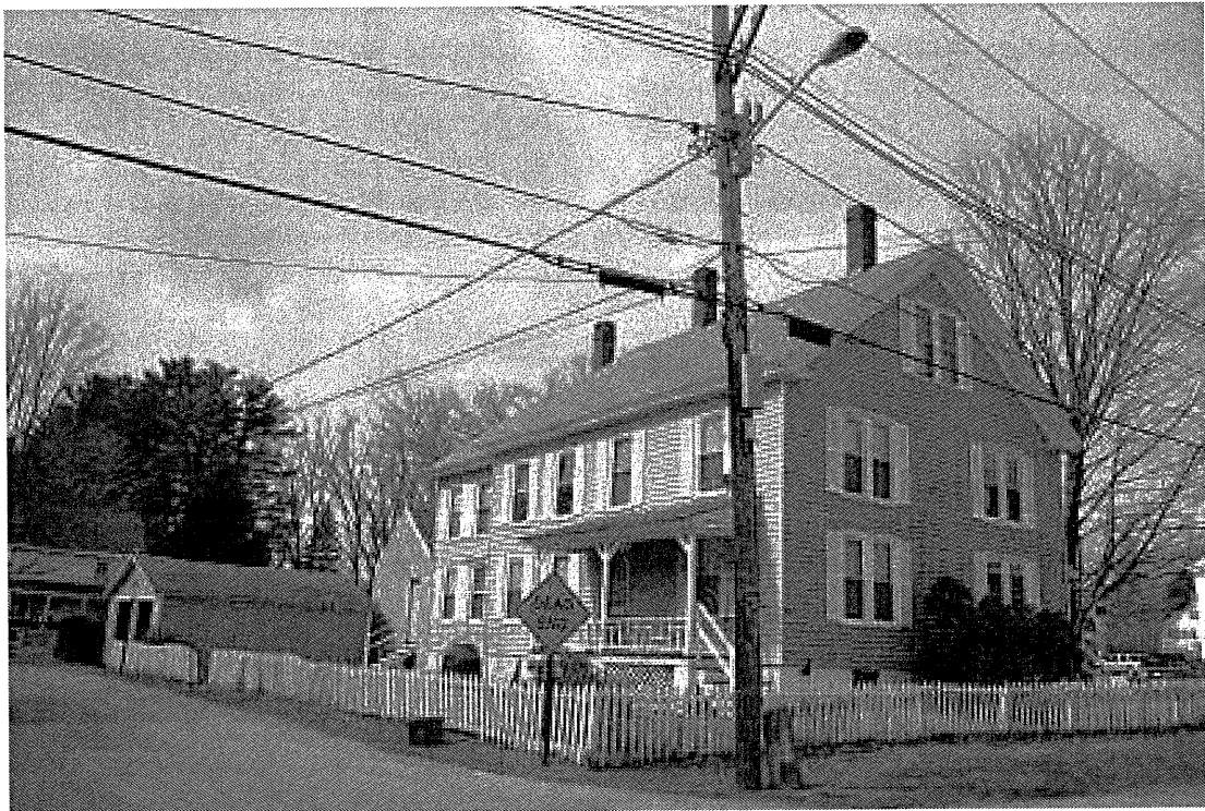
Photo 76) 38-40 South St. side elevation and garage
