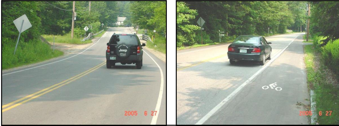
Left: Kingston Road with no shoulders. Right: Newly recently constructed shoulders on Hampton Road.
