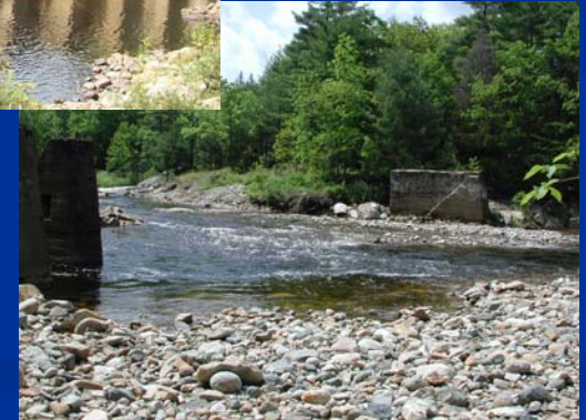
Bearcamp River Dam - Tamworth, NH
