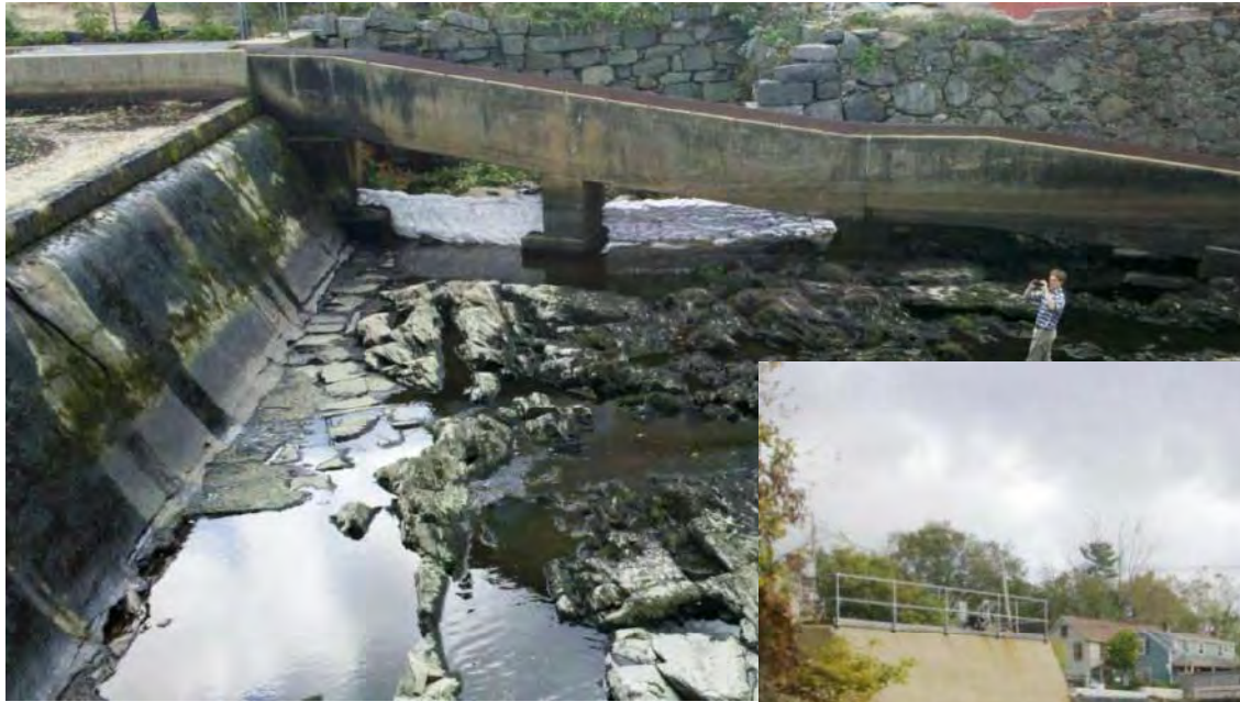
Dam & fish ladder, Nov 2011
