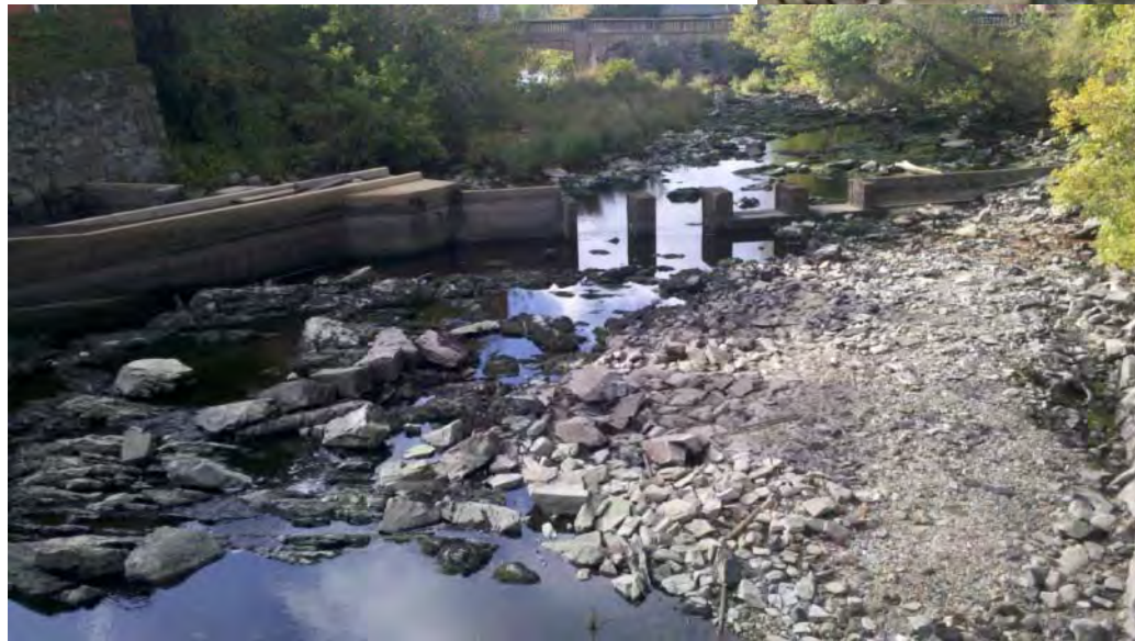
Fish ladder & weir, Nov 2011
