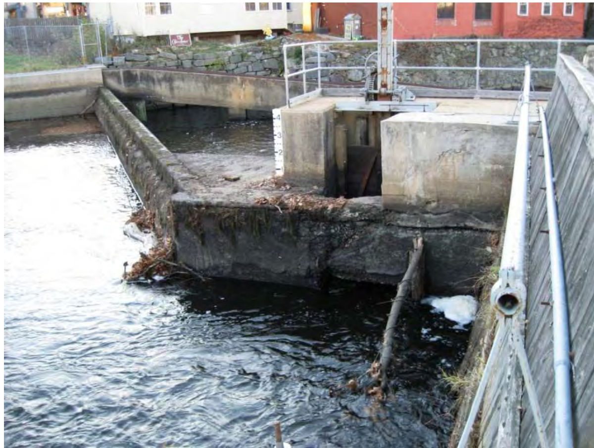
A view of the Great Dam during drawdown, November 2009
