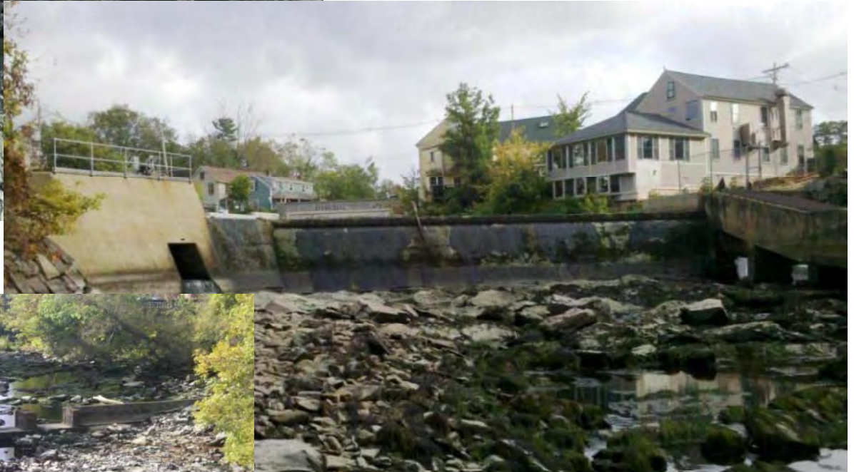
Dam & fish ladder looking upstream, Nov 2011
