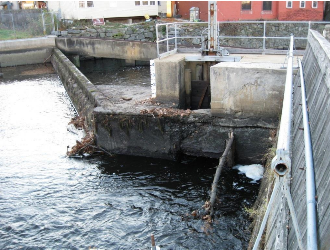
View of dam, fish passage (top center), portion of penstock baffle wall (far right), and low-level gate (center). Facing W.
