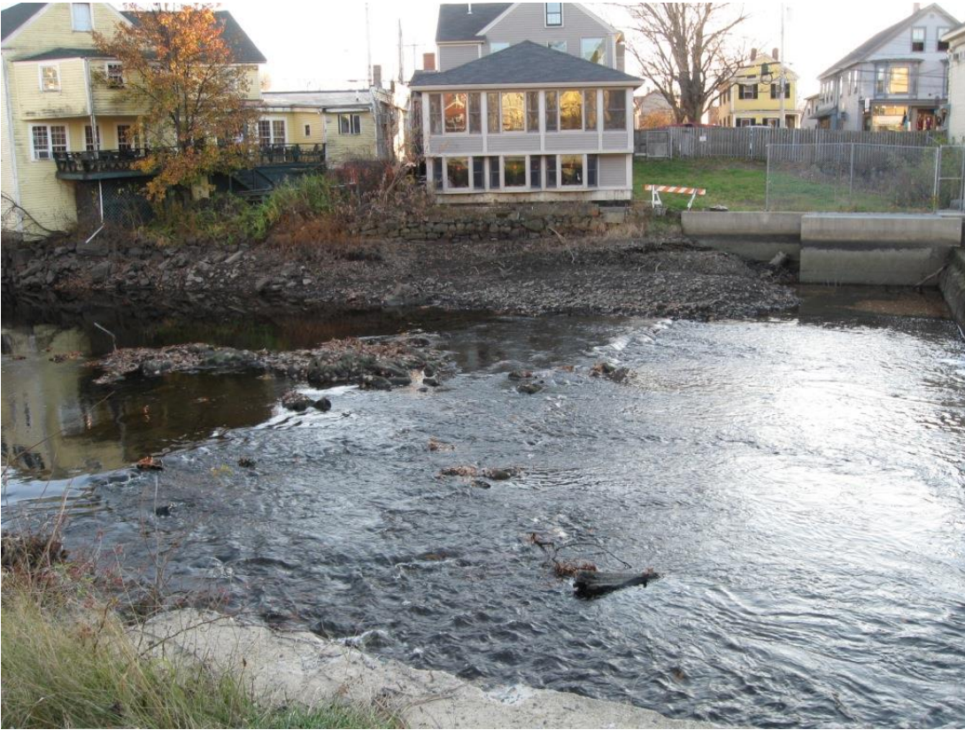
View of ledge outcrops in area just upstream of dam (dam is on far right), facing W
