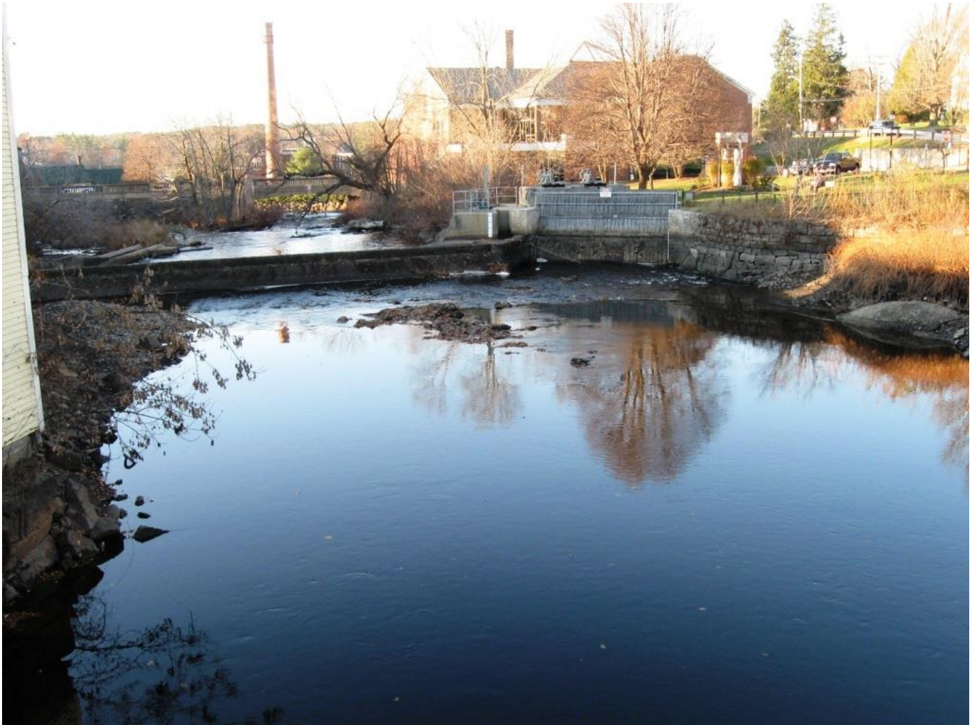
View of dam from High Street Bridge, facing N. Dam is shown in center, with penstock baffle (wood) wall and low-level gate on right hand side of photograph.
