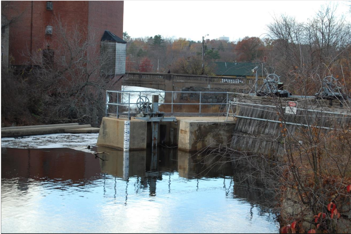
Photo # 4 Description: Low-level gate (center) and penstock baffle wall (right) Roll and Frame # OR Digital file name: EXE0043_04 Direction: NW
