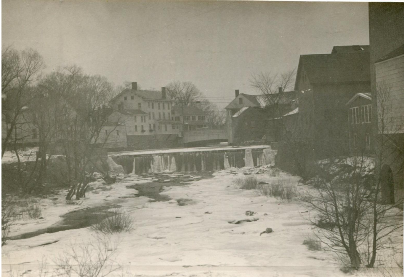
Photograph of Great Dam facing southeast, post-1915 (Ioka Theater visible on extreme right, constructed 1915). Great Bridge in background. Exeter Historical Society, MSS12_1990.35.2.
