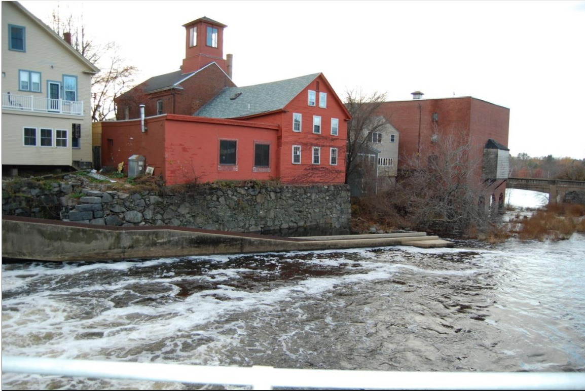
Photo # 2 Description: Ca. 1968 Fish Passage structure at west bank of Exeter River Roll and Frame # OR Digital file name: EXE0043_02 Direction: NW
