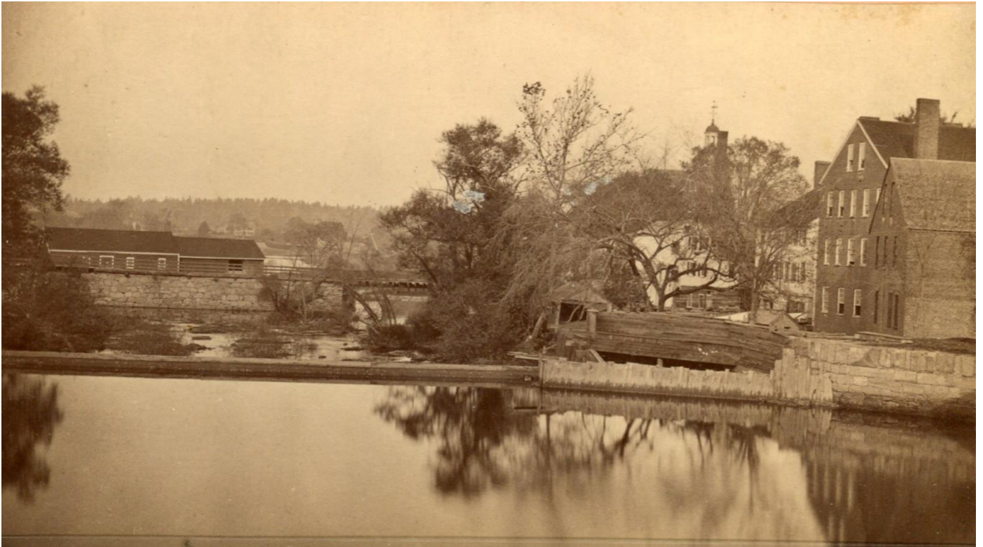
Photograph of Great Dam facing northwest, taken from Great Bridge, J.S. Mitchell photographer, no date. String Bridge and Kimball's Island in background. Exeter Historical Society, MSS12.
