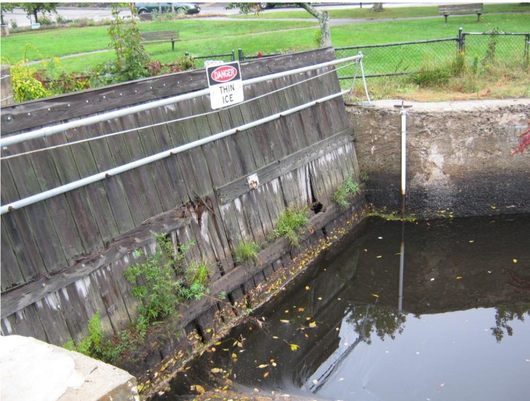
Detailed view of penstock baffle wall, facing SE
