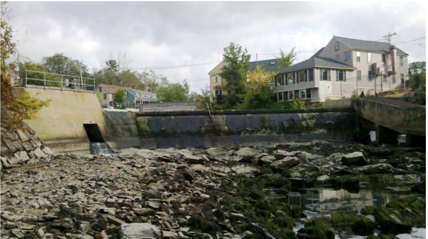
View of low-level gate (left), dam (center), and fish passage (right), facing S
