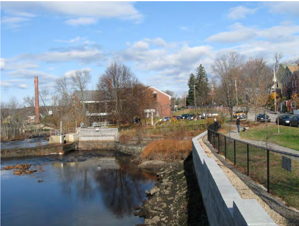
View of dam (on left), low-level gate, and penstock baffle wall, facing NE from Founders' Park
