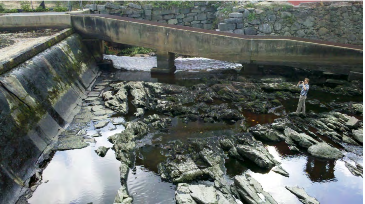
View of dam parabolic side (downstream) and fish passage, facing W
