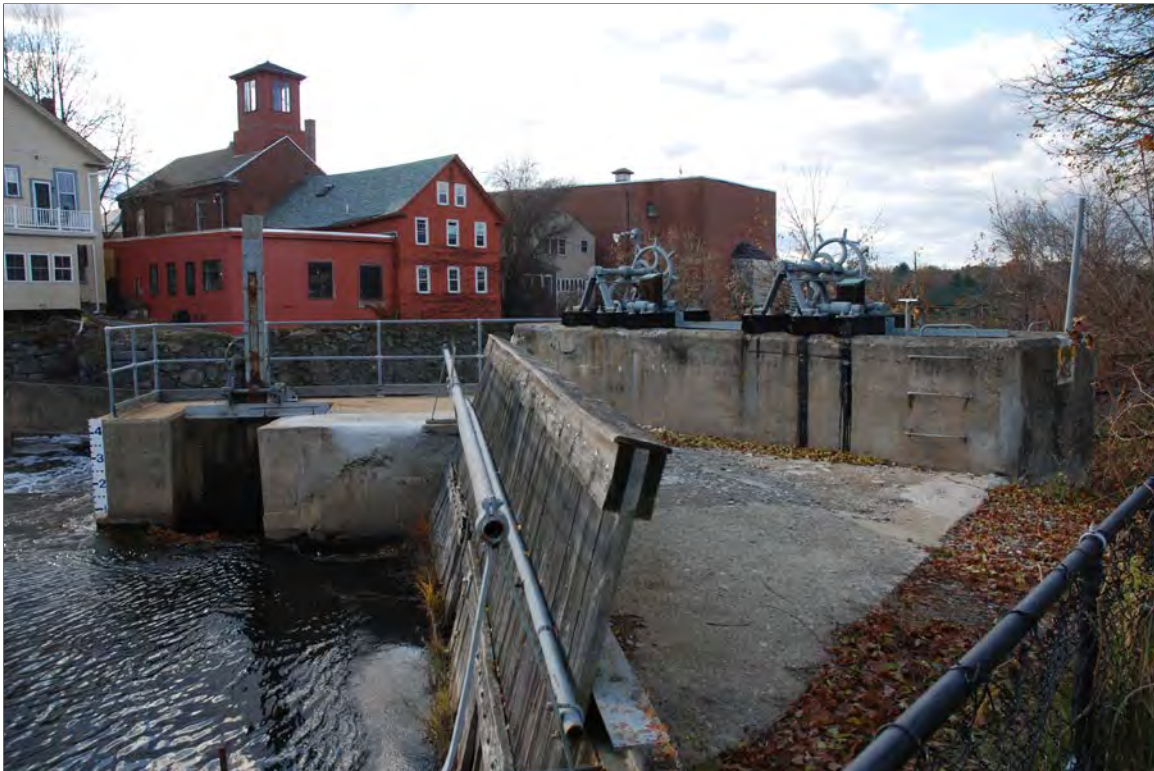
Photo # 5 Description: Low-level gate (center) and penstock baffle wall Roll and Frame # OR Digital file name: EXE0043_05 Direction: NW
