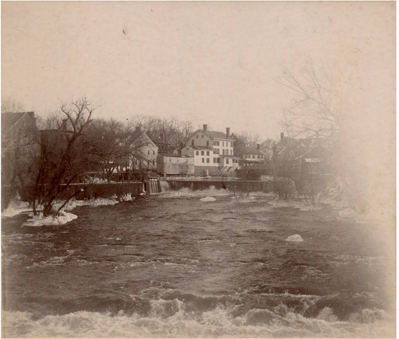
Photograph of Great Dam site facing southeast, 1896. Great Bridge in background. Exeter Historical Society, photographer Lizzie G. Rollins, presented by Dana W. Baker June 1928.
