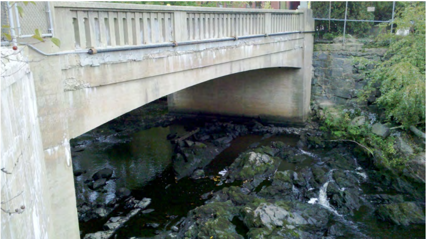
View of ledge outcrops under east of String Bridge (downstream of the dam), facing W
