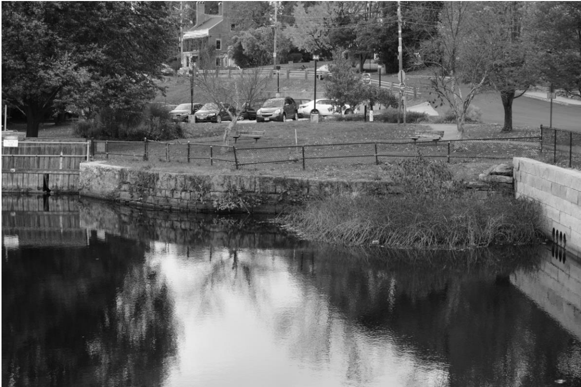
Photo 101 description: View of Wall No. 2, looking north from the Great Bridge.
