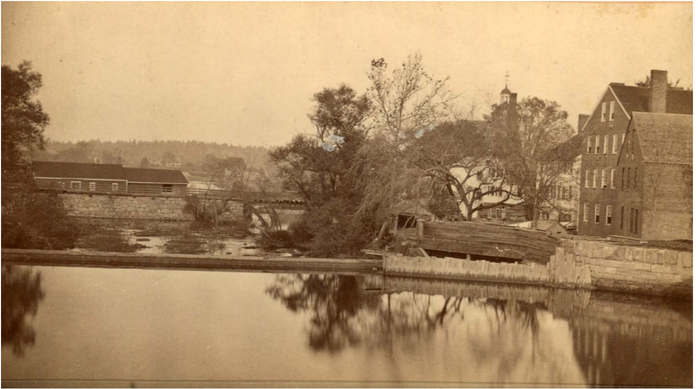
Photograph of Great Dam facing northwest, taken from Great Bridge, J.S. Mitchell photographer, no date. String Bridge and Kimball's Island in background. Exeter Historical Society, MSS12.
