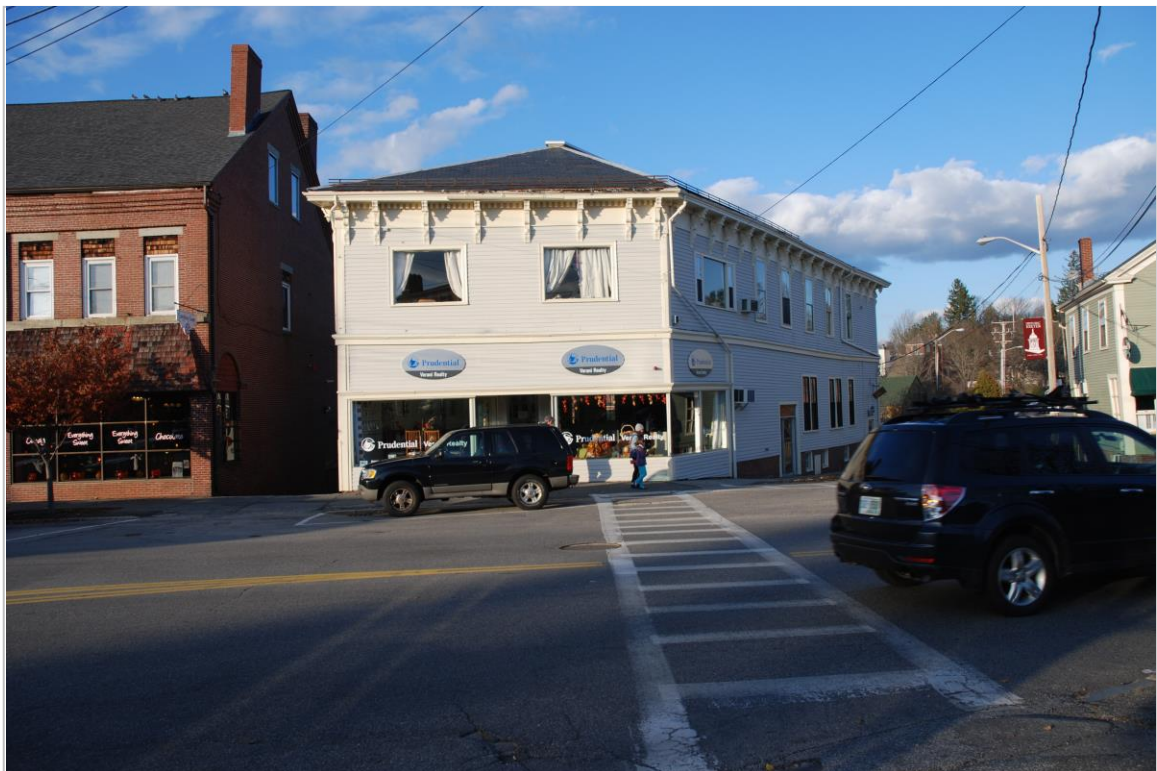
Photo 10 description: Water Street at String Bridge, east side
