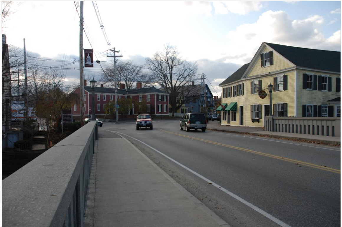
Photo 49 description: High Street Bridge, facing towards intersection with Water Street on right and Franklin Street on left
