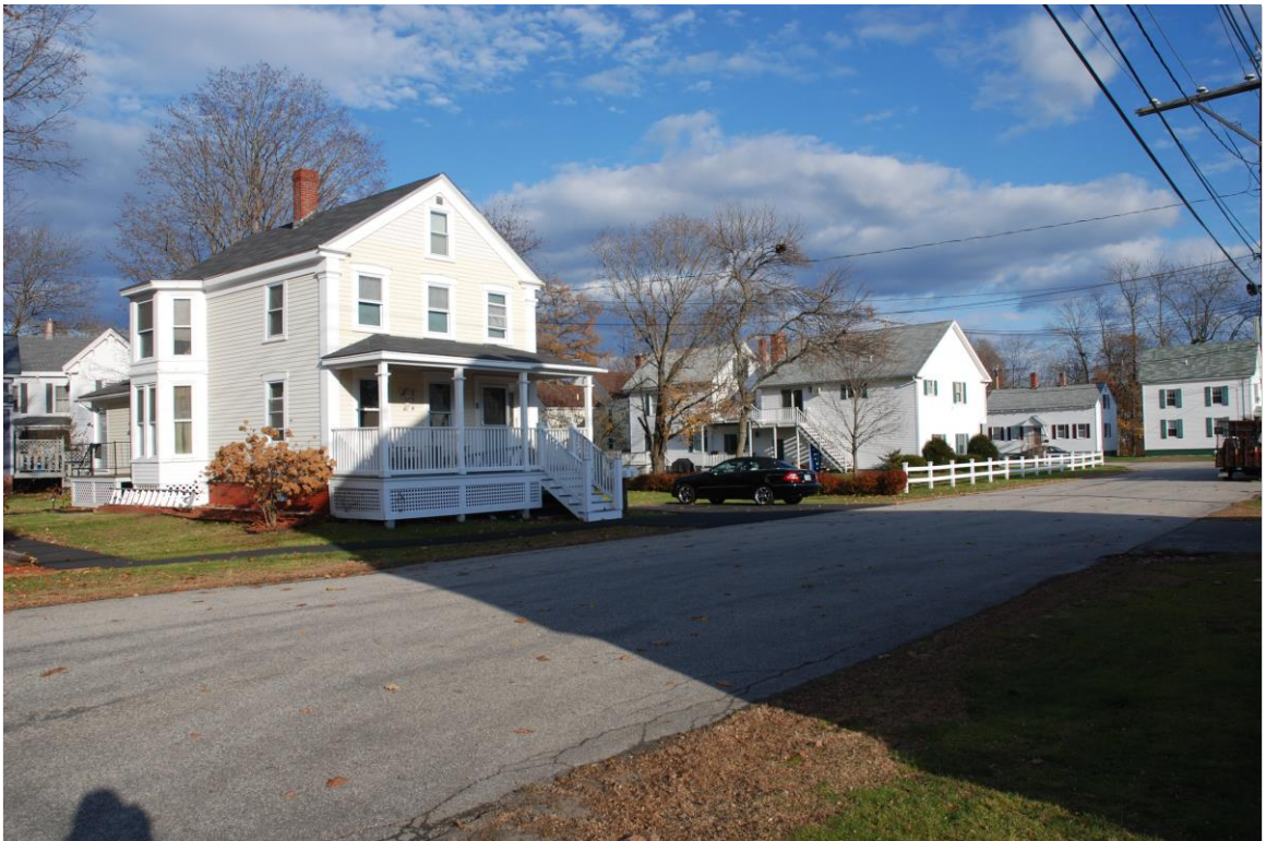
Photo 98 description: Outside of project area, 8 River Street Extension
