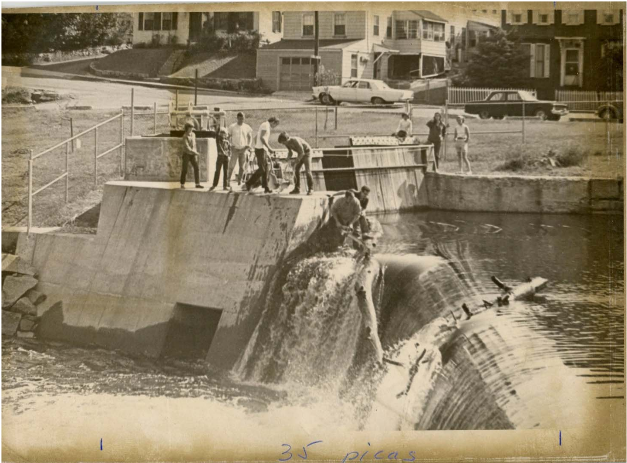
Photograph of Great Dam facing east, 1972, Pleasant Street in background. Exeter Historical Society, MSS12_1998.91.99.
