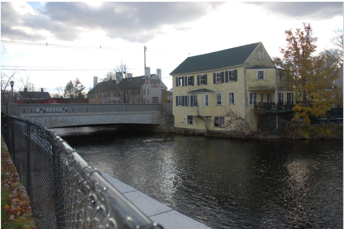
Photo 22 description: High Street Bridge and Loaf and Ladle building, 1-9 Water Street+ from Founders Park
