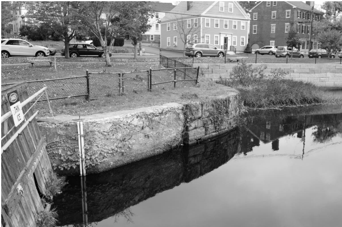
Photo 102 description: Wall No. 2 (granite), at junction with concrete penstock abutment.
