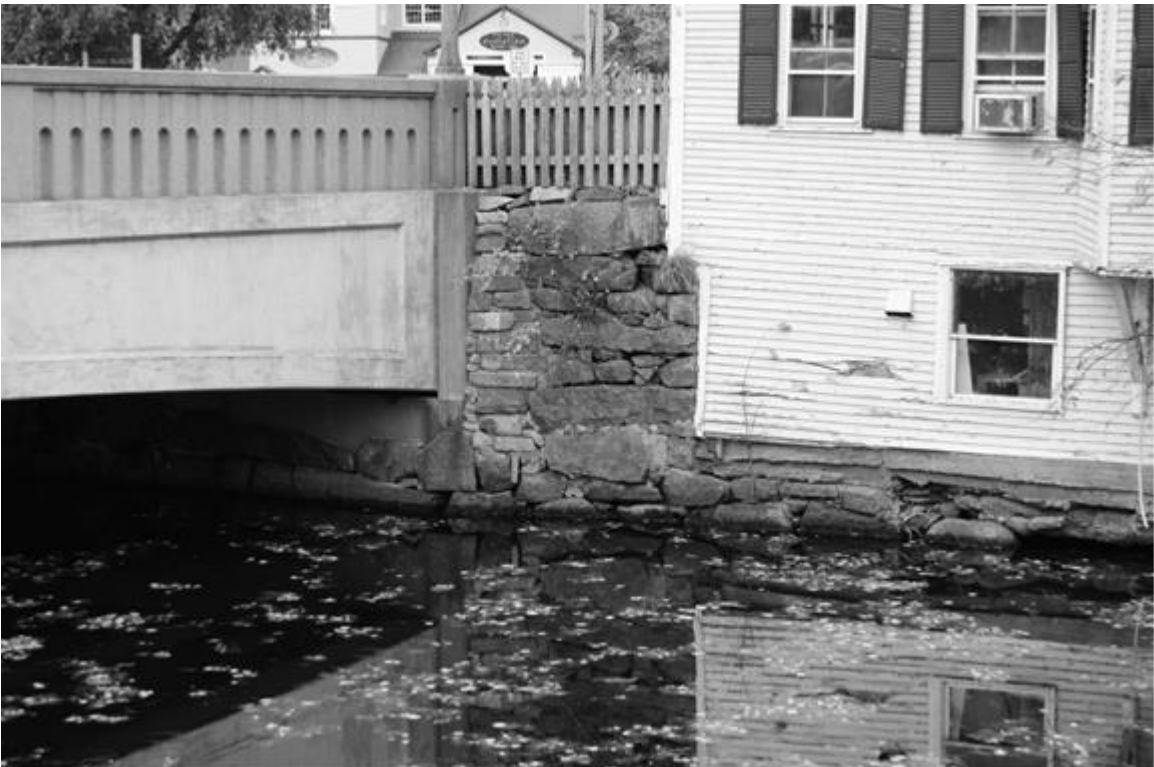
Photo 116 description: View of foundation wall at 1-9 Water Street (Wall No. 10).
