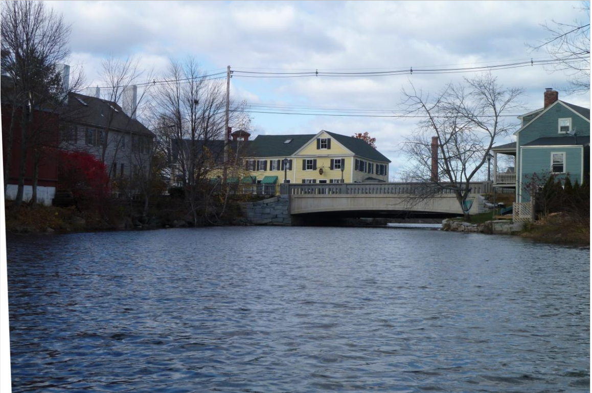
Photo 75 description: View of High Street Bridge, facing north from Exeter River
