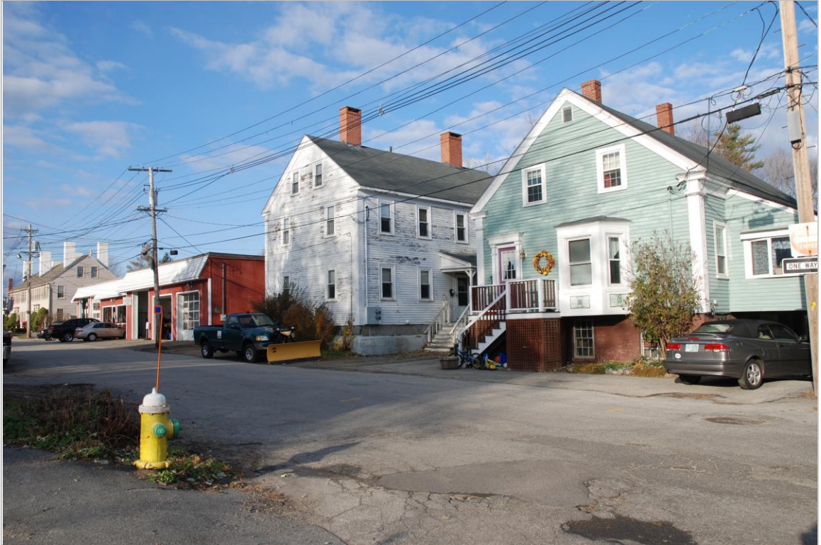
Photo 55 description: 26 and 30 Franklin Street
