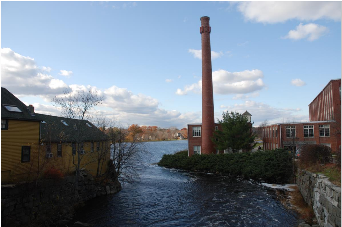
Photo 28 description: East side of Exeter River, north of String Bridge, Exeter Mfg. Co. complex on right
