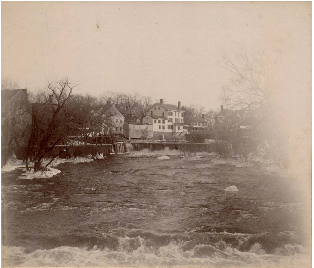
Photograph of earlier dam on site of Great Dam facing southeast, 1896. Great Bridge in background. Exeter Historical Society, photographer Lizzie G. Rollins, presented by Dana W. Baker June 1928.
