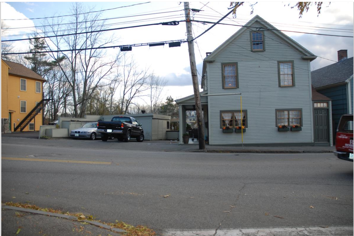
Photo 46 description: 11 High Street, facing west
