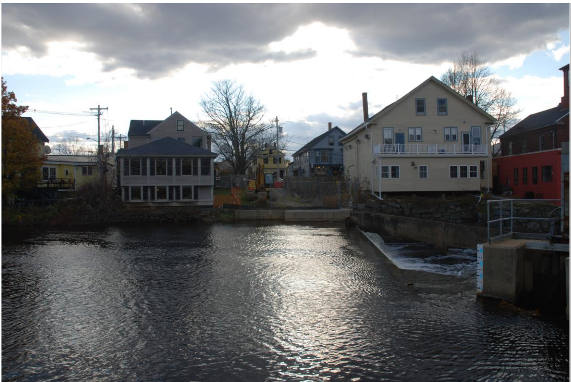
Photo 20 description: Rear of Water Street buildings and Great Dam and portion of fish ladder, from Founders Park
