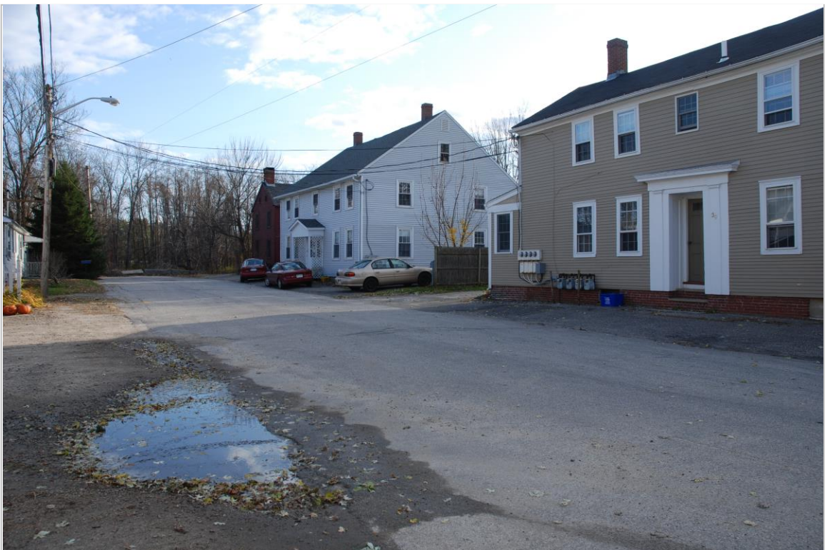
Photo 62 description: 47, 43-45 and portion of 2 South Street (left to right)
