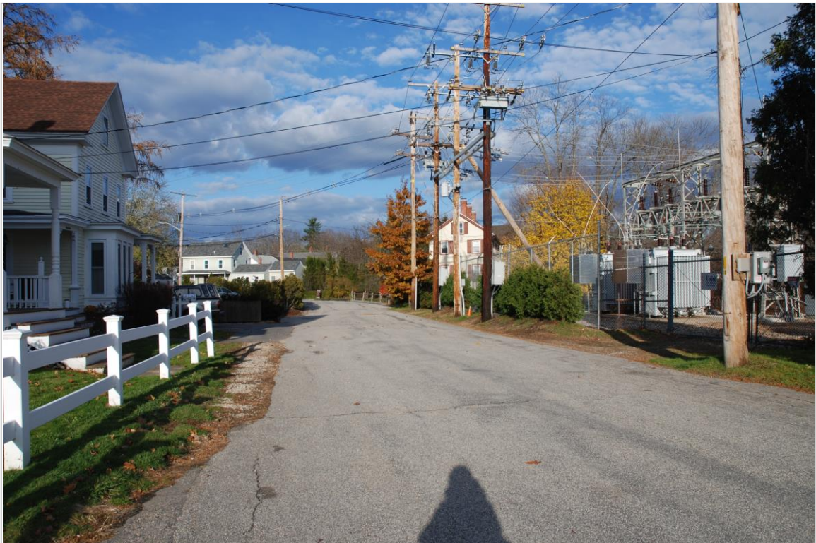
Photo 66 description: River Street, facing northeast from in front of 19 River Street
