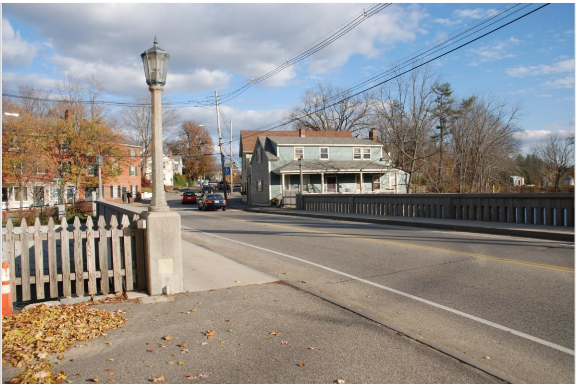
Photo 44 description: High Street Bridge, from intersection with Water and Franklin Streets
