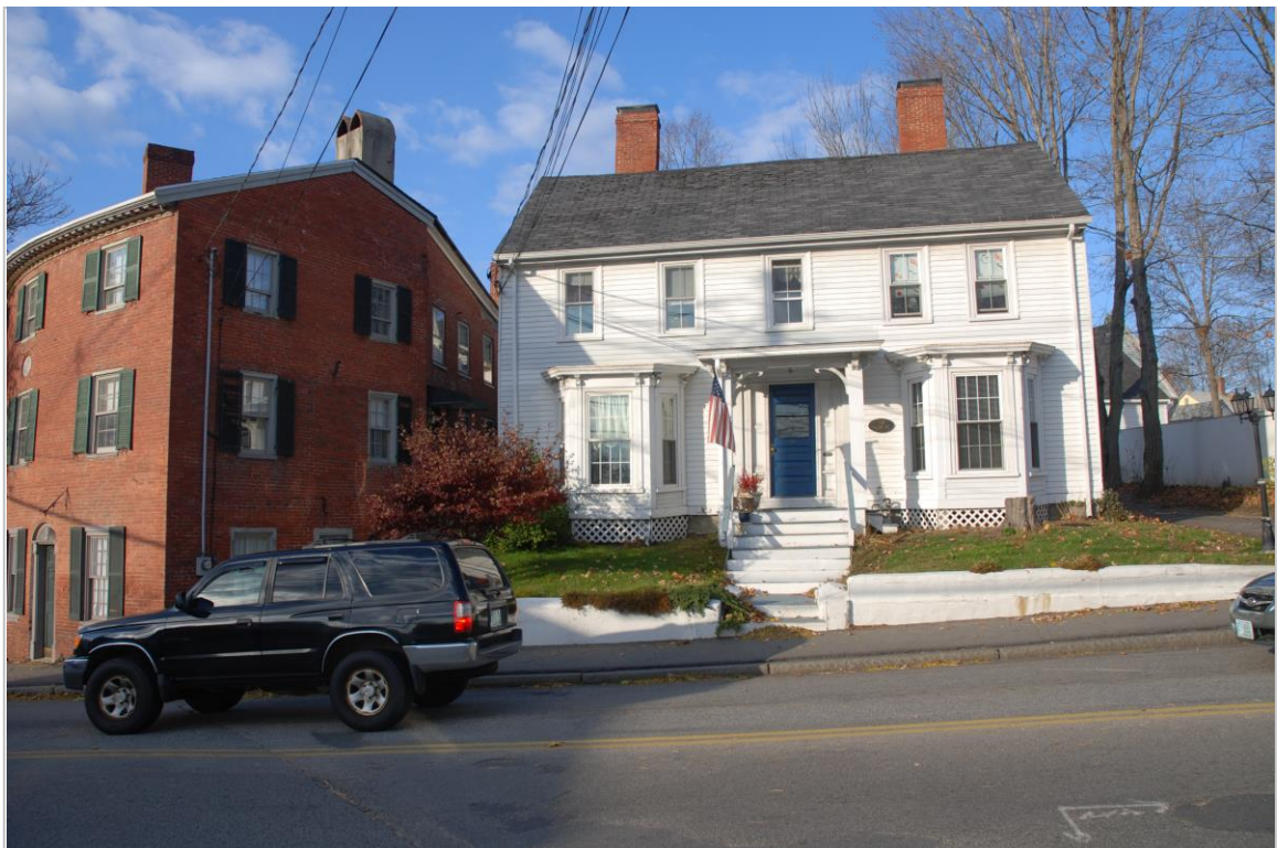
Photo 42 description: 8 and 10 High Street, facing north
