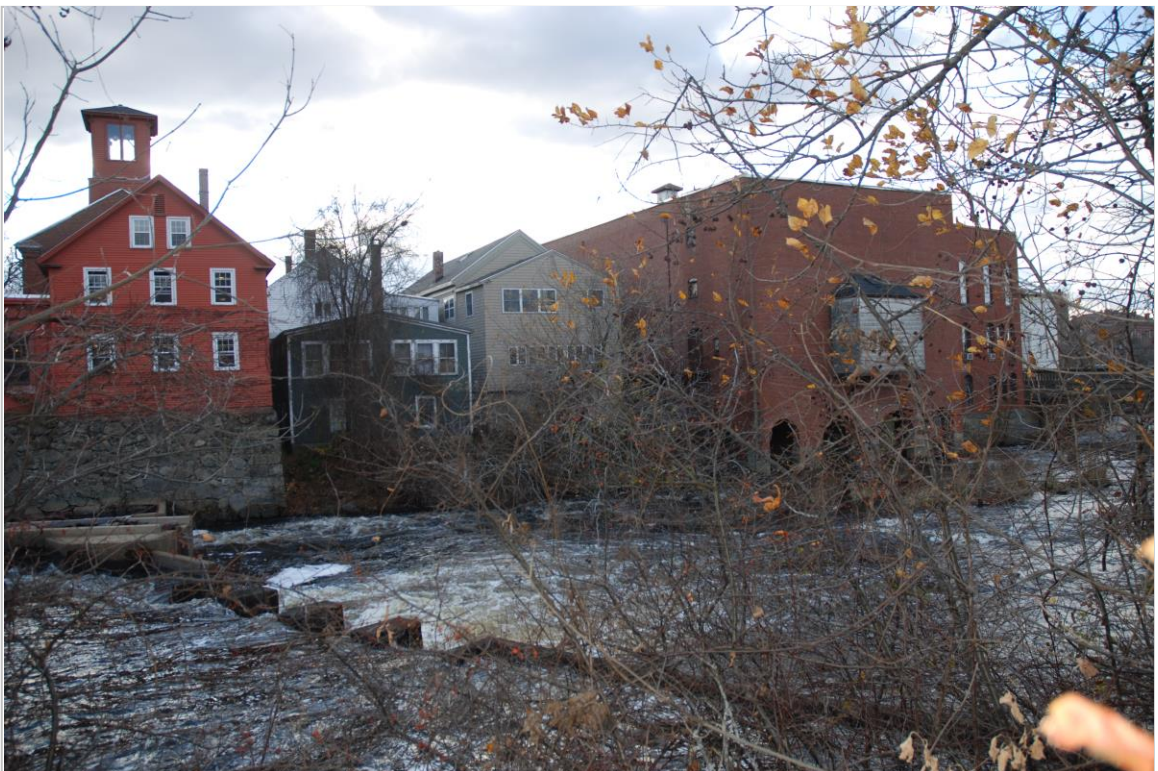
Photo 16 description: Fish ladder (on extreme left) and concrete weir, rear of Water Street buildings, from Founders Park
