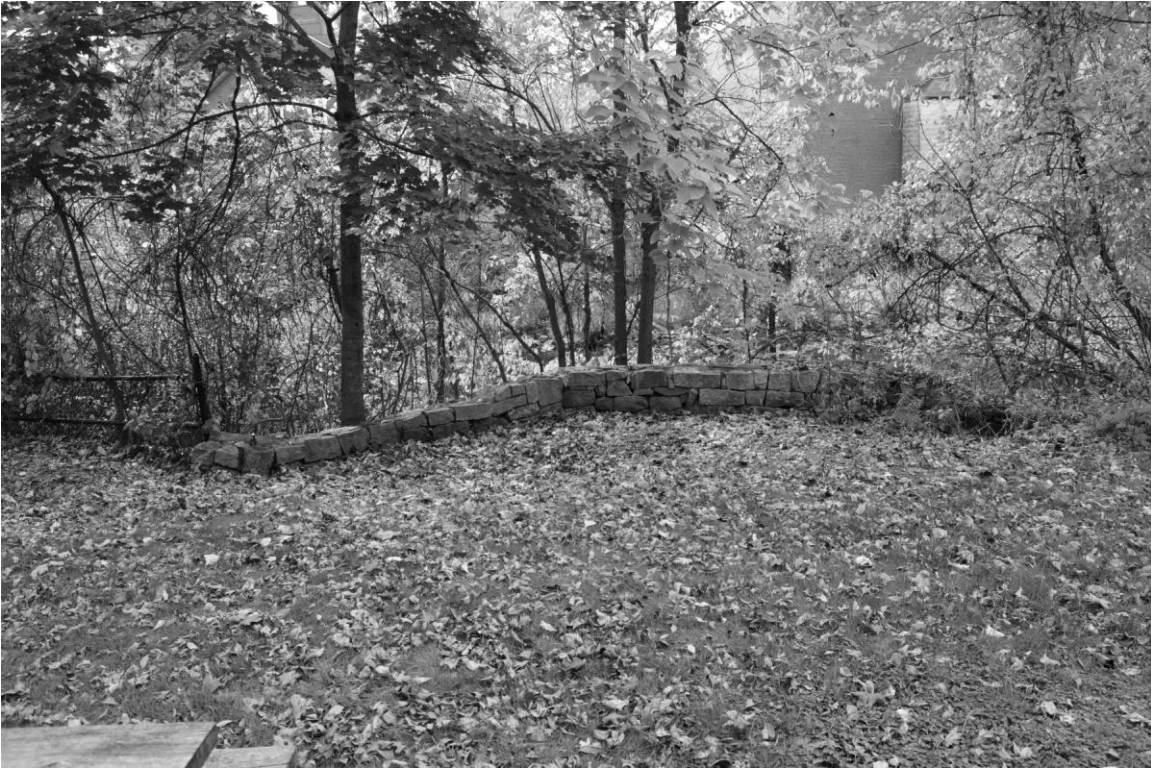
Photo 105 description: Wall No. 5, showing uphill face.
