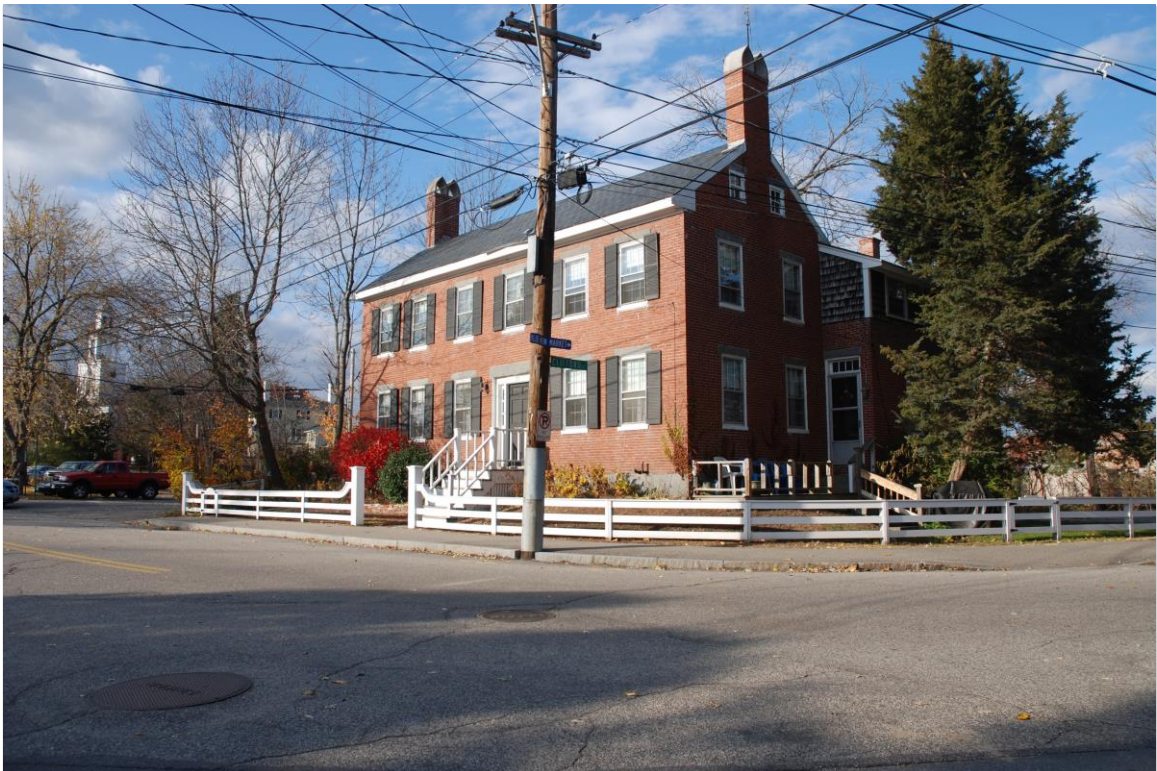
Photo 92 description: Outside of project area, 10 Bow Street, from intersection of Bow and Clifford Streets
