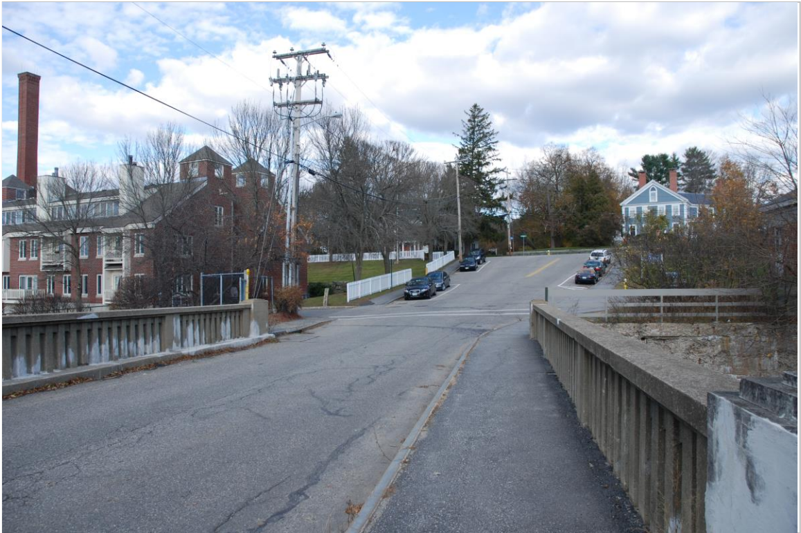
Photo 31 description: String Bridge towards Chestnut Street (new housing in former Exeter Mfg. Co. complex on left Roll: Frame: Direction: E Date taken: 11-2011 Negative stored:
