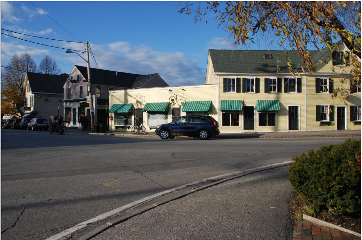
Photo 12 description: Loaf and Ladle Building, northeast corner Water Street and High Street, 1-9 High Street
