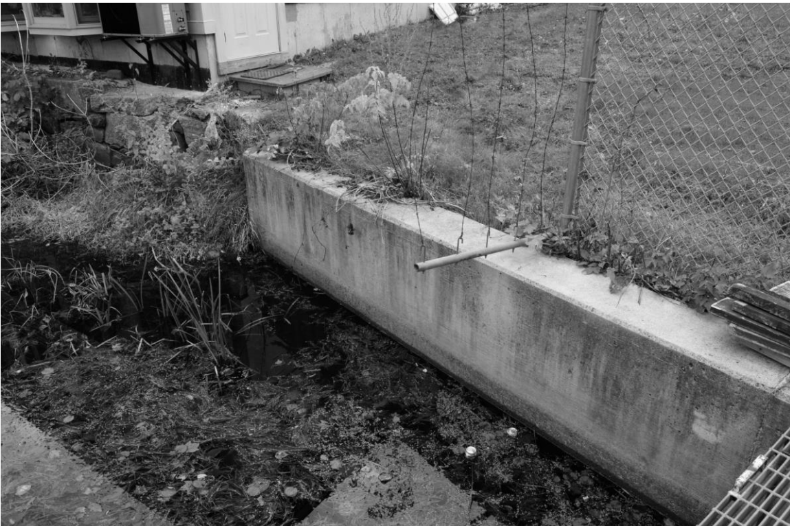
Photo 112 description: Concrete retaining wall at 23 Water Street (Wall No. 8).
