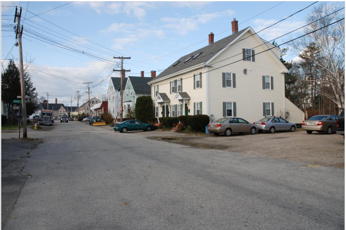
Photo 56 description: East side of Franklin Street, 32-36 Franklin Street on right, foreground
