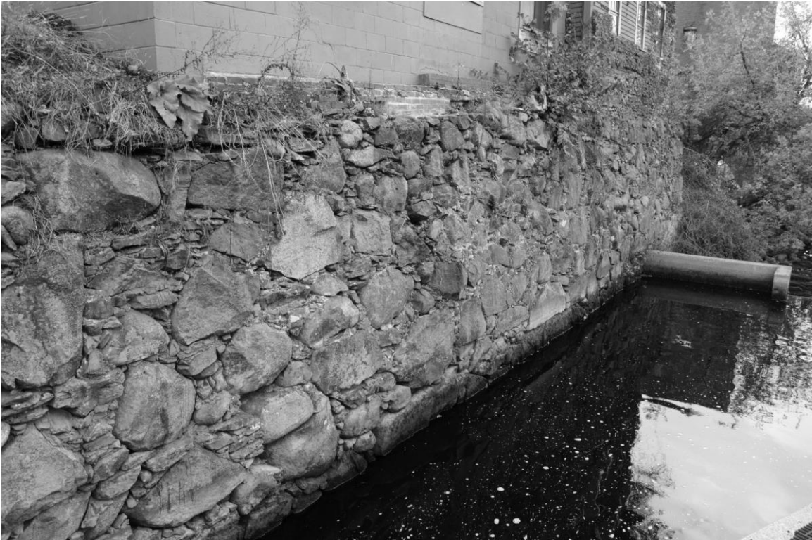
Photo 109 description: Detail of Wall No. 6, showing connection to lower dam (fish weir). Roll: _____ Frame: _____ Direction: W Date taken: 10/2014 Negative stored: _____
