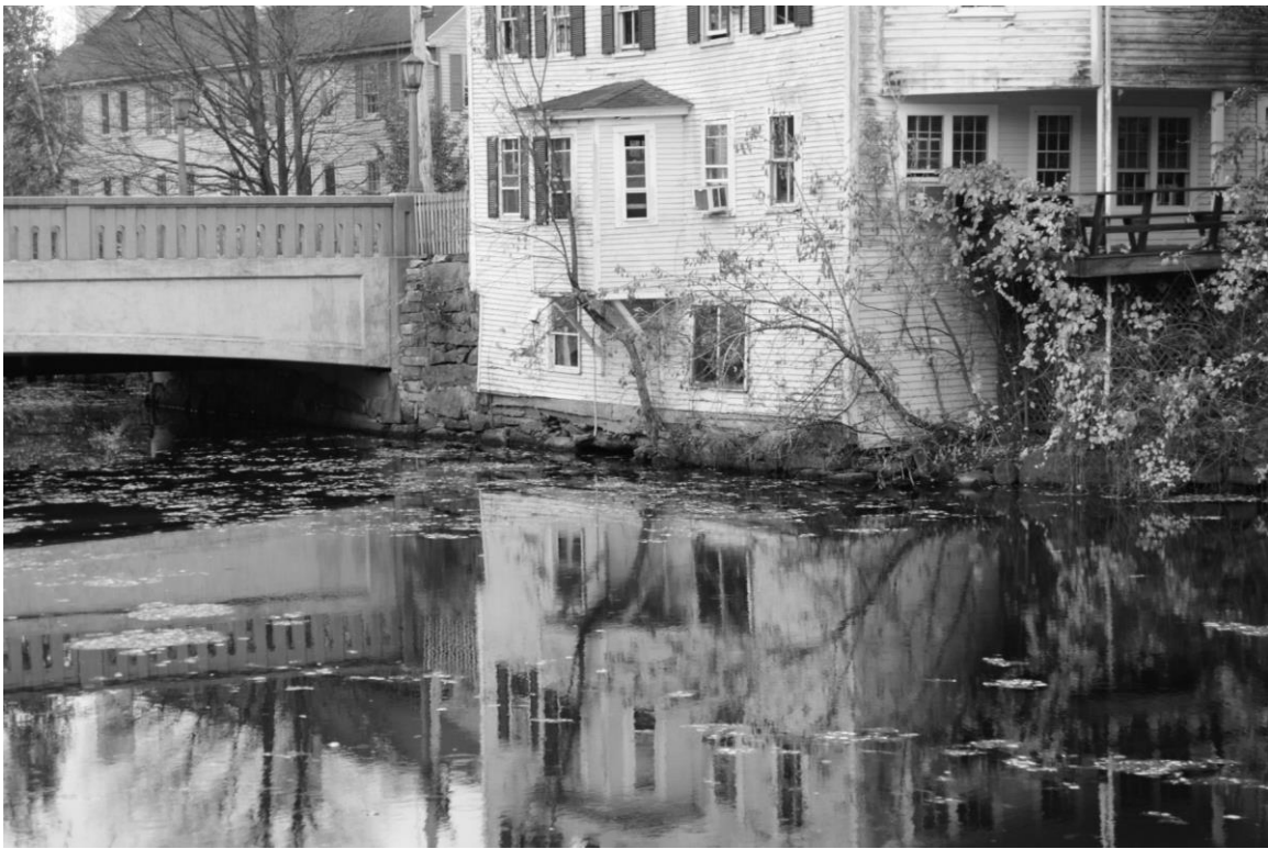
Photo 115 description: View of foundation wall at 1-9 Water Street (Wall No. 10).
