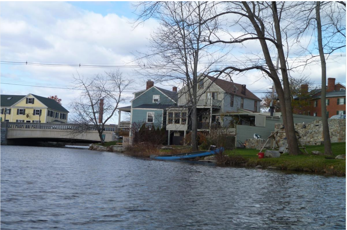
Photo 76 description: View north, east of High Street Bridge, 5 and 11 High Street in center from Exeter River
