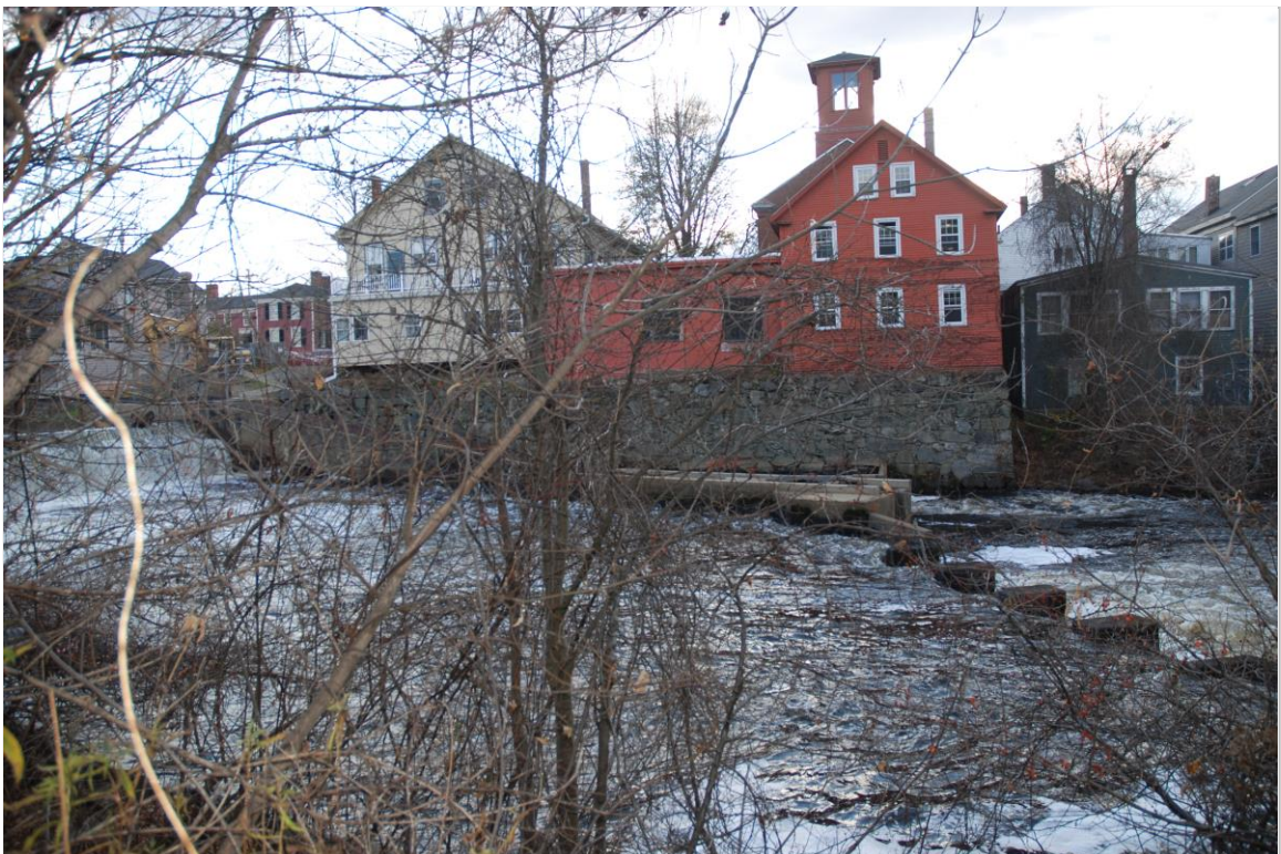
Photo 18 description: Great Dam, fish ladder, and concrete weir, rear of Water Street buildings, from Founders Park
