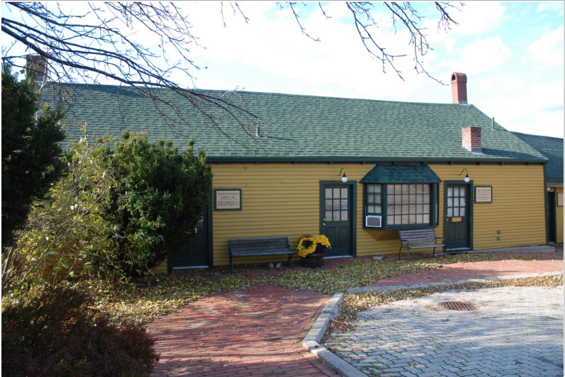
Photo 23 description: West building on Kimball's Island
