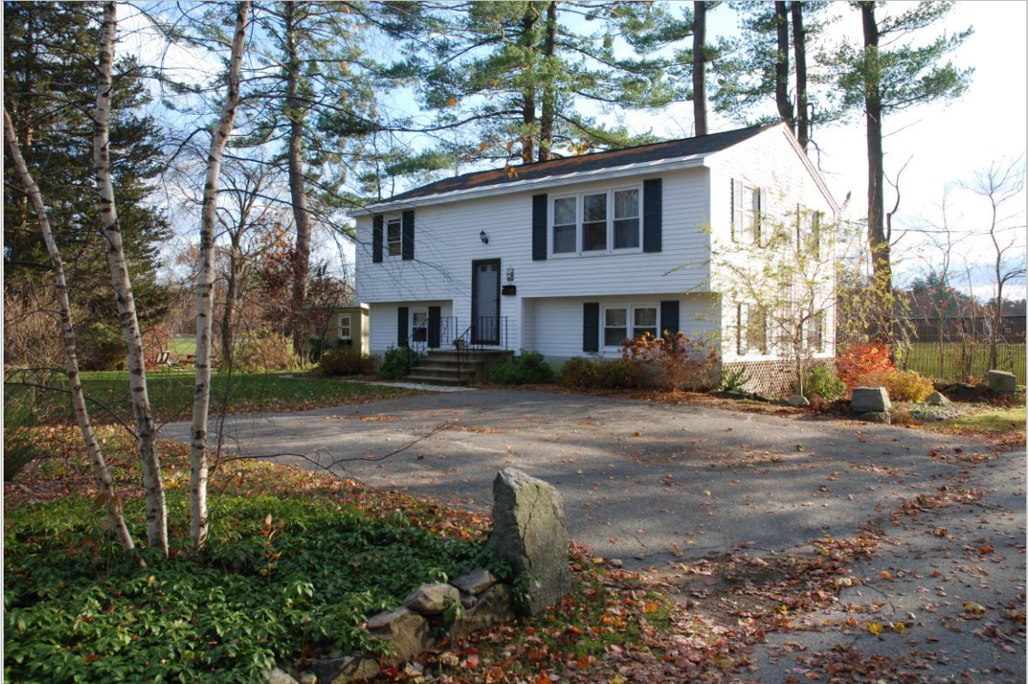
Photo 71 description: 44 River Street, facing southeast
