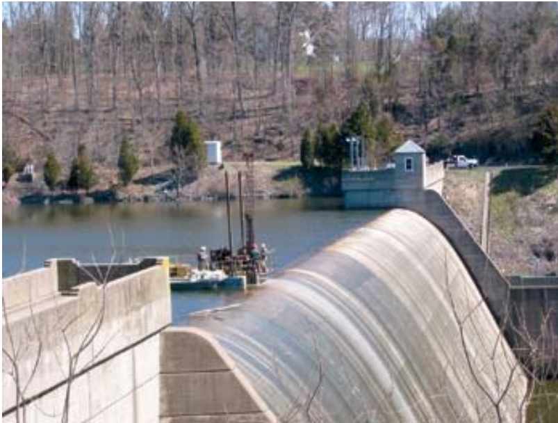
Drilling the Dam
