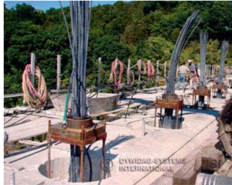
Installing the Anchors
