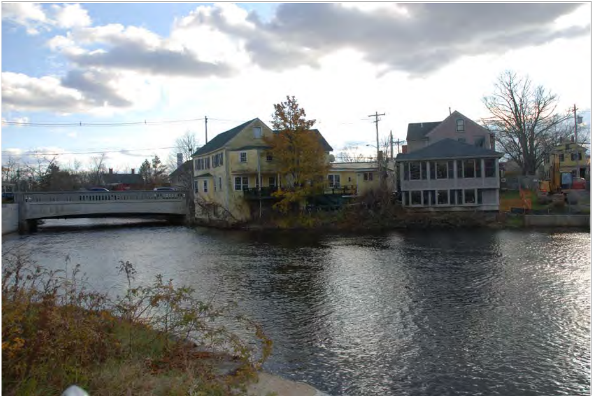
Photo 21 description: High Street Bridge, Loaf and Ladle Building, 1-9 Water Street and 11 Water Street on right
