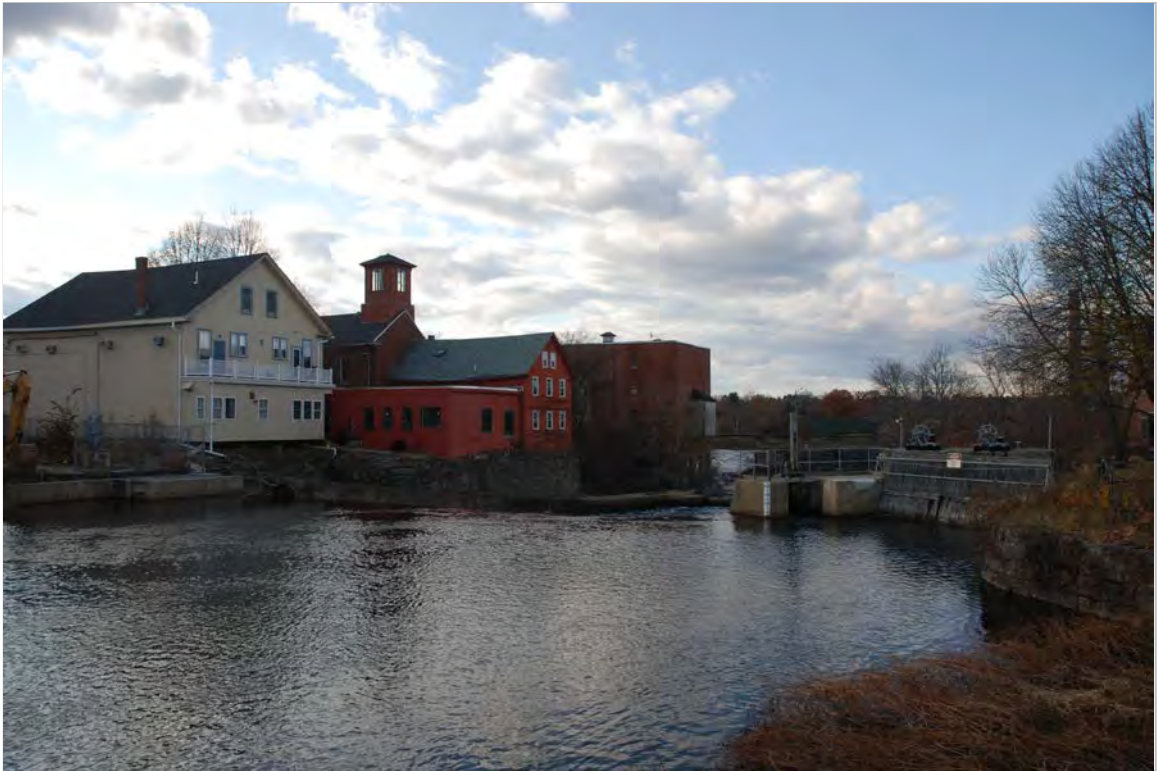
Photo 17 description: Rear of Water Street buildings, facing west from Pleasant Street
