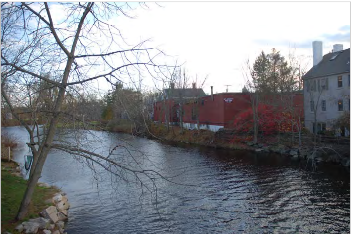
Photo 52 description: East, rear sides of buildings on east side of Franklin Street, south of High Street
