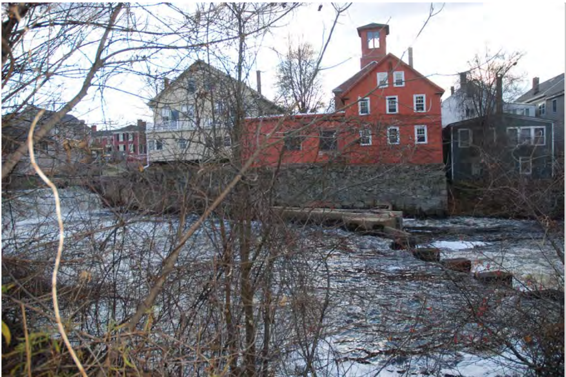
Photo 18 description: Great Dam, fish ladder, and concrete weir, rear of Water Street buildings, from Founders Park
