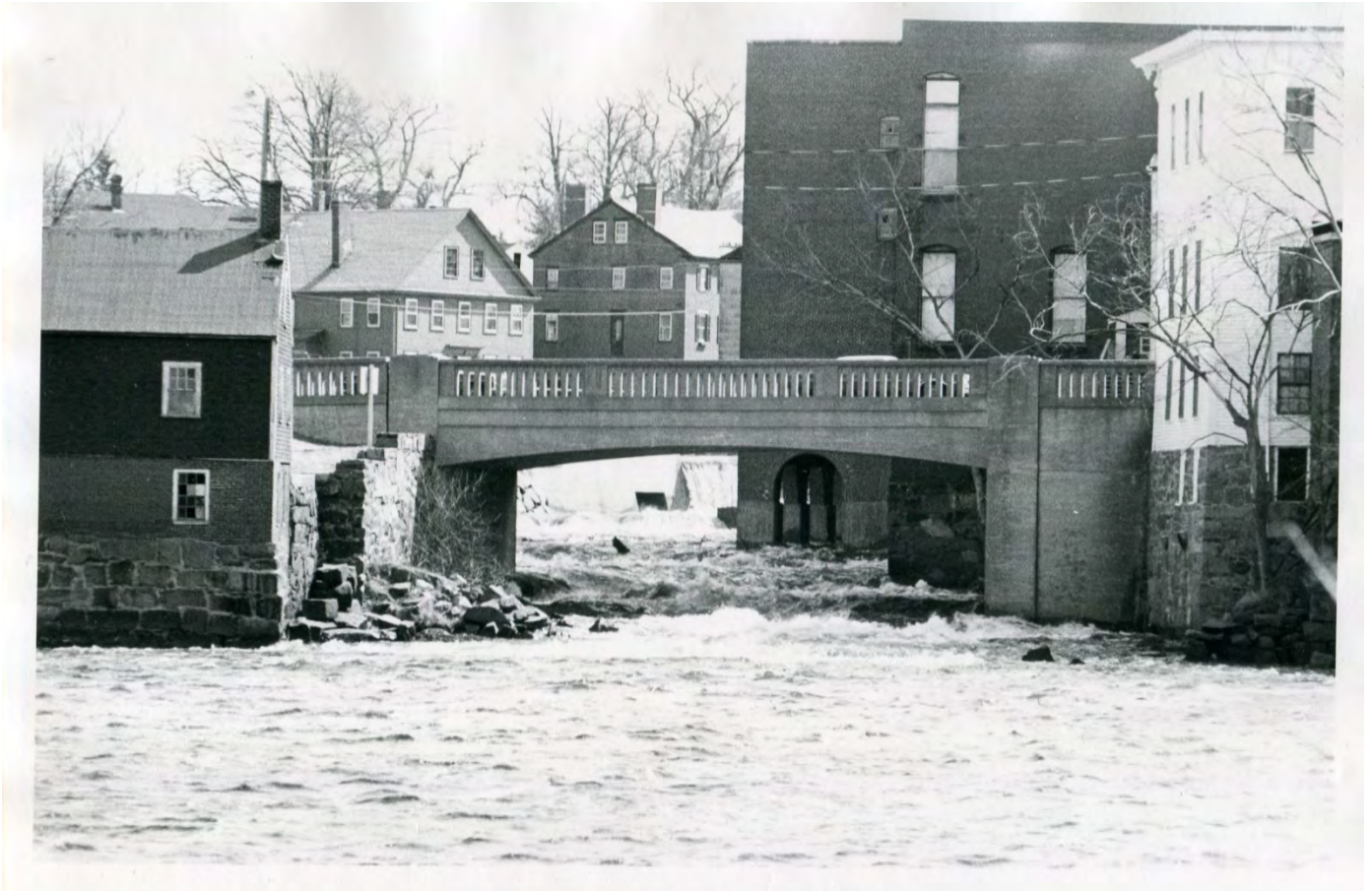
Photograph of String Bridge and Kimball's Island facing southeast, Great Dam visible in background through bridge, post-1935 (concrete bridge constructed 1935). Exeter Historical Society, MSS12_1998.89.24.
