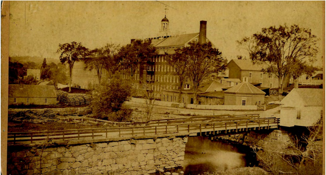
Photograph of String Bridge facing north, Exeter Manufacturing Company mill in background. J.S. Mitchell, identified by Aten (2003) as 1882-1884. Exeter Historical Society, MSS91.
