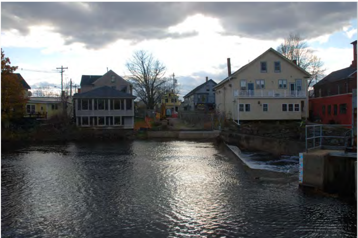
Photo 20 description: Rear of Water Street buildings and Great Dam and portion of fish ladder, from Founders Park
