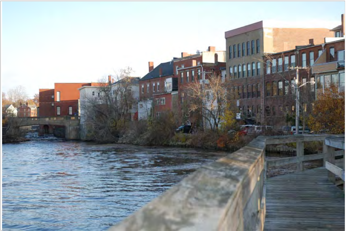
Photo 5 description: East side of Water Street buildings, north of String Bridge
