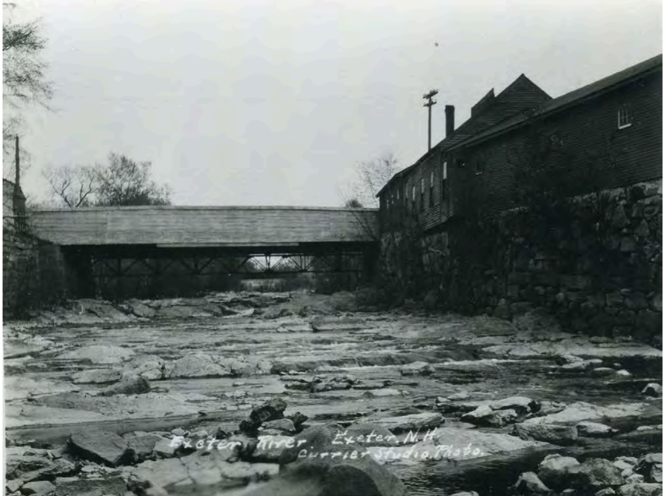
Photograph of Great Bridge facing south, pre-1935 (concrete bridge constructed 1935). Exeter Historical Society, MSS12_1995.45.3.
