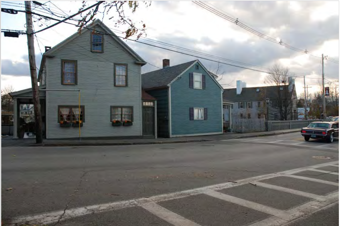
Photo 45 description: 11 and 5 High Street, west of High Street Bridge
