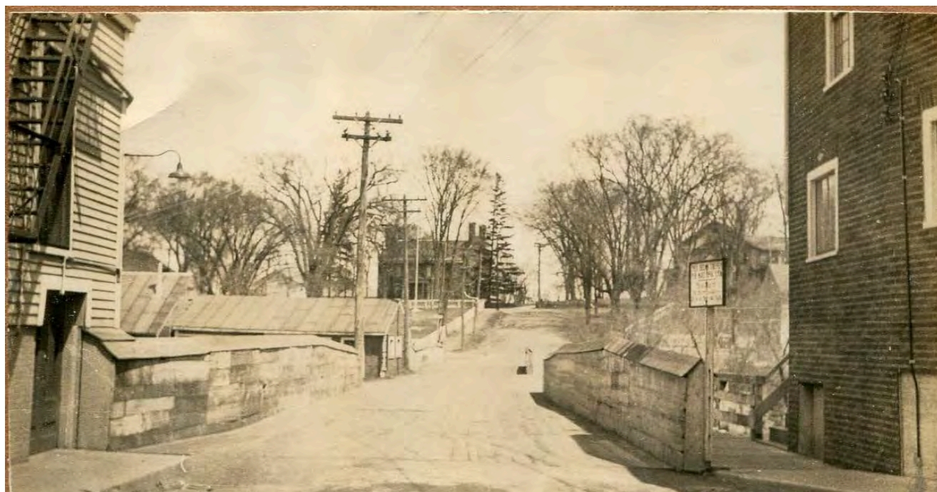
Photograph of String Bridge facing east, pre-1935 (concrete bridge constructed 1935). Exeter Historical Society, MSS91_89.21.77.
