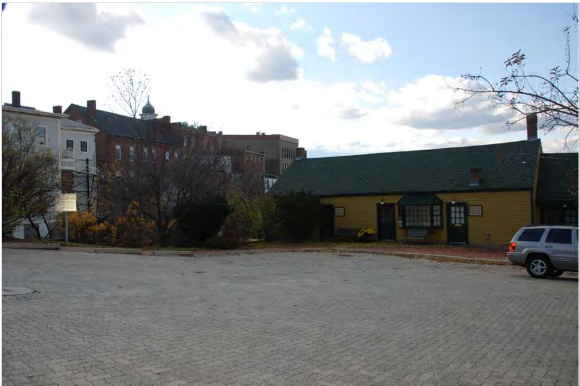
Photo 24 description: West building on Kimball Island's and rear of Water Street buildings from String Bridge
