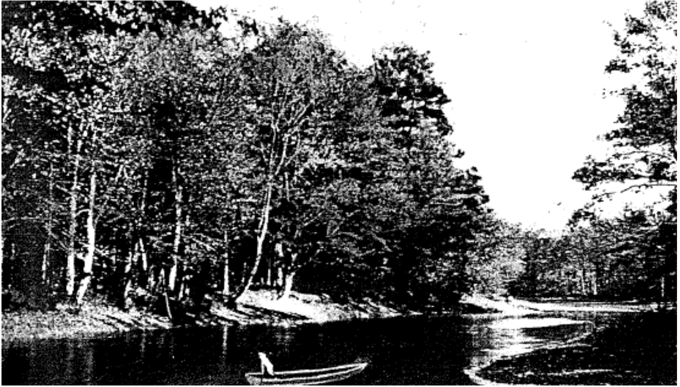
Photograph of Exeter River at Gilman Park, 1910. Aten, 2003.
