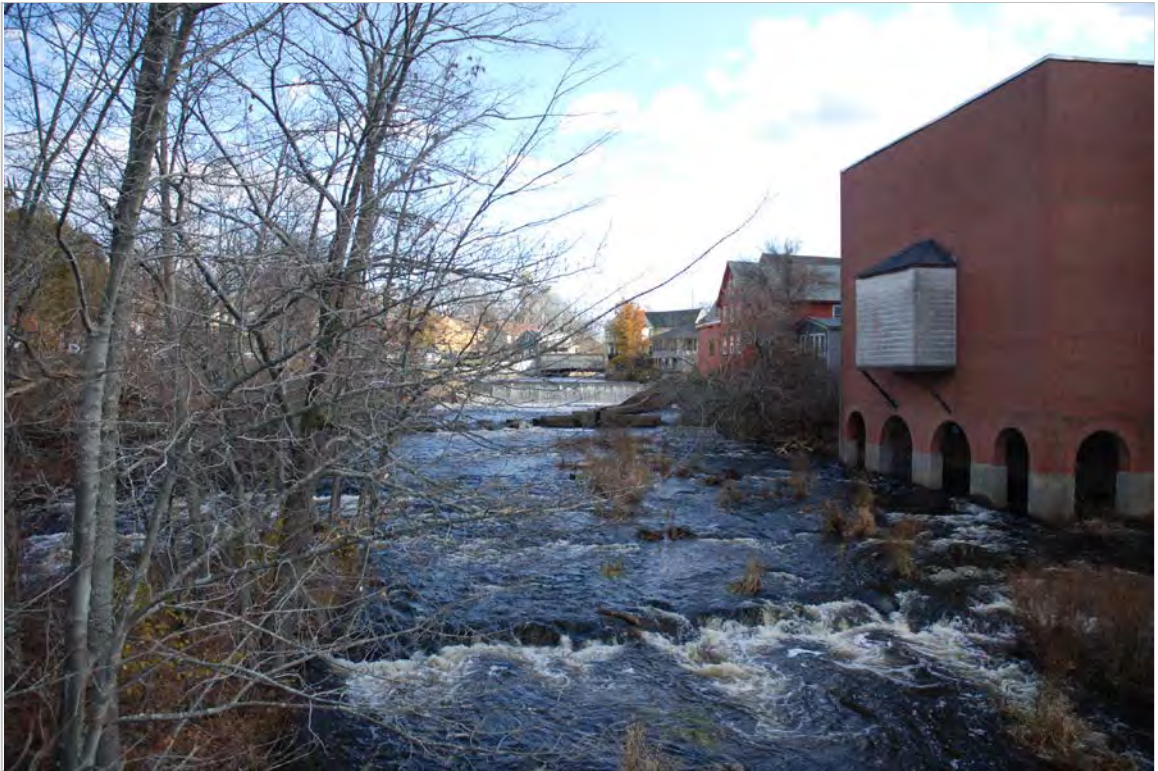
Photo 15 description: Exeter Great Dam and falls, facing north from String Bridge Roll: Frame: Direction: N Date taken: 11-2011 Negative stored:
