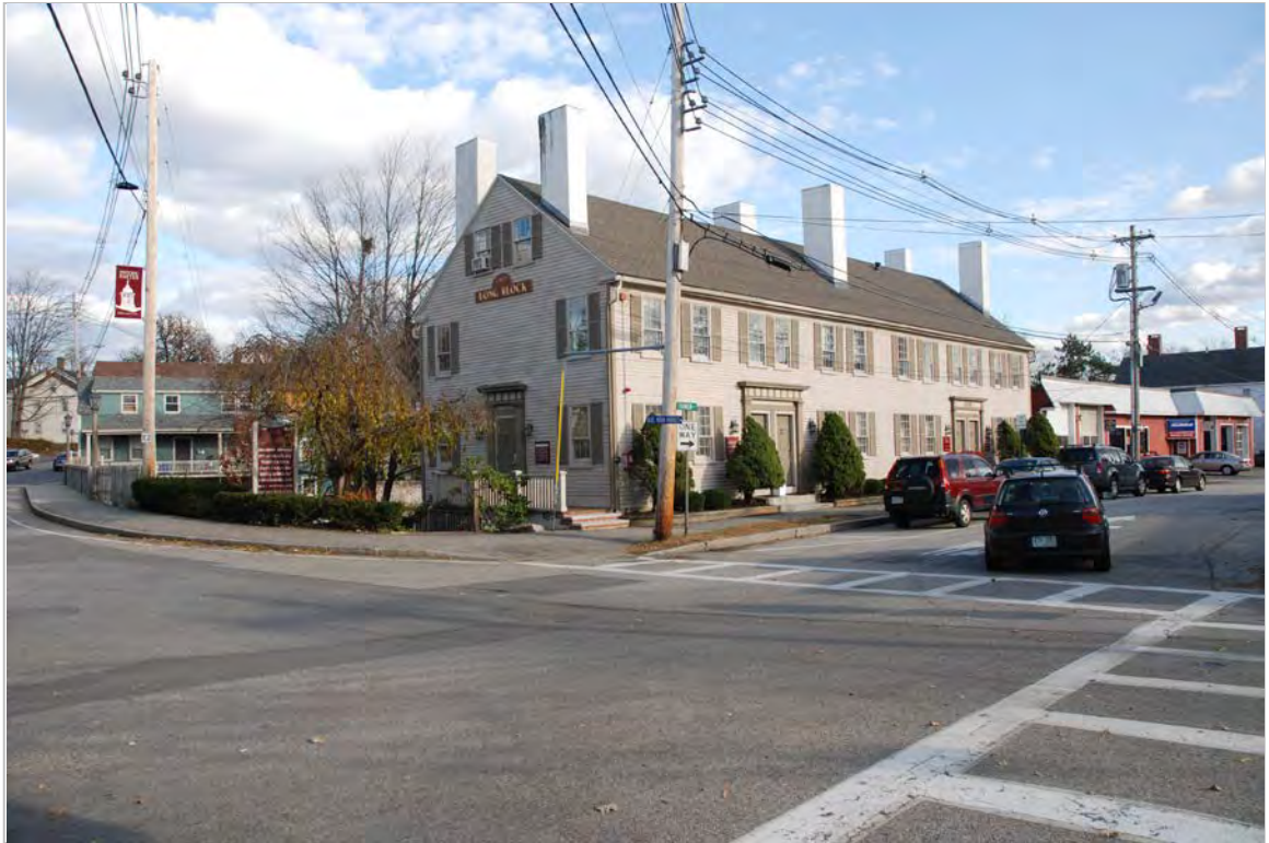
Photo 53 description: Franklin, High and Clifford Street intersection, 4-10 Franklin Street in foreground
