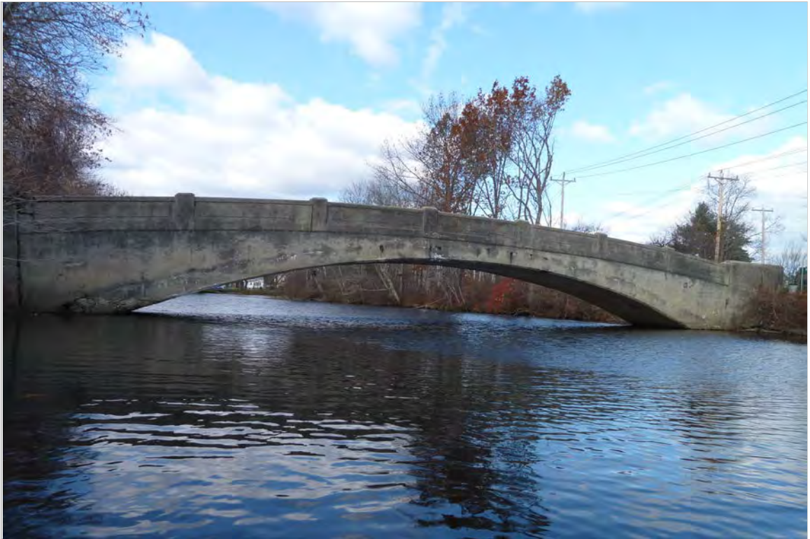
Photo 85 description: View of Phillips Exeter Academy footbridge, facing north from Exeter River
