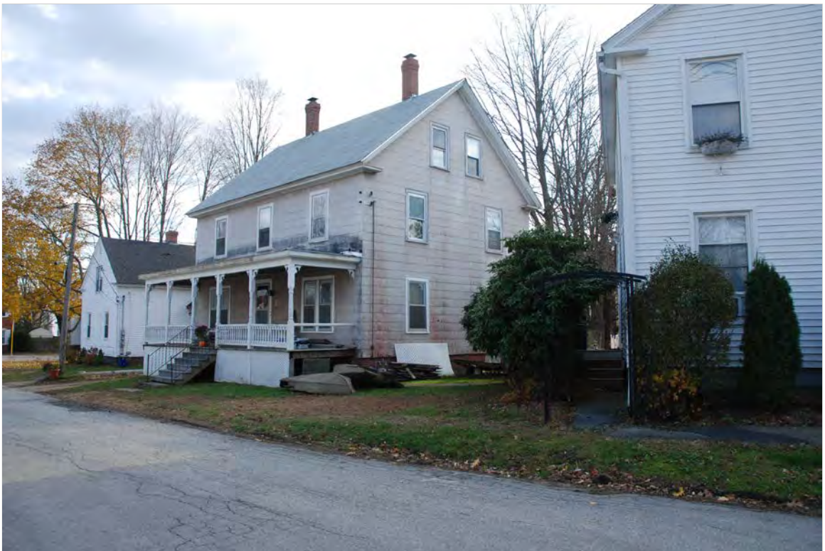
Photo 94 description: Outside of project area, 19 and 21 Bow Street
