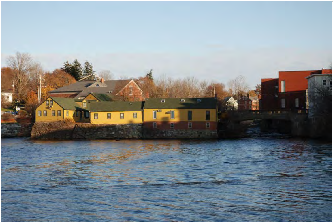
Photo 4 description: North side of Kimball Island buildings, facing south
