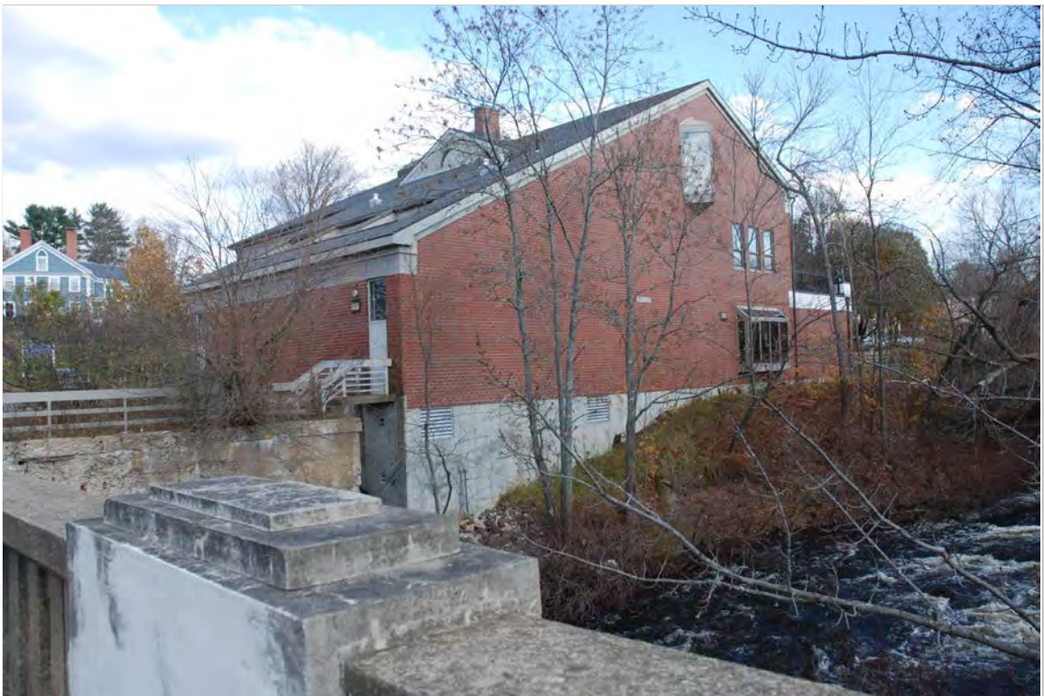
Photo 32 description: Exeter Public Library, 4 Chestnut Street, from String Bridge Roll: Frame: Direction: E Date taken: 11-2011 Negative stored:
