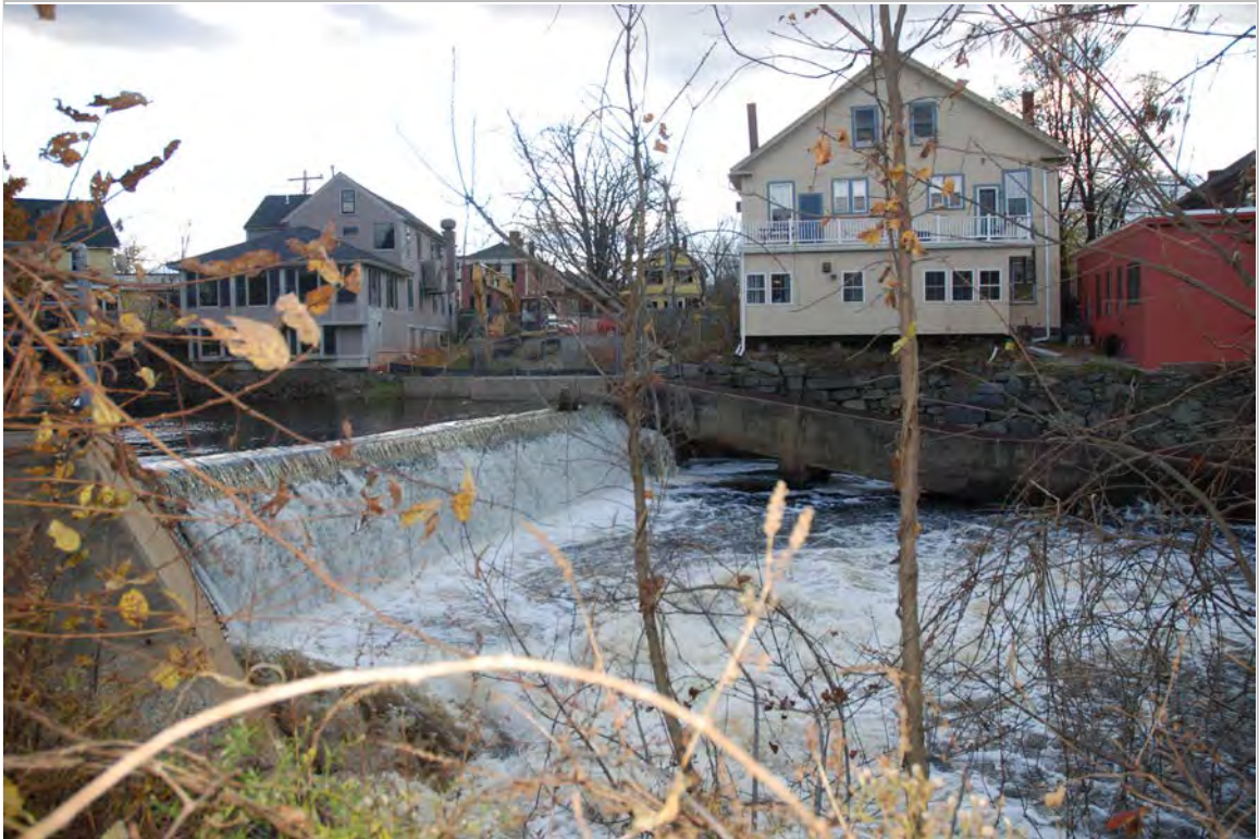
Photo 19 description: Great Dam and fish ladder, rear of Water Street buildings, from Founders Park
