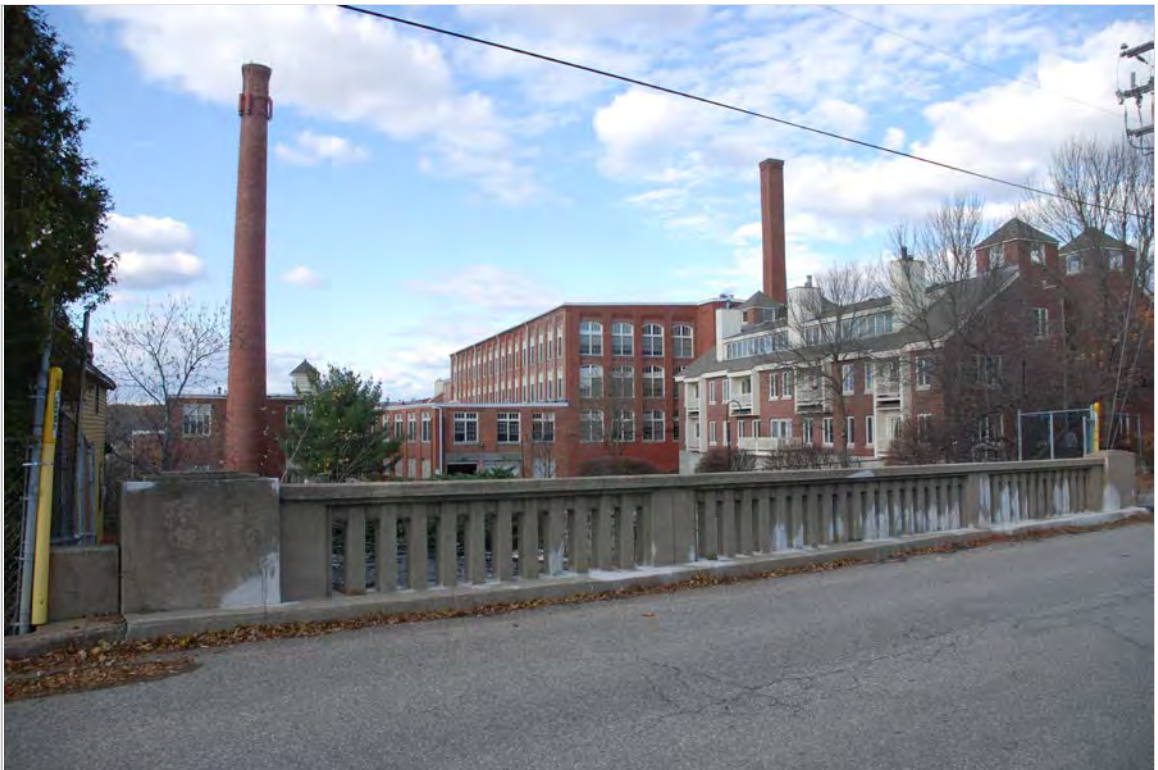
Photo 30 description: Former Exeter Manufacturing Company buildings from String Bridge Roll: Frame: Direction: NR Date taken: 11-2011 Negative stored:
