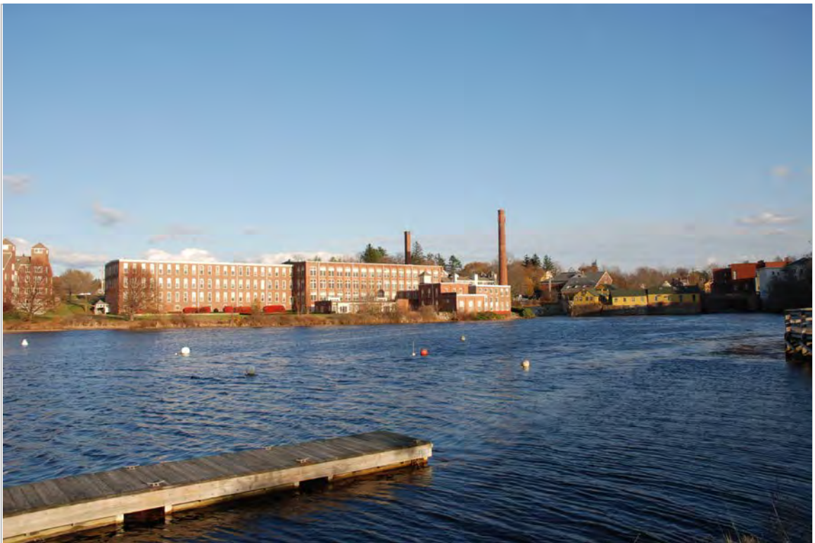
Photo 6 description: Exeter Manufacturing Company and Kimball Island buildings
