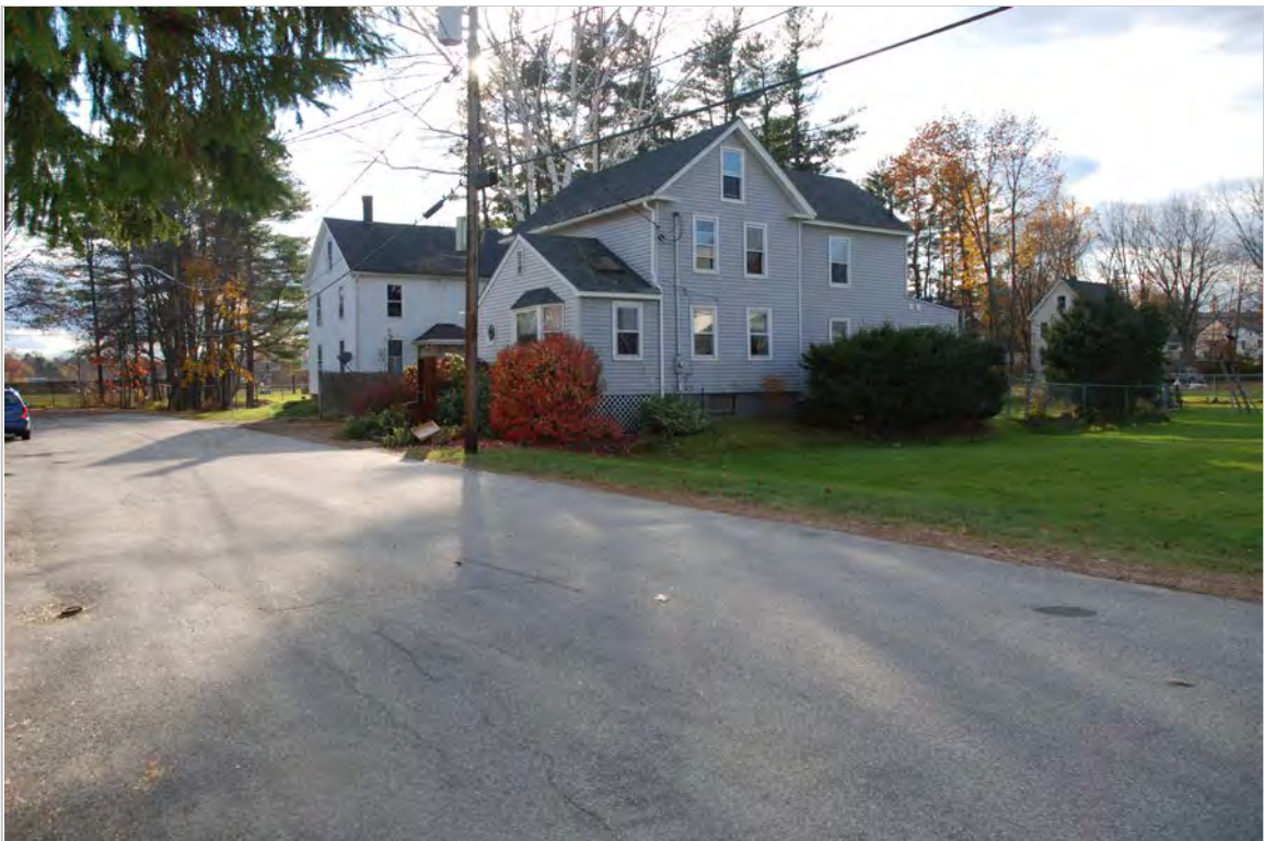
Photo 74 description: 25-27 and 31 River Street, facing southwest
