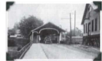
2 Thompson Covered Bridge
