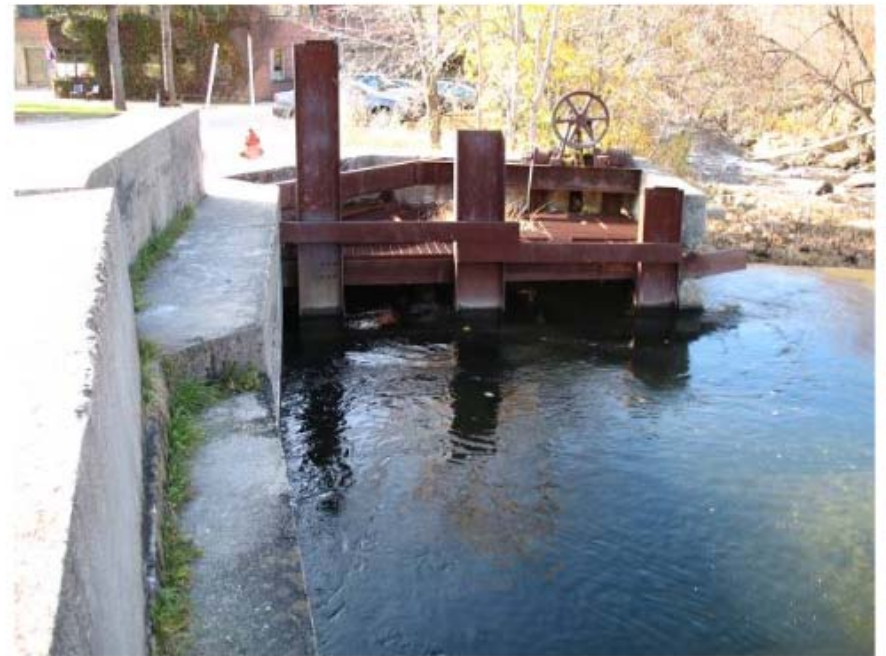
Outlet gear works (to be preserved in situ)
