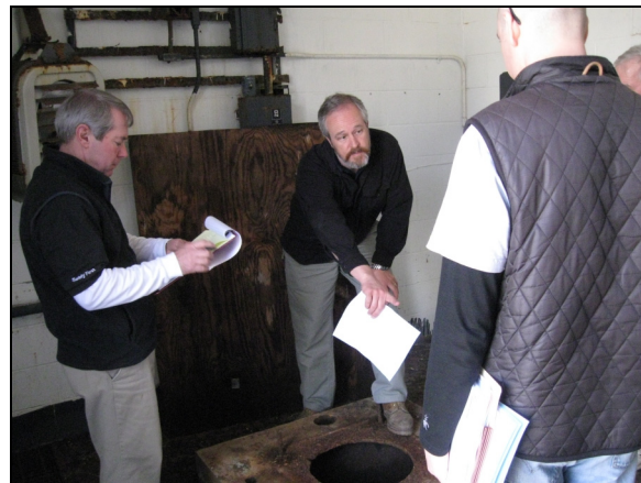
Well Inspection Prior to Rehabilitation in 2009
