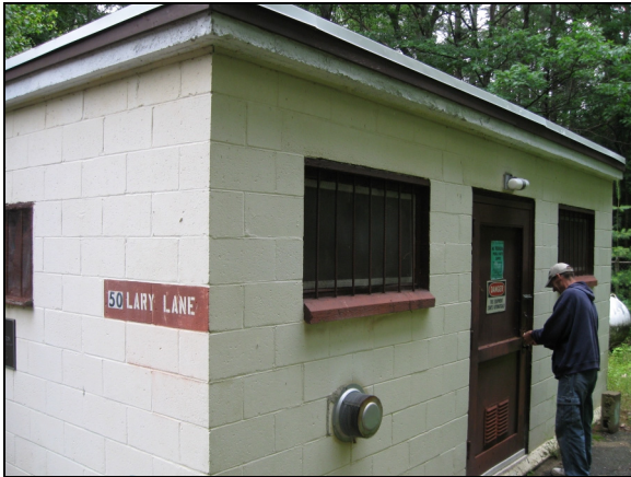
The Lary Lane Well Pumphouse
