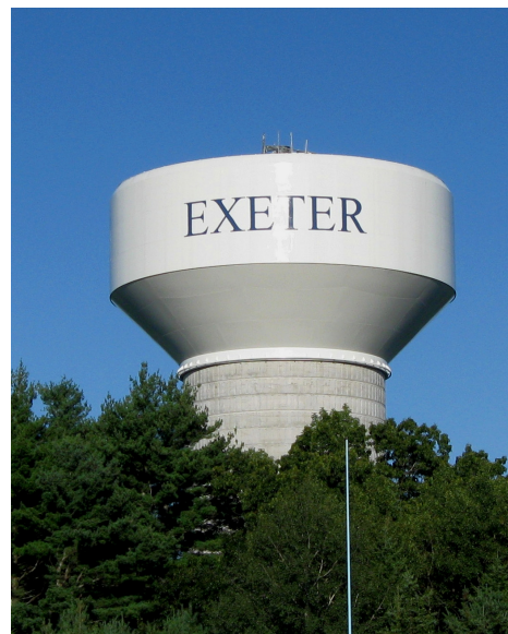
New Epping Road Water Tank Installed in 2008
