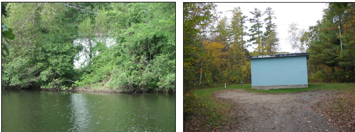
River Intake Area and Pumping Station
