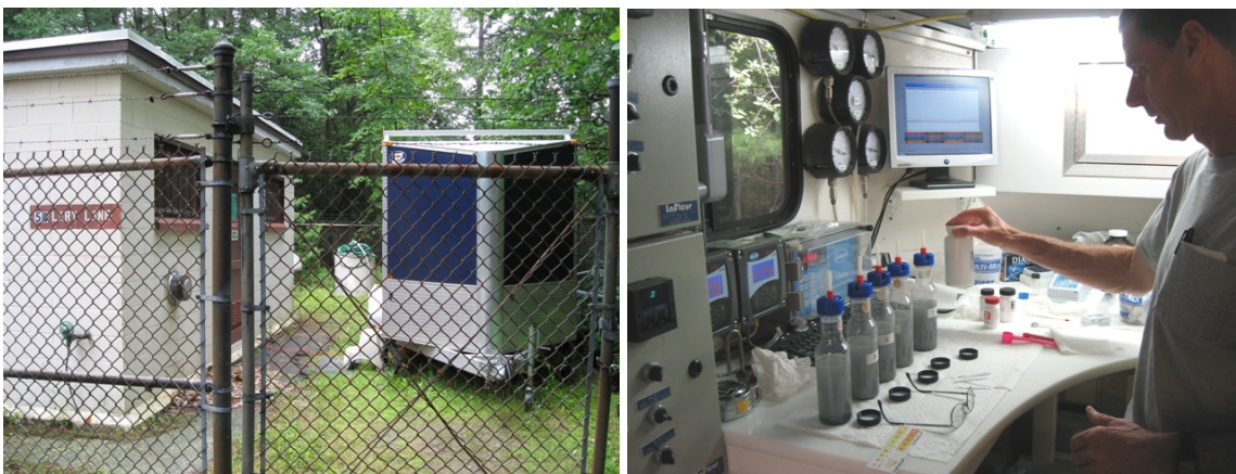
Piloting a Groundwater Pressure Filtration System at the Lary Lane Well
