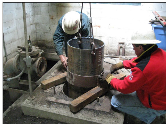
Installing a New Screen and Casing in 2009
