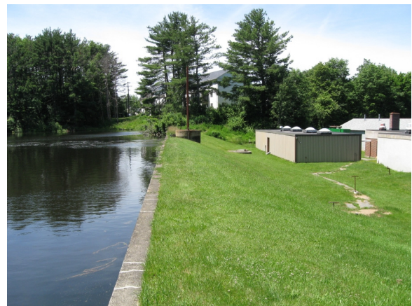
Reservoir Dam and Intake Chamber
