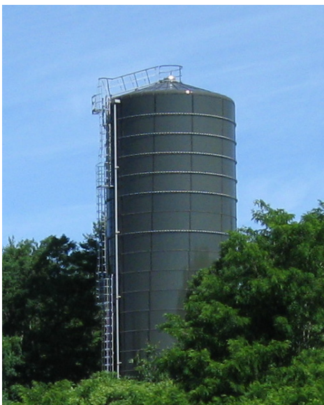
The Kingston Road Standpipe
