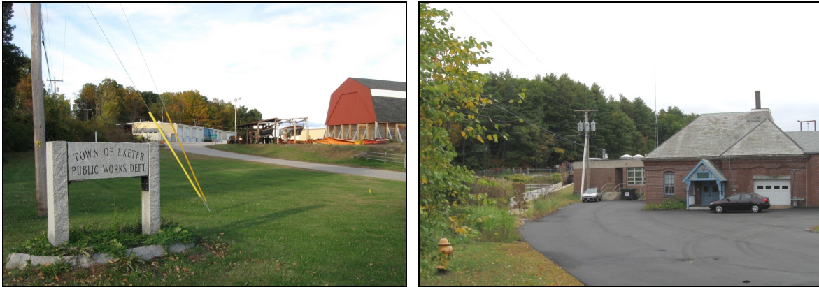
Exeter's Public Works and Surface Water Treatment Facilities
