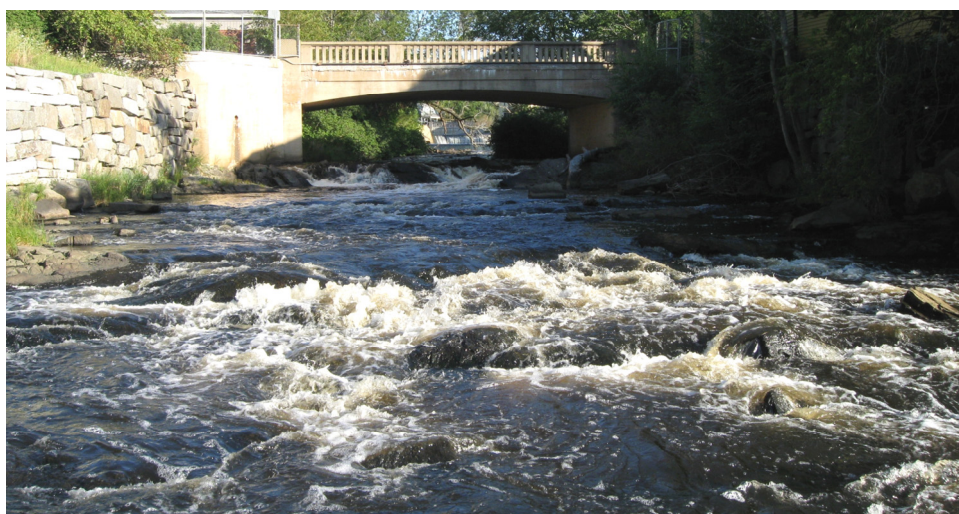
Bedrock Streambed Area Downstream of the Great Dam and String Bridge
