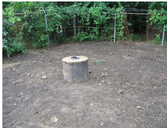
Stadium Well Restoration
