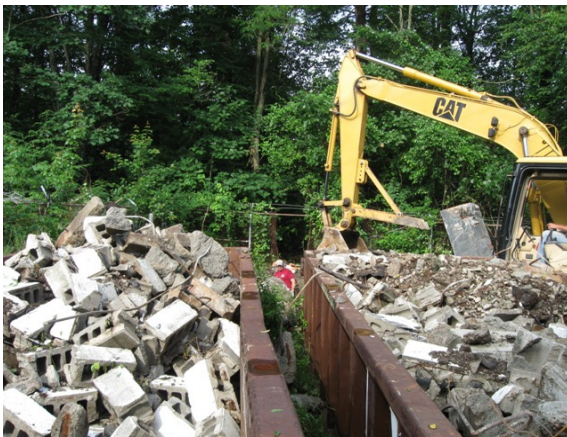
Demolition of the Stadium Well Pumphouse
