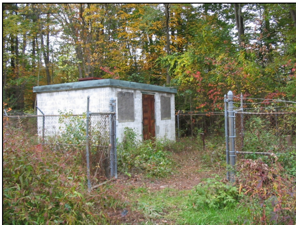
Stadium Well Pumphouse in 2009
