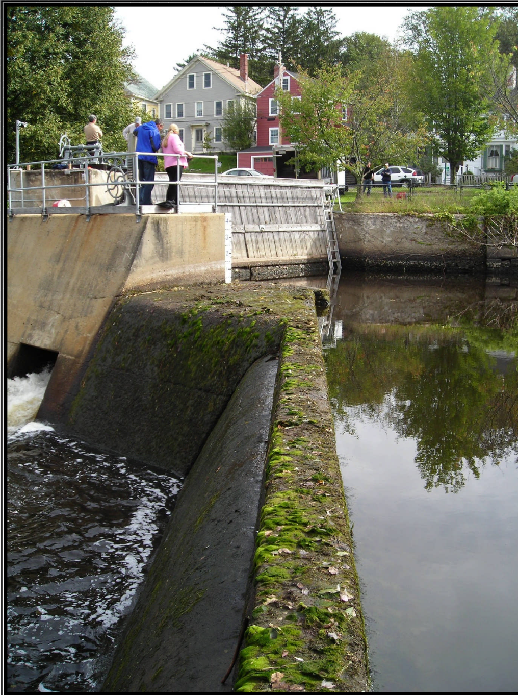
Great Dam looking northeast
