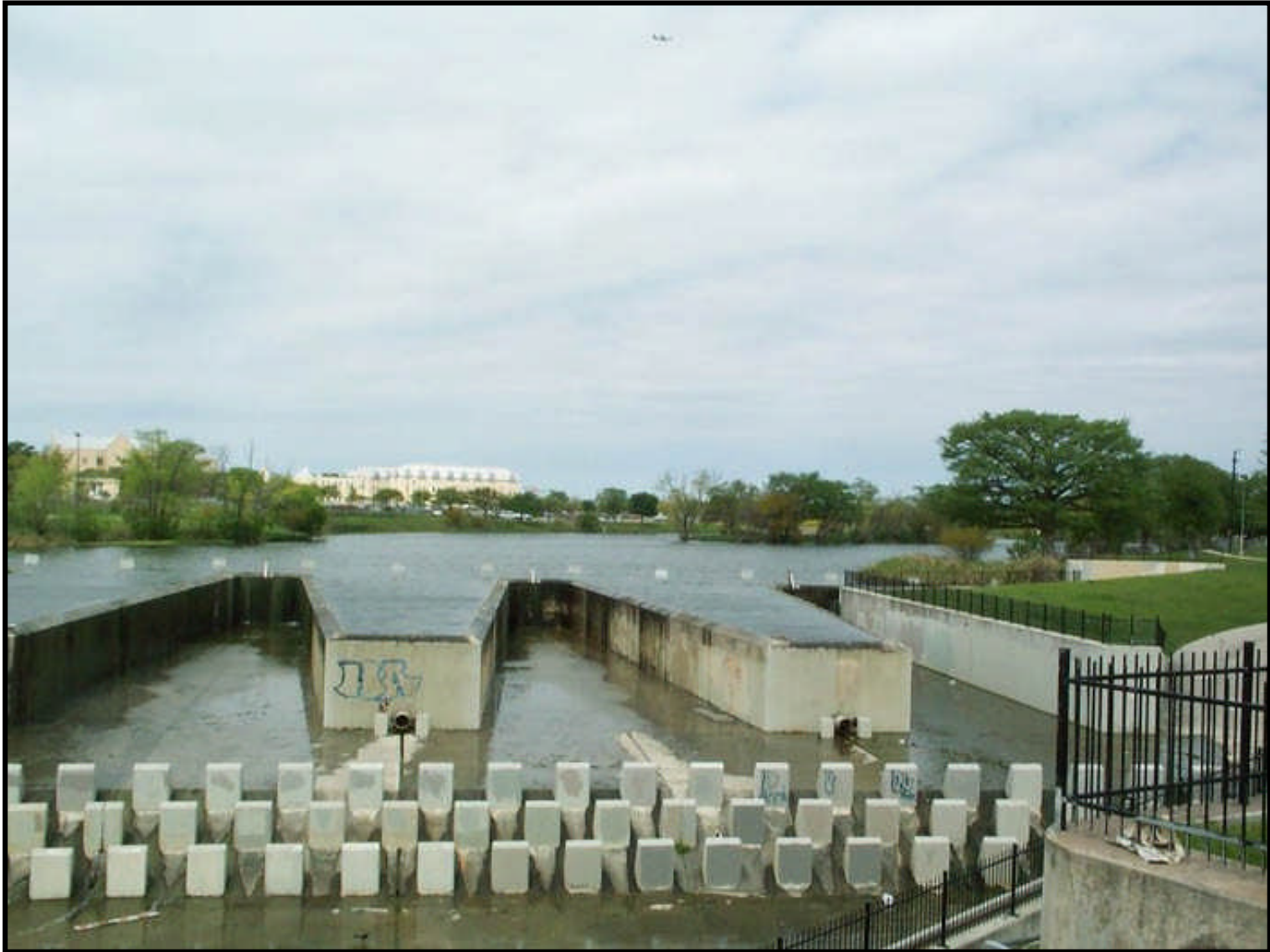
Labyrinth Weir Style Dam
