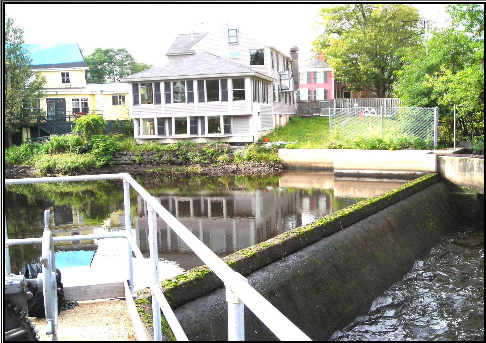
Great Dam looking southwest
