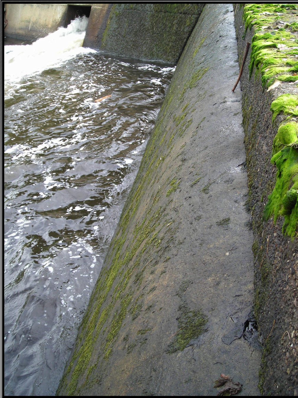
Downstream face of Great Dam
