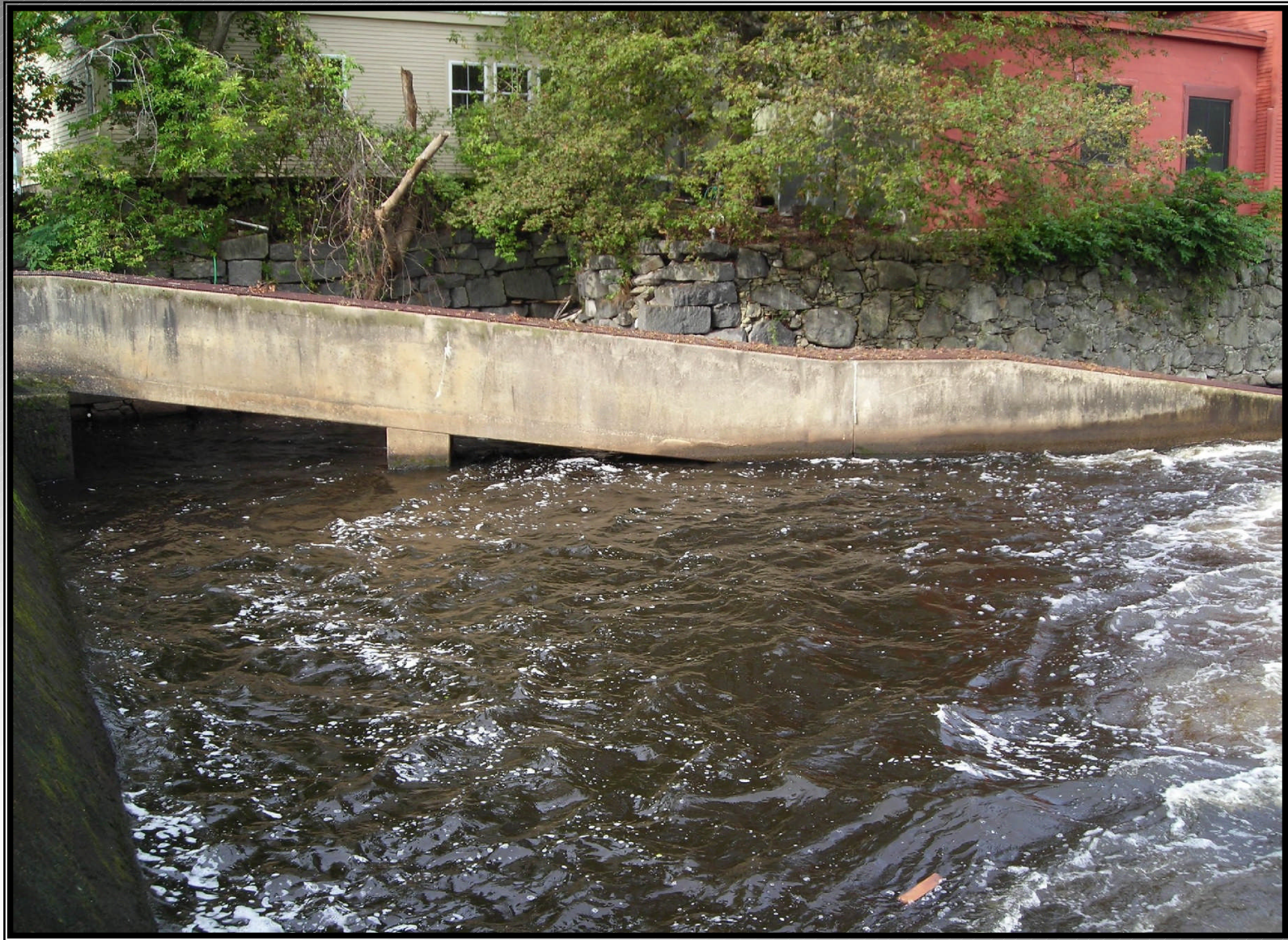
Great Dam Fish Ladder
