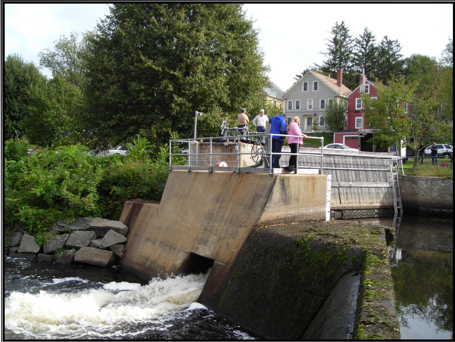
Great Dam Low Level Gate
