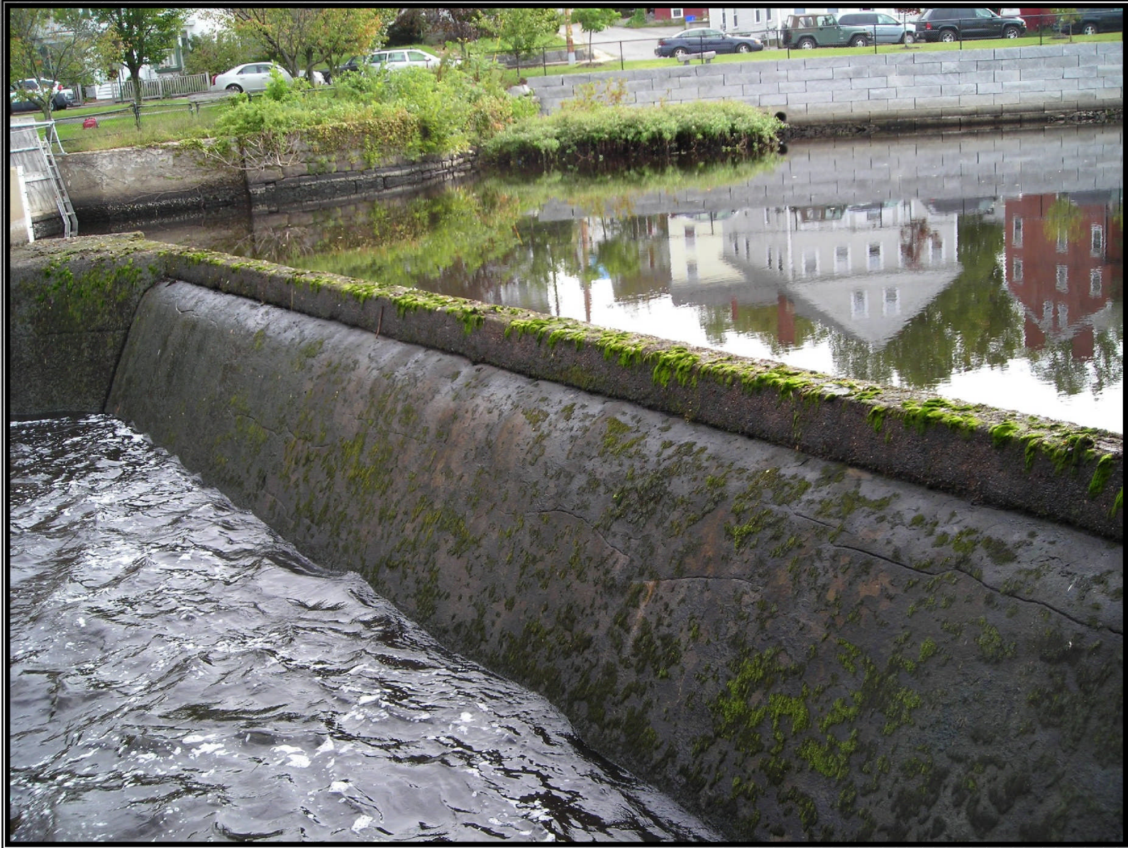
Great Dam downstream face
