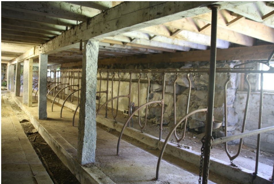
Photo 53) Milking stanchions, south wall, looking east
