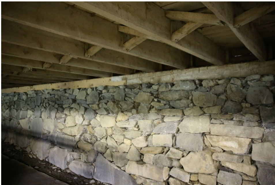
Photo 55) Interior of north foundation wall, reconstructed in 2004 Direction: NNW
