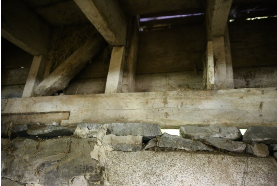
Photo 58) North foundation wall and sill, replaced sill Direction: N
