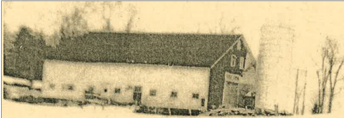
South and east elevations and silo under construction. Historic photo ca. 1958
