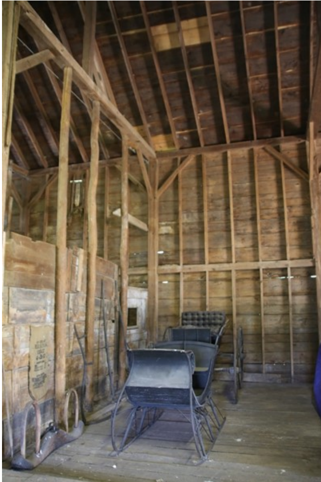
Photo 33) North aisle, hay storage area Direction: NNW
