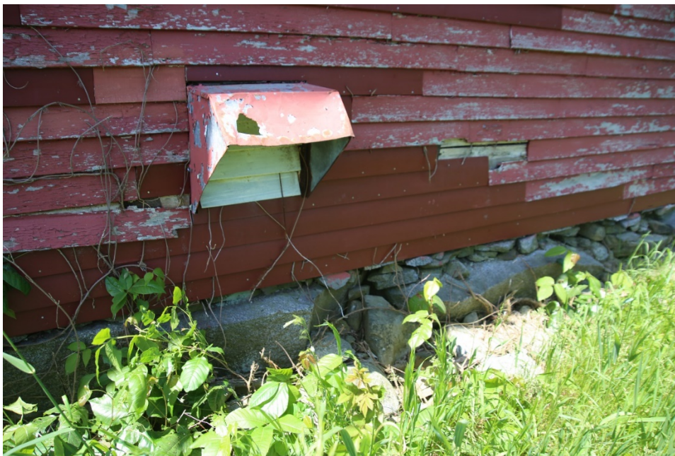
Photo 16) North elevation, ventilator hood
