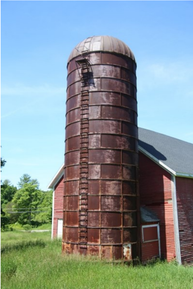
Photo 9) Silo Direction: WSW
