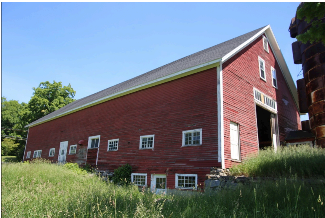
South and east elevations, 2018
