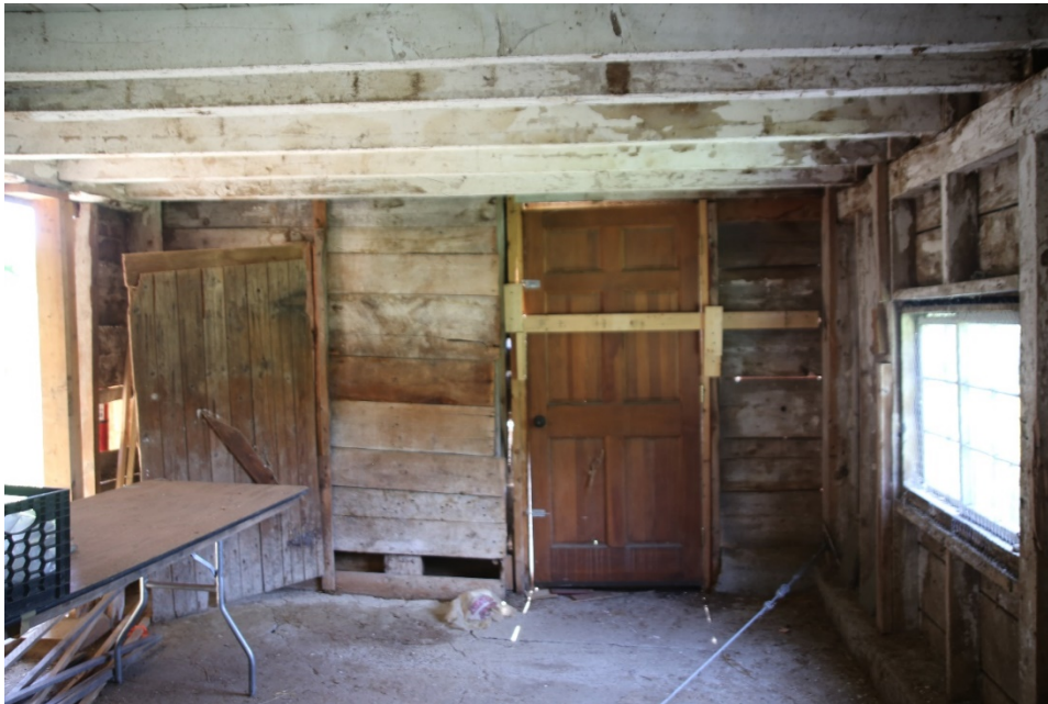
Photo 43) Southeast corner and wall, whitewashed privy area, showing 1960s residential door Direction: E
