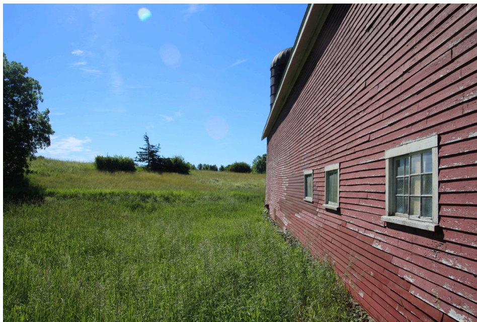
North elevation after repairs to foundation, 2018
