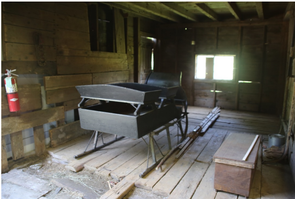
Photo 30) Northwest corner, carriage storage area Direction: NNW
