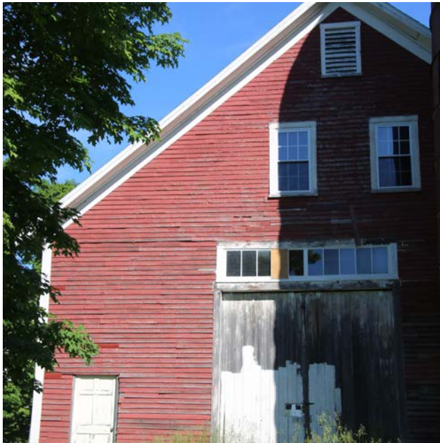
Photo 6) East elevation showing central bay drive doors Direction: W
