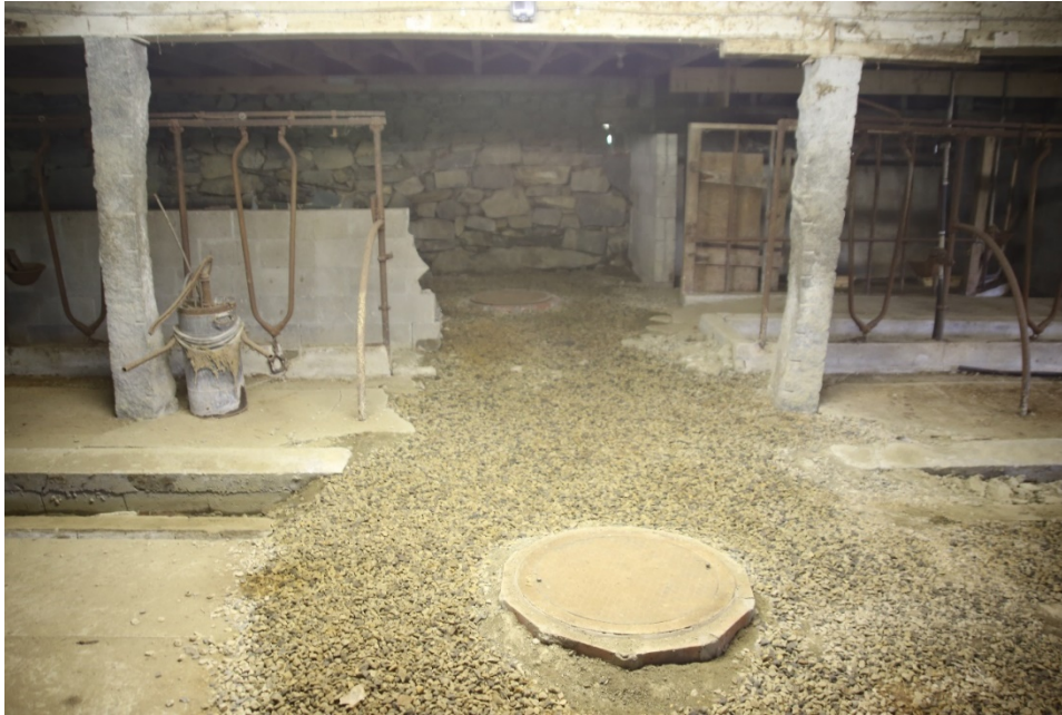
Photo 64) Basement milking area floor, showing stormwater drainage system in floor installed in 2004
