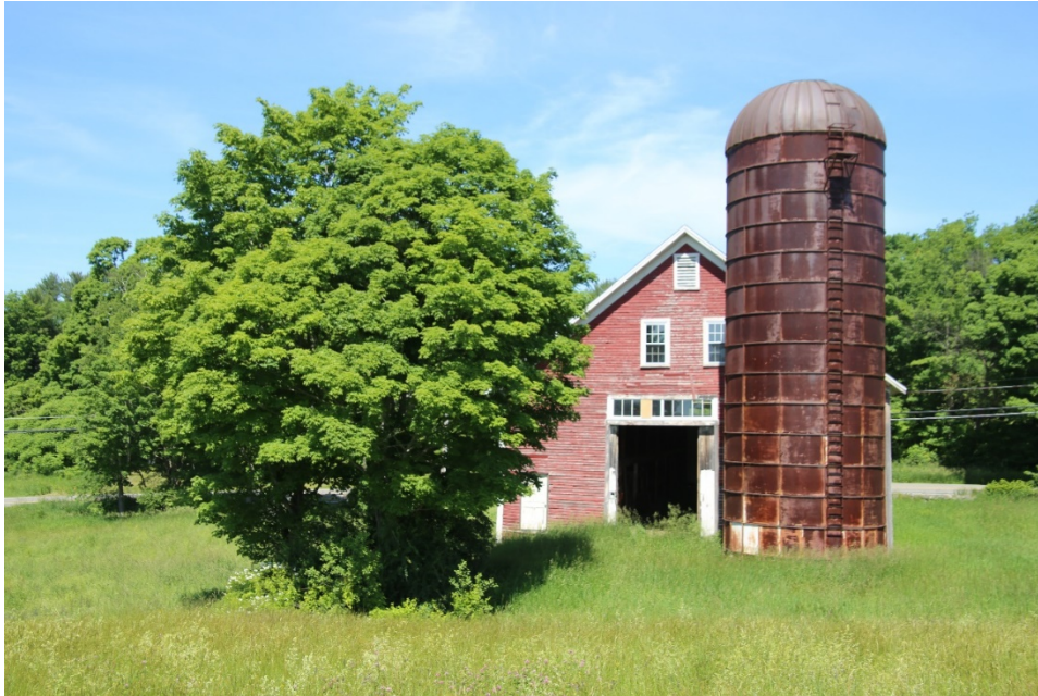
Photo 5) East elevation and silo Direction: W
