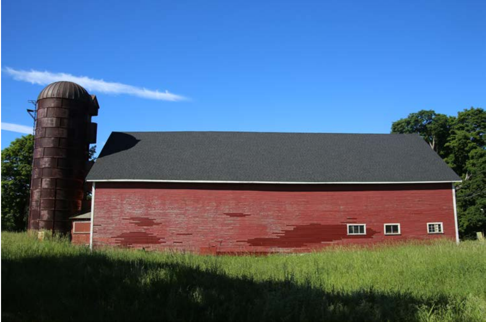
Photo 10) North elevation Direction: S
