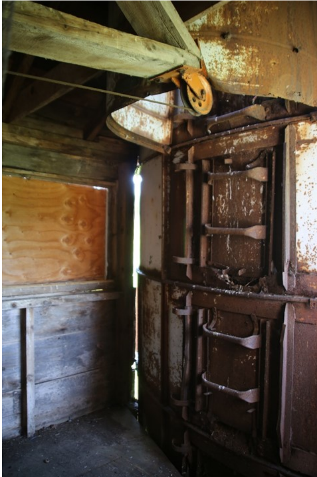
Photo 46) Silo ladder within connector Direction: NNE
