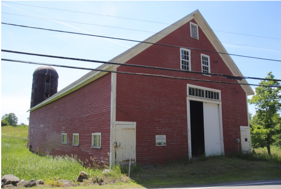
Photo 1) North and west elevations, from Newfields Road Direction: SE
