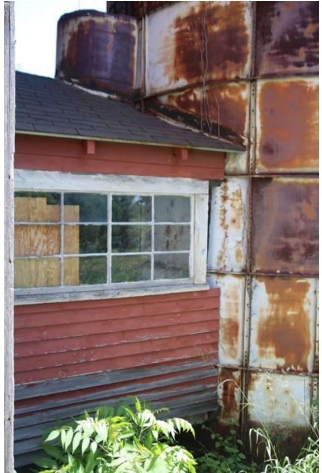
Photo 24) Silo connector, south side Direction: NE
