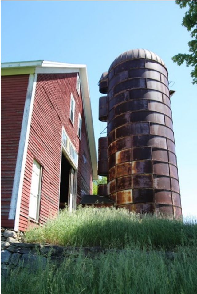
Photo 7) East elevation and silo, from the south Direction: NW
