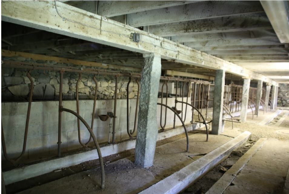
Photo 54) Milking stanchions, north wall, looking east Direction: NE
