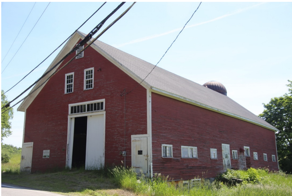
Photo 2) West and south elevations, from Newfields Road Direction: NE
