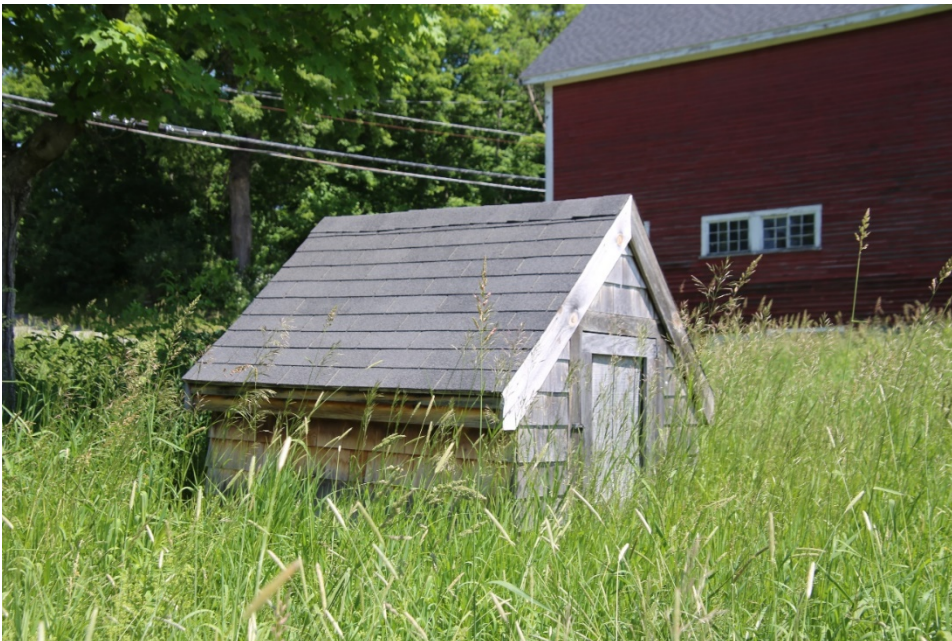
Photo 12) Pump house Direction: NW
