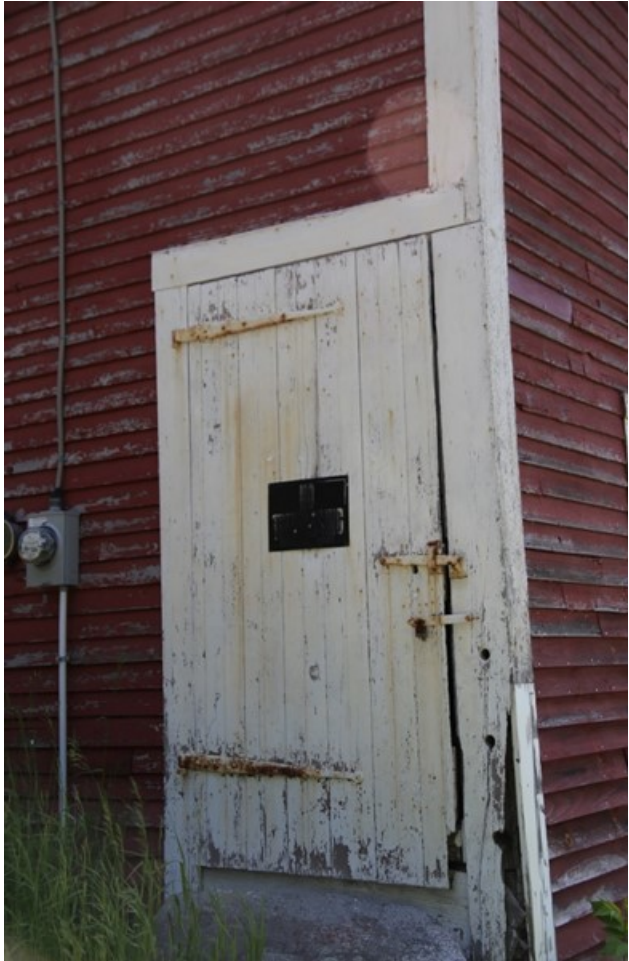
Photo 19) West elevation, door at south end Direction: NE
