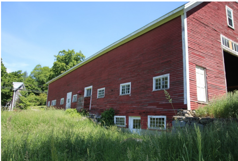
Photo 4) Southeast corner, south elevation
