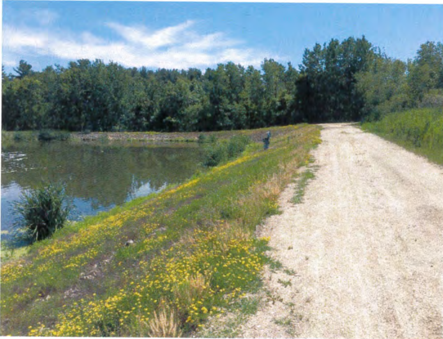
Easterly perimeter road location. SW corner of lagoon 3 to be utilized for stormwater and fire protection.
