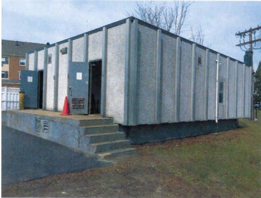
Main Pump Station Building
