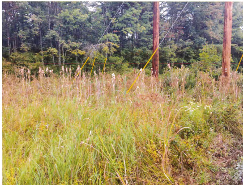
Photograph No. 6: Looking easterly at A126 Structure 186 guy wires to be replaced.
