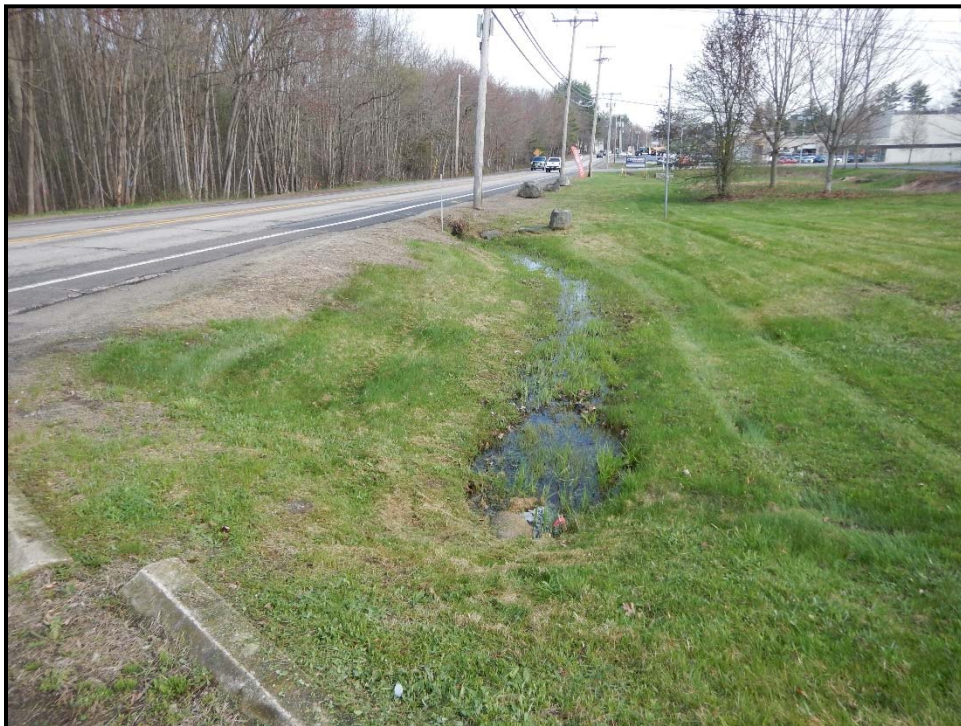
Photo 6: View southeast toward wetland W-03, located west of Epping Road and south of a driveway to an auto repair shop.
