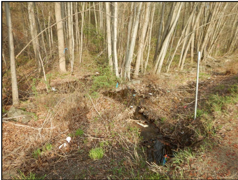
Photo 4: View northeast of the intermittent stream entering wetland W-01 from the culvert underneath Epping Road.
