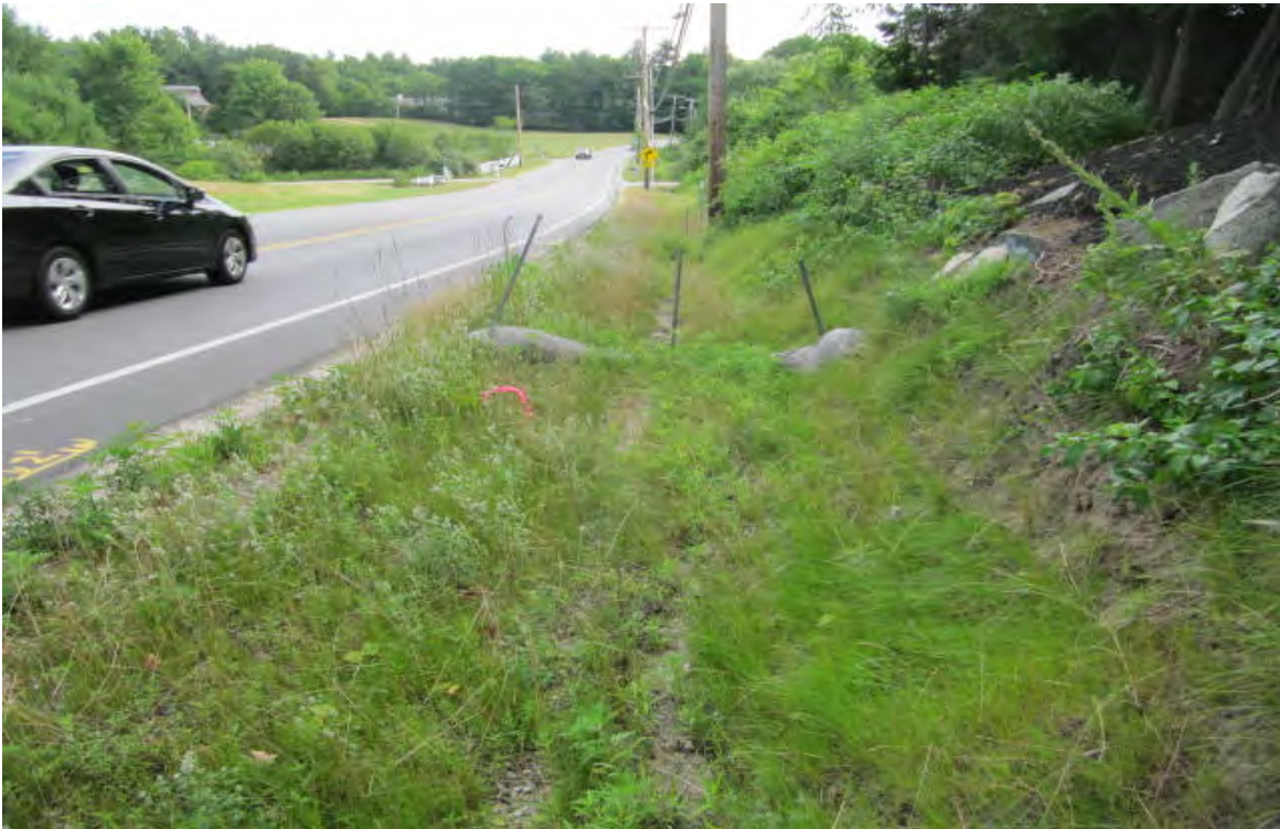
Photo A-1. Easterly view of drainage ditch along the south side of Kingston Road.
