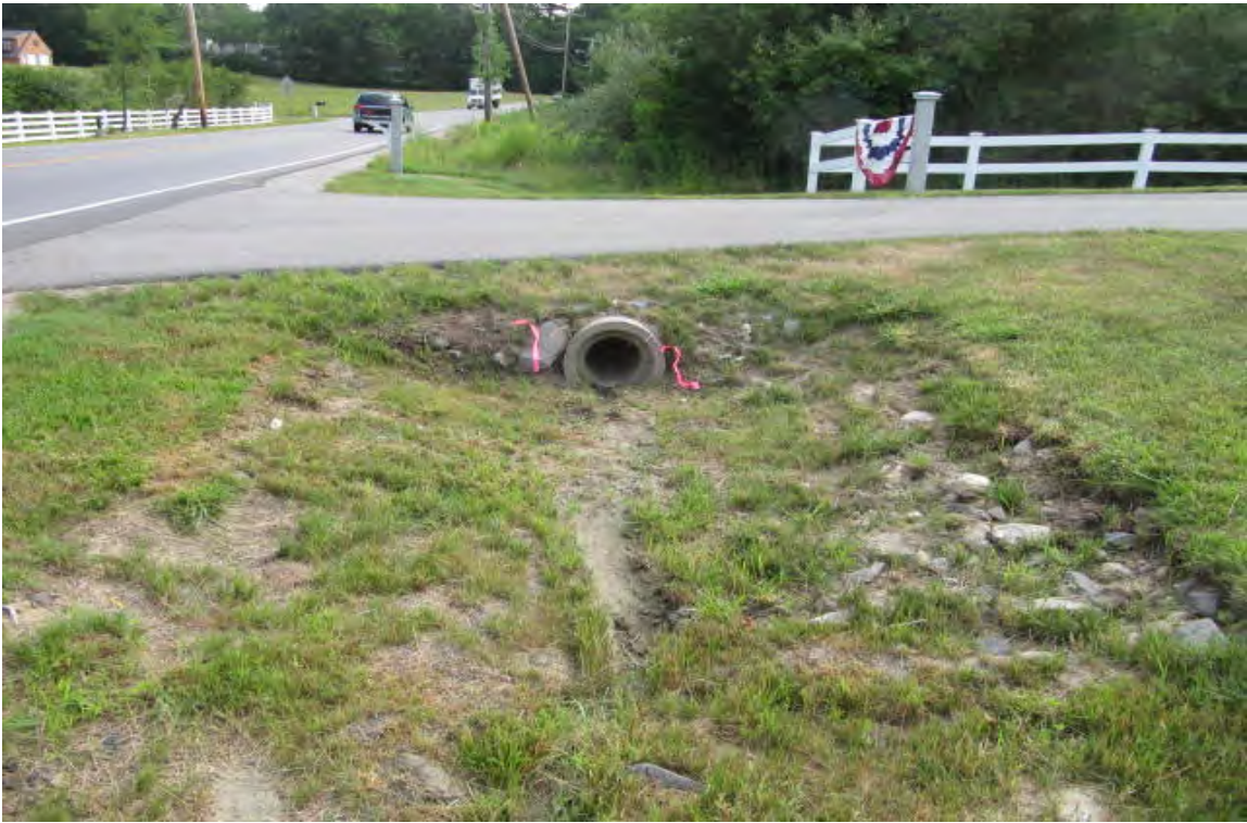
Photo A-2. 12” cp that wetland A drains through into wetland B.
