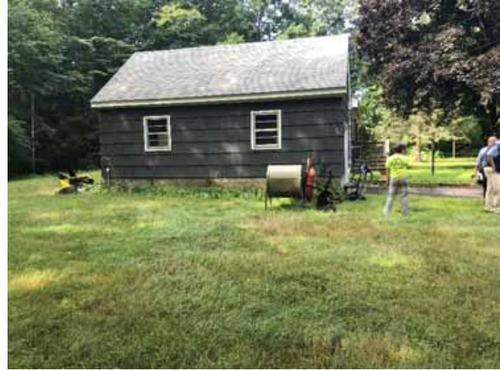
Photo 2: East side of the attached garage, facing west.
