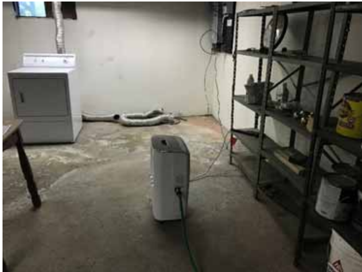
Photo 11: Dryer, dehumidifier, and shelf storage located in the basement.
