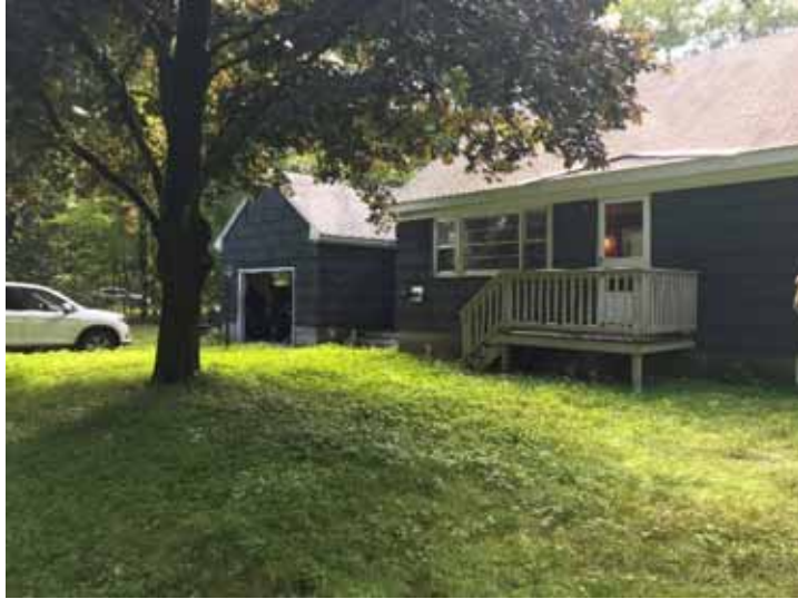
Photo 1: North side of the residence, facing southeast.
