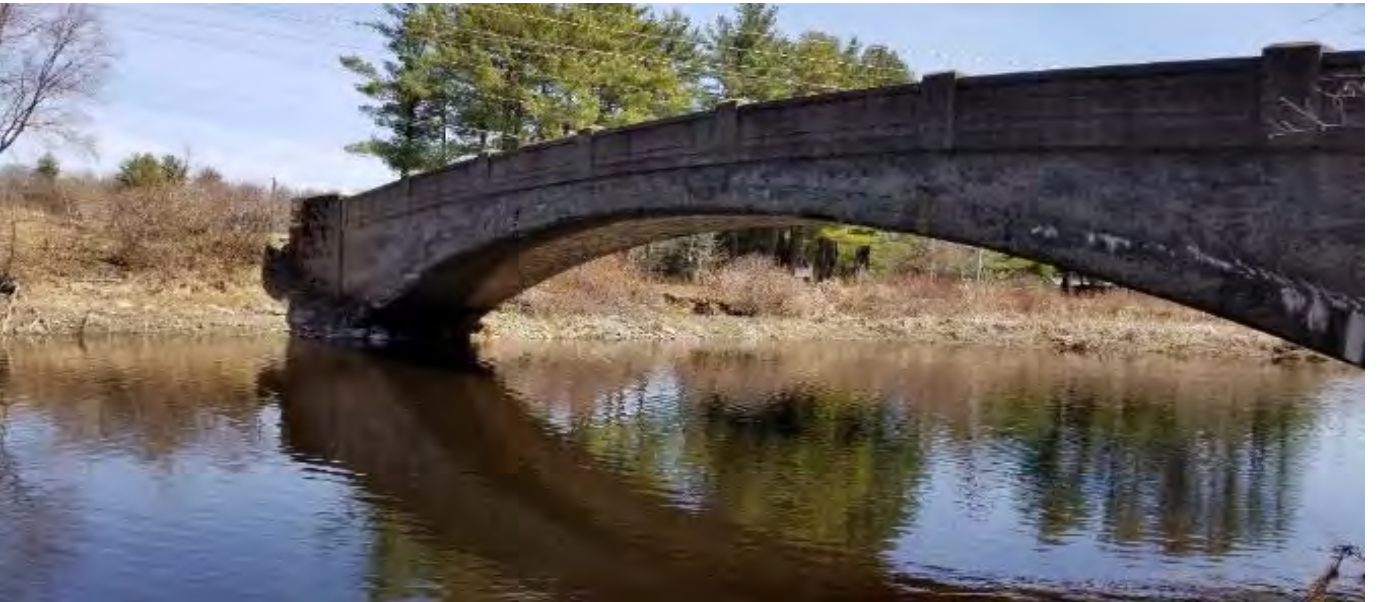
Photo No. 2 Description: Overview of bridge downstream face Photo Date: 4/24/2018
