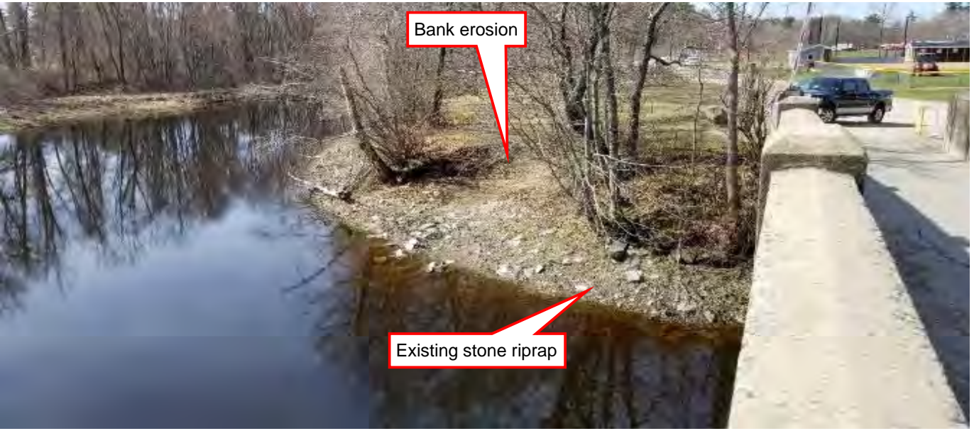
Photo No. 4 Description: Upstream left river bank Photo Date: 4/24/2018
