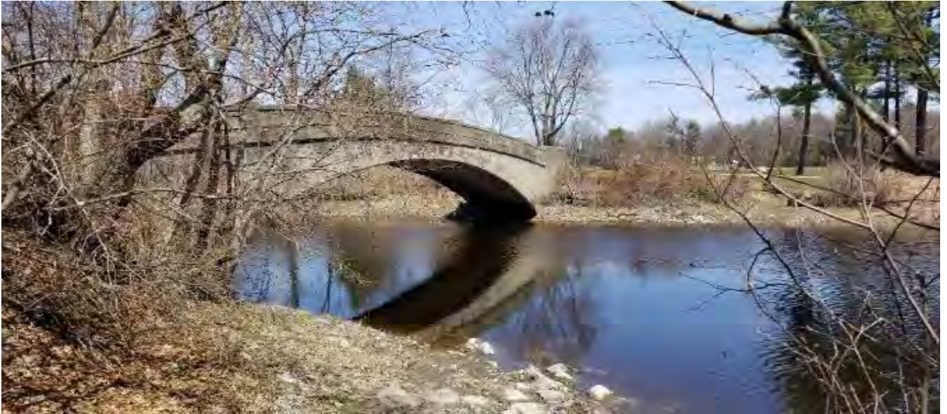
Photo No. 1 Description: Overview of bridge upstream face Photo Date: 4/24/2018
