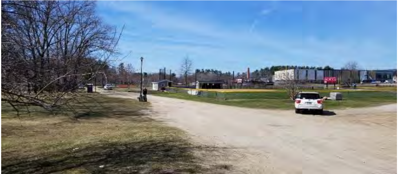
Photo No. 9 Description: Overview of area left (southwest) of bridge Photo Date: 4/24/2018
