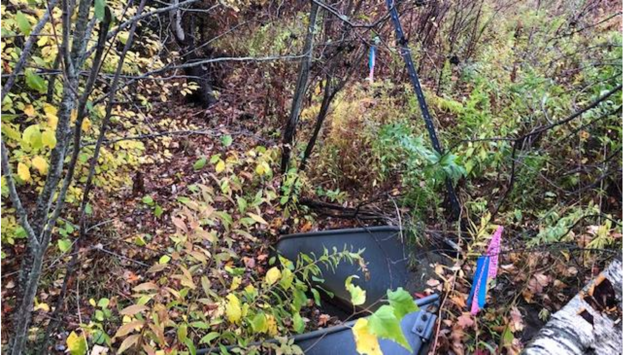
Photo #1 Looking at the culvert inlet that extends under Holland Way
