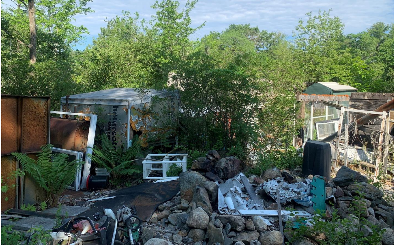
Photo #5: Looking at the extensive debris on site.
