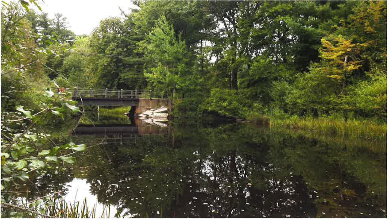
Photo 2: Little River and Garrison Lane Bridge (Facing Northeast)
