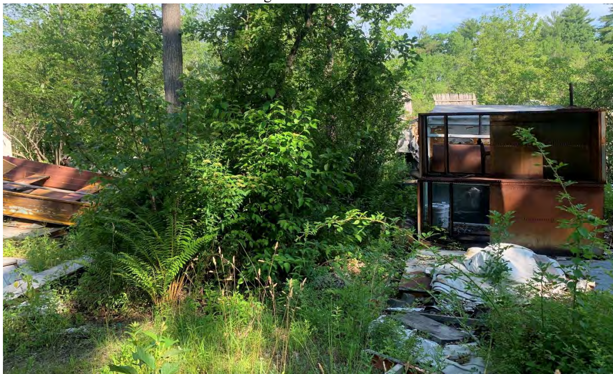
Photo #6: Looking at the debris mixed with the thick vegetation.
