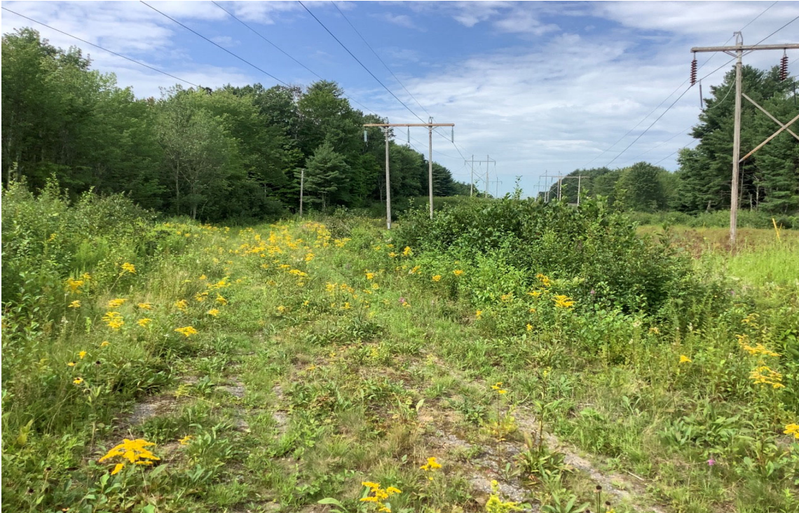
Photo 2. View southwest at approximate location where new Structure 176 will be installed and where a temporary work pad will be required. Portions of the work pad will require matting within Wetland W31 and the associated combined buffer of Wetland W31 and W32.
