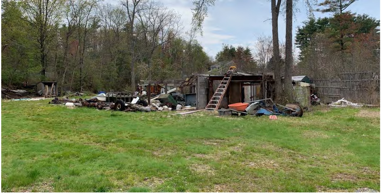
Photo #3: Looking to the west at another building and associated debris/trash that extends into the wetlands.
