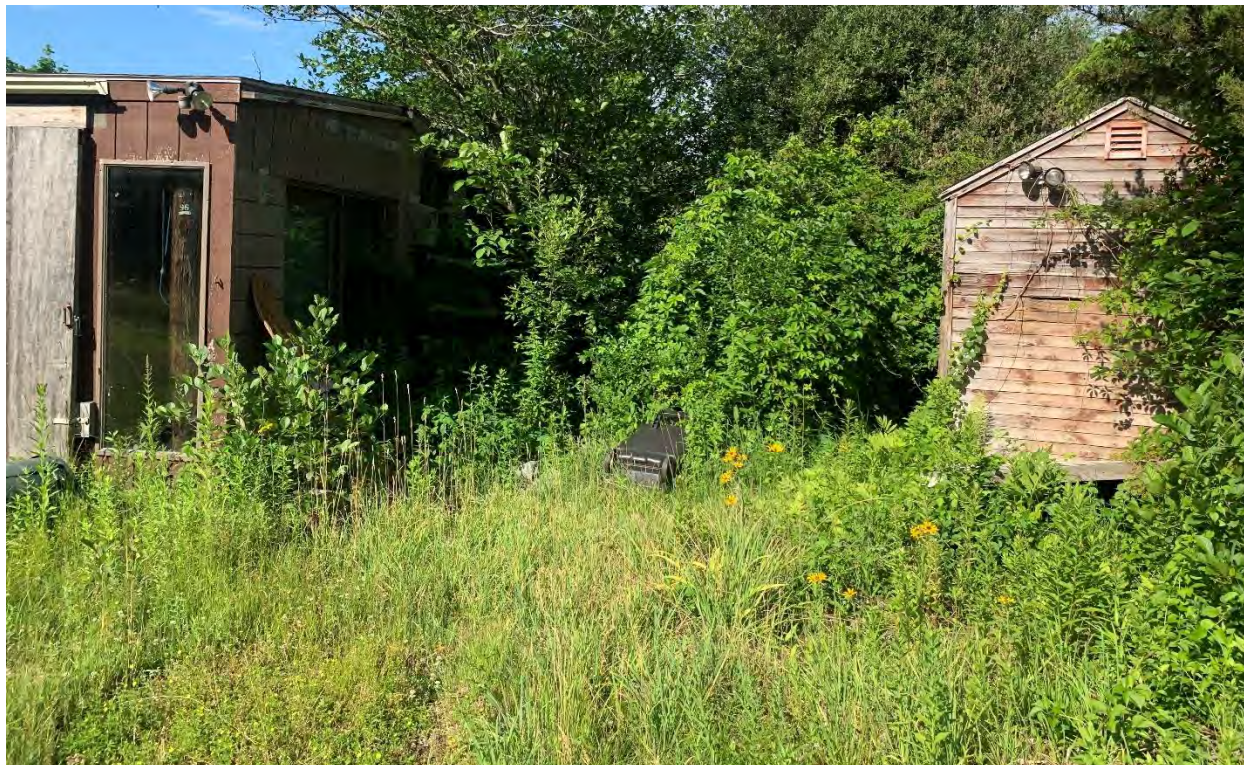
Photo #3: Looking at the thick vegetation between two of the structures on site
