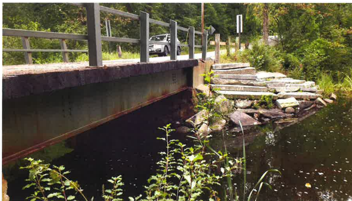
Photo 2: Work Area (Facing East)
