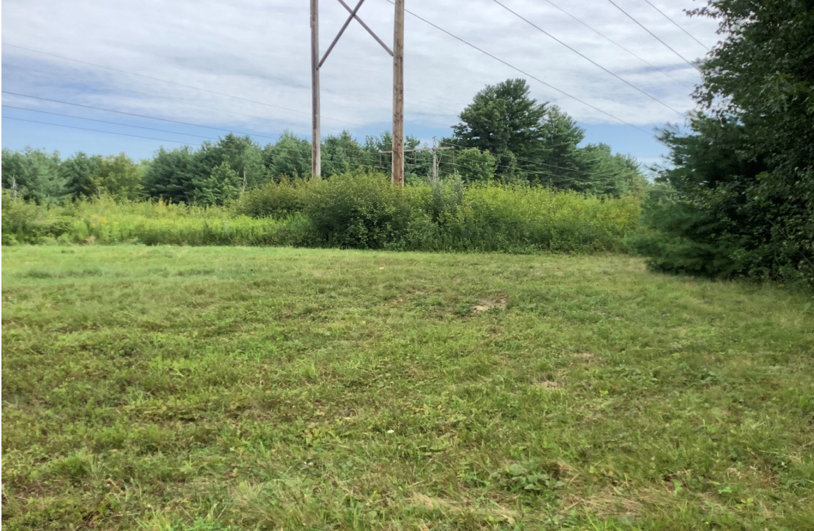
Photo 1. View northeast at existing Structure 177 to be replaced within the 300 foot shoreland buffer of the Little River in Exeter. Structure 177 is located immediately north (downslope) of Route 101 WB.
