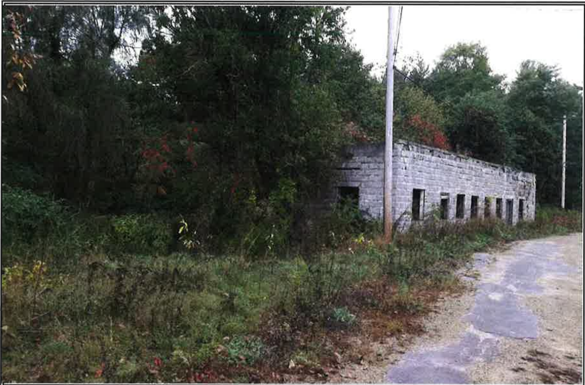
Photograph 3 - View facing north of former packing building. (StoneHill, October 11, 2017)
