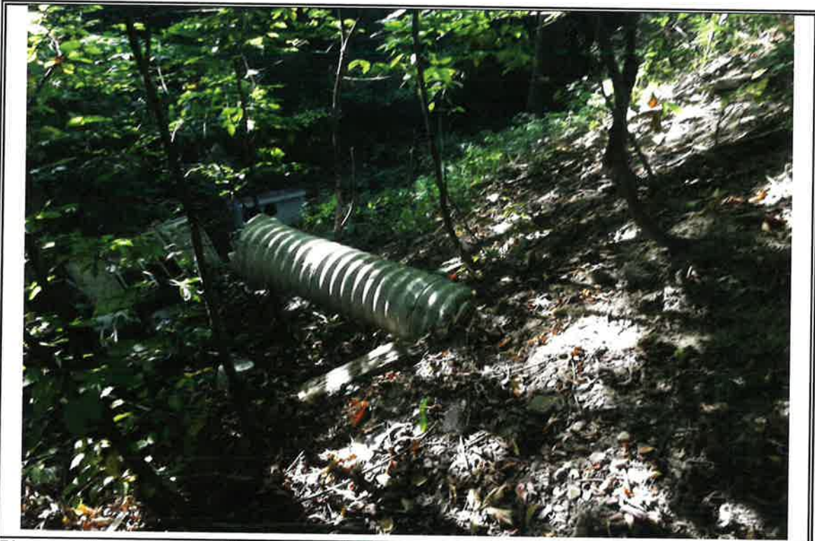
Photograph 7 - View west of 12-inch pipe behind former packing building. (StoneHill, September 26, 2016)
