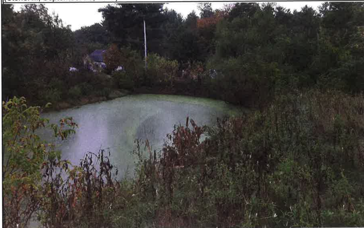
Photograph 10 - View looking west of Basin #4. (StoneHill, October 11, 2017)
