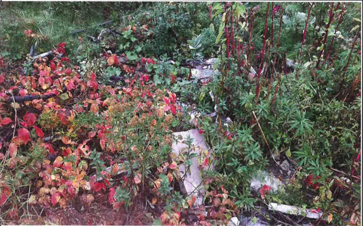
Photograph 14 - View of concrete in GH Area. (StoneHill, October 11, 2017)
