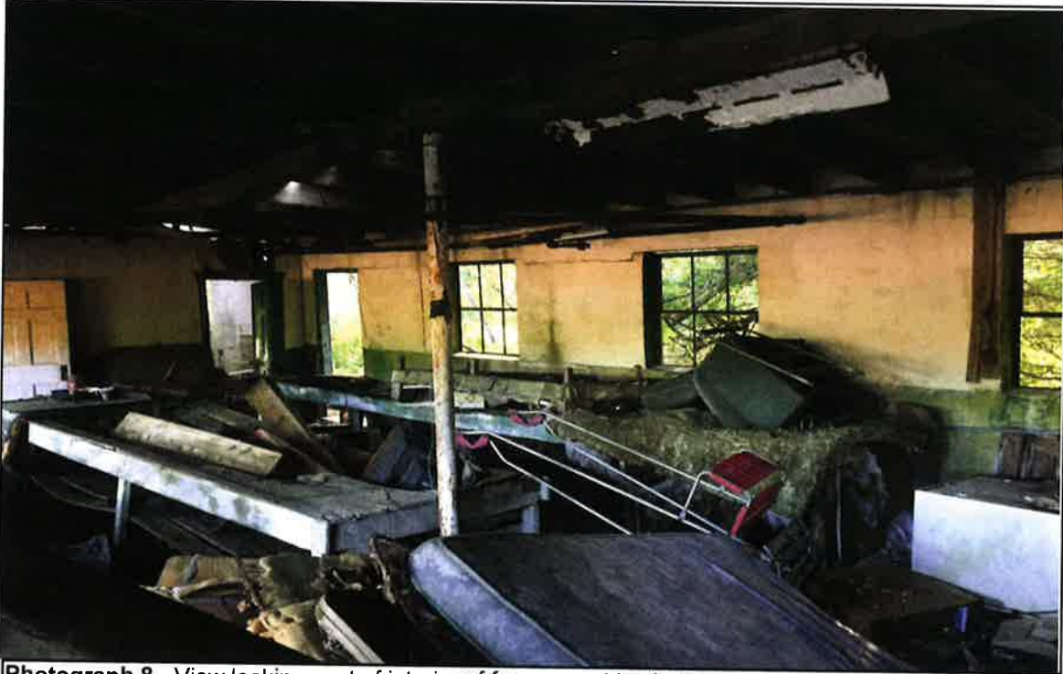
Photograph 8 - View looking east of interior of former packing building. (StoneHill, September 26, 2016)
