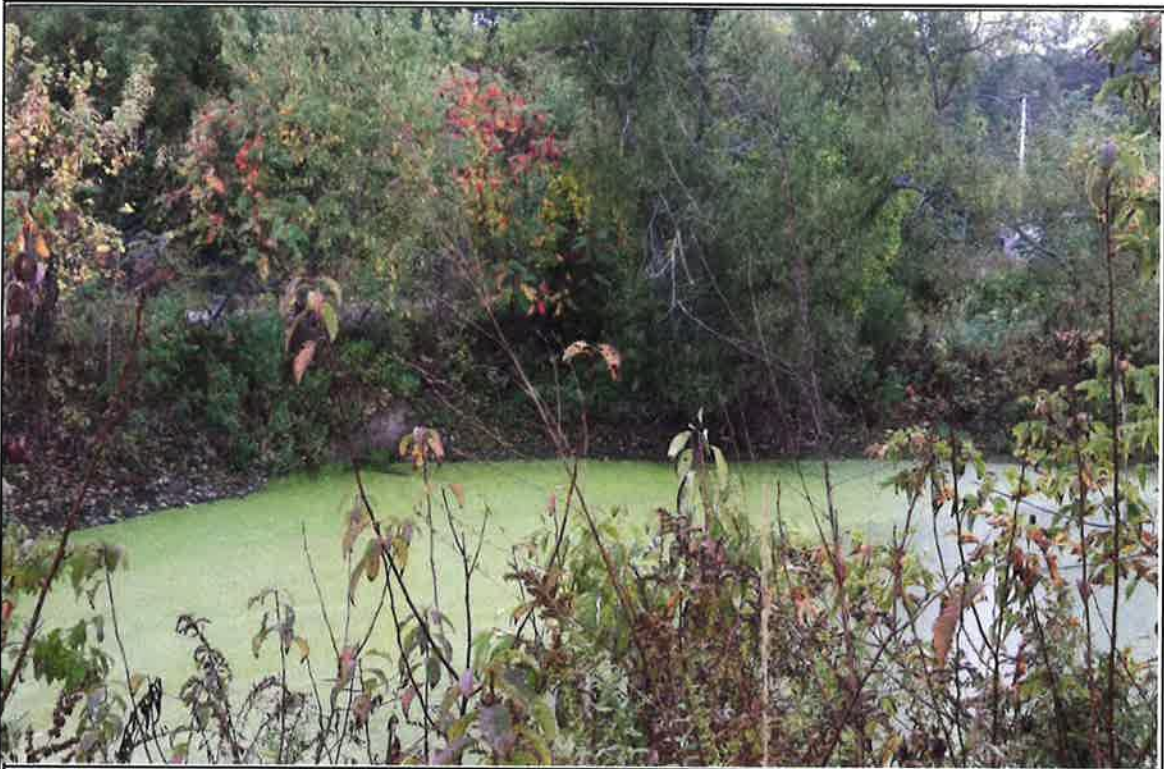
Photograph 11 - View looking west of 12-inch culvert in Basin #4. (StoneHill, October 11, 2017)
