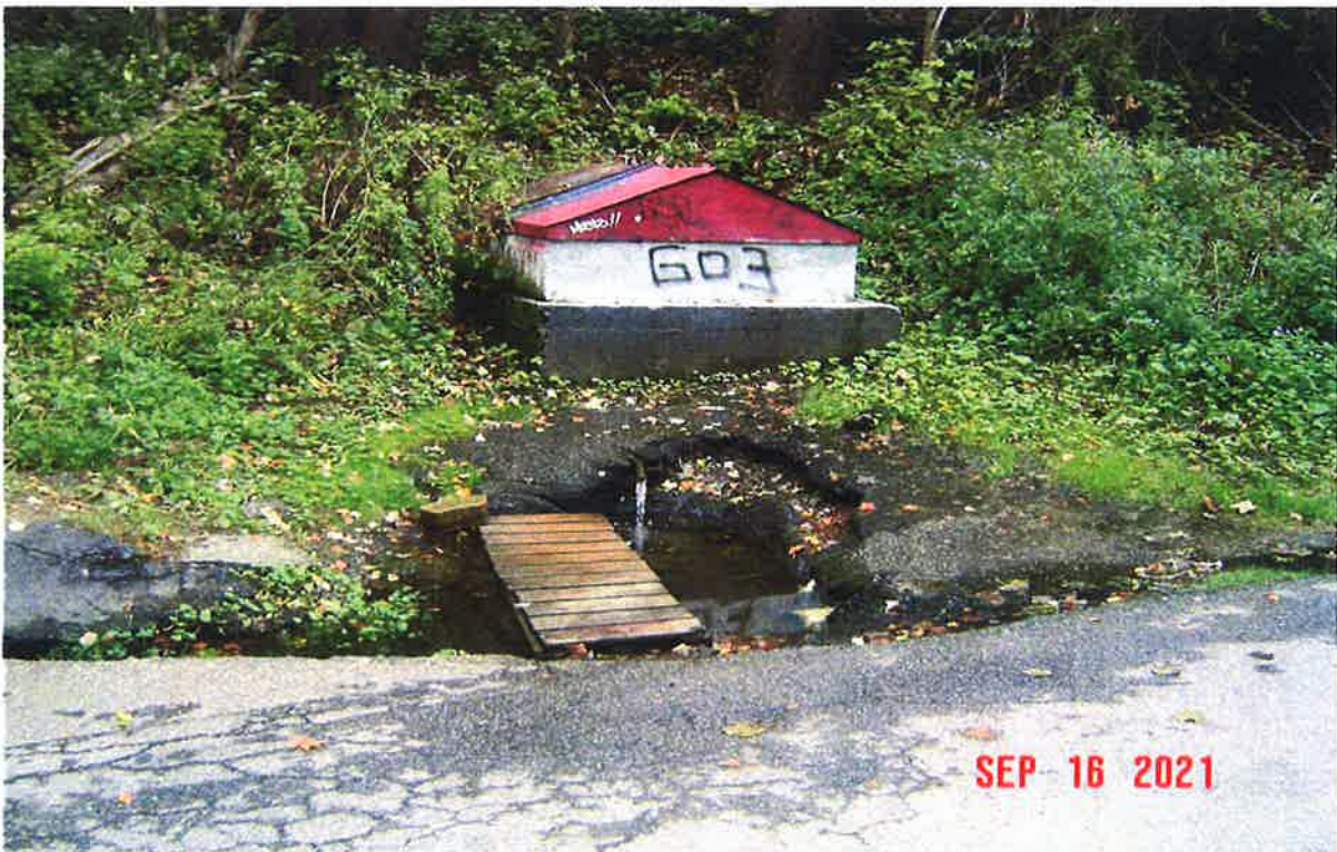
Image 34 – Looking east at the 'Jailhouse Spring' house. Refer to Figure 6. ©Jacobs2021
