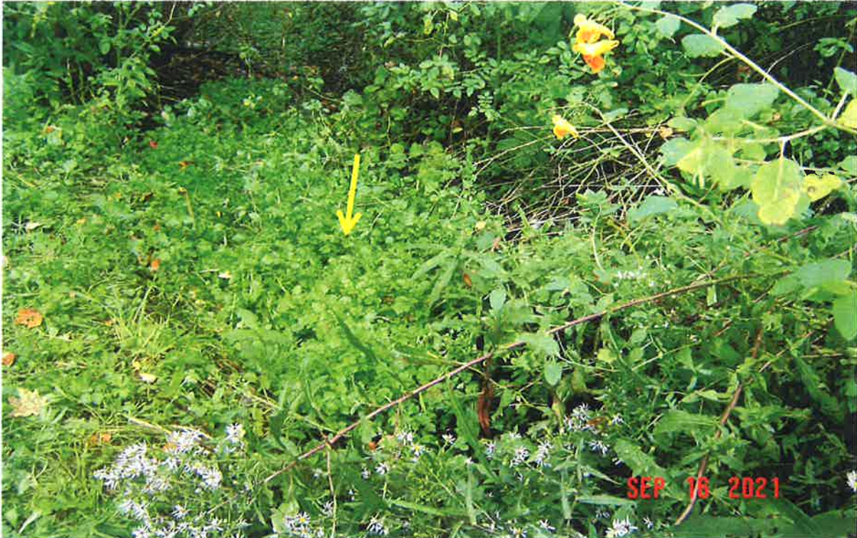
Image 25 – Looking at upstream / plugged end of culvert D2 (yellow arrow). 118 SF of impact to Wetland K proposed here for replacement of culvert D2. Refer to Figure 3. ©Jacobs2021
