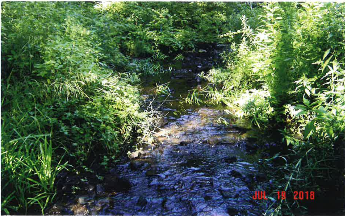
Image 2 – Looking westerly /upstream at Norris Brook from just downstream of the proposed 5' X 24' box culvert. Note the bricks in the stream. Refer to Figure 1. ©Jacobs2018
