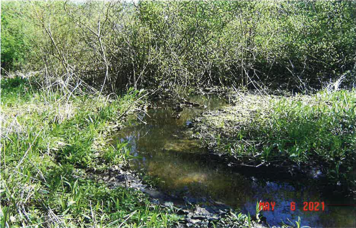
Image 15 – Looking east @ Oak St Ext (just behind dogwood shrubs) & upstream end of culvert D3. Refer to Figure 3. ©Jacobs2021
