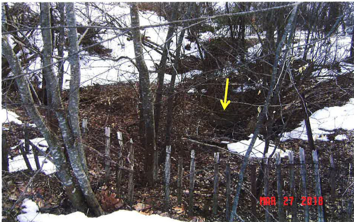
Image 14– Looking southerly at man-made Wetland H from Oak St. Ext. Note the reinforced concrete culvert section installed vertically (yellow arrow). Refer to Figure 2. ©Jacobs2018
