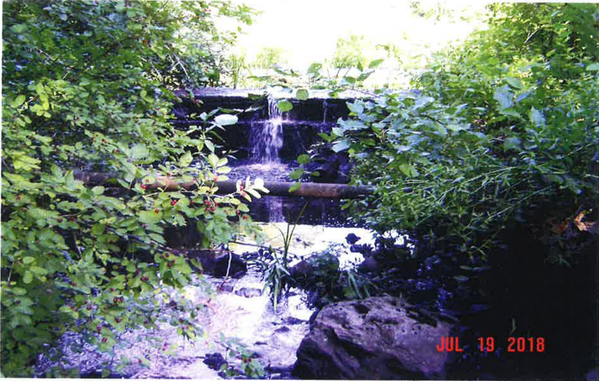
Image 5 – Looking westerly at the concrete weir from Norris Brook. Note the pipe in foreground and impounded man-made pond in the background. Refer to Figure 1. ©Jacobs2018
