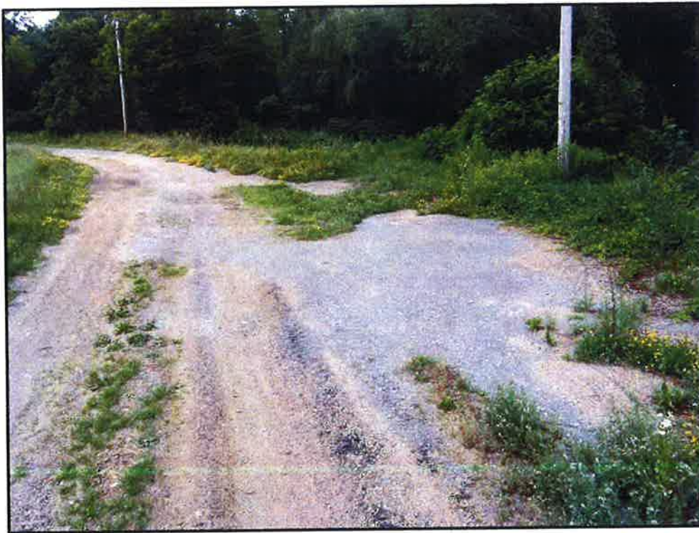
Plate 12. View Southeast of Old Asphalt Surface, Oak Street Extension
