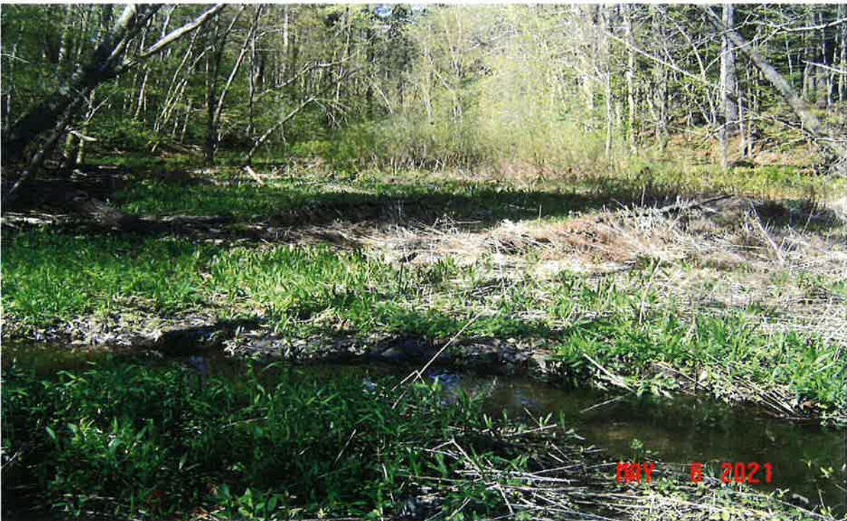
Image 16 – Looking west (upstream) from Oak St Extension at culvert D3. Refer to Figure 3. ©Jacobs2021
