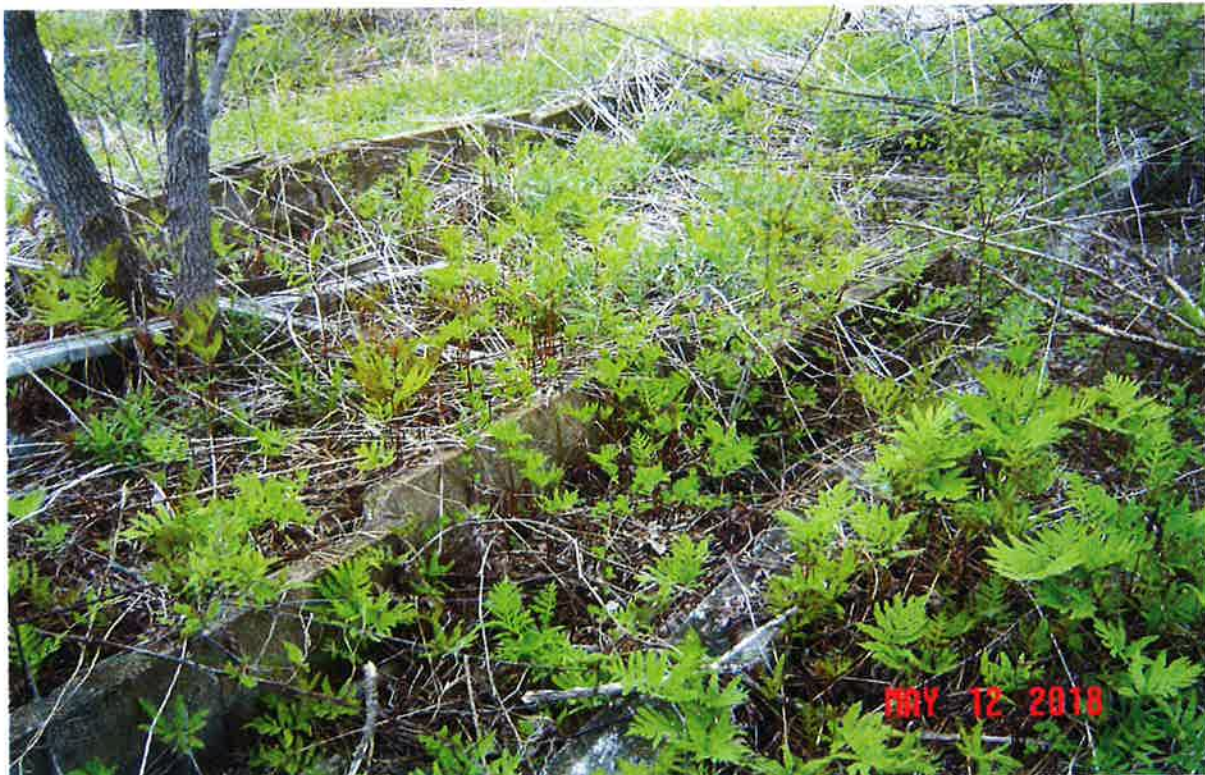
Image 8 – Looking northerly at man-made Wetland C. Note concrete slabs (typical). Refer to Figure 2. ©Jacobs2018
