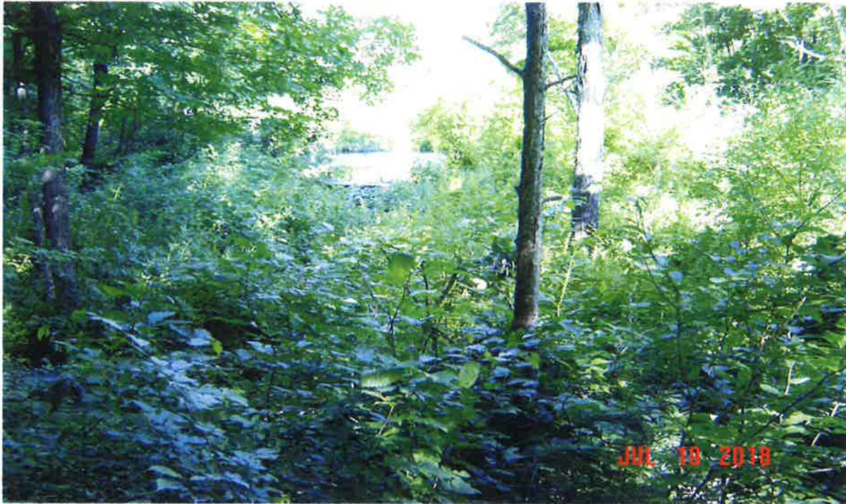
Image 1 - Looking westerly at the proposed Norris Brook 5' X 24' box culvert (Impact K1/K2) crossing from downstream. Note the concrete weir and pond in the background. Refer to Figure 1. ©Jacobs 2018
