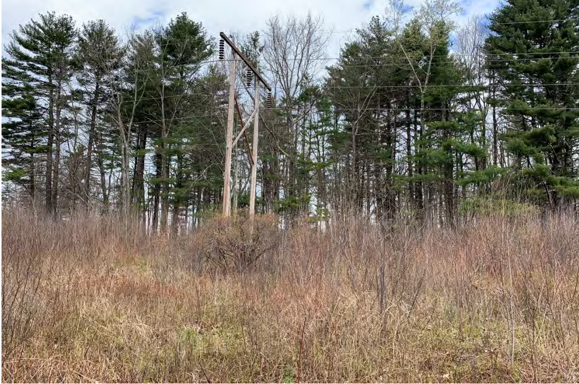
Photo 1. View northwest at existing Structure 202 proposed for replacement. Photo depicts the approximate location of temporary impacts within Wetland EW-1 and its associated 40' buffer resulting from timber matting and the structure work pad.
