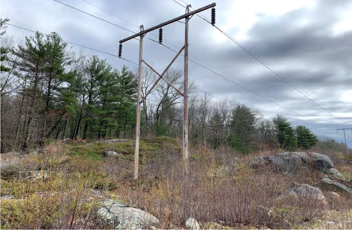
Photo 7. View northeast at existing Structure 166 proposed for replacement. Photo depicts approx. location of temporary impacts within the 40' wetland buffer of Wetland EW-23 located immediately west of the structure.
