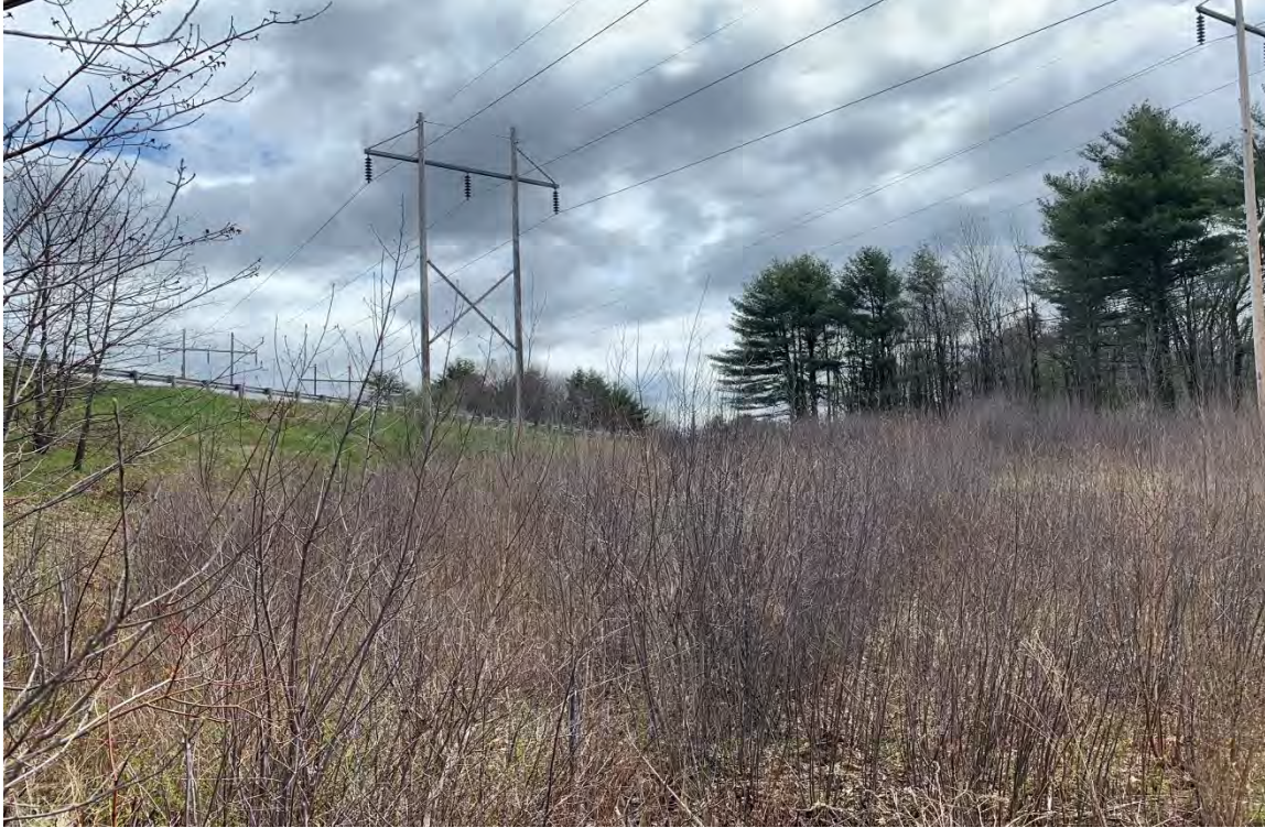
Photo 5. View southeast at existing Structure 200 proposed for replacement. Photo depicts approximate location of temporary impact to Wetland EW-2 and its associated 100' prime wetland buffer resulting from timber matting and the structure work pad.
