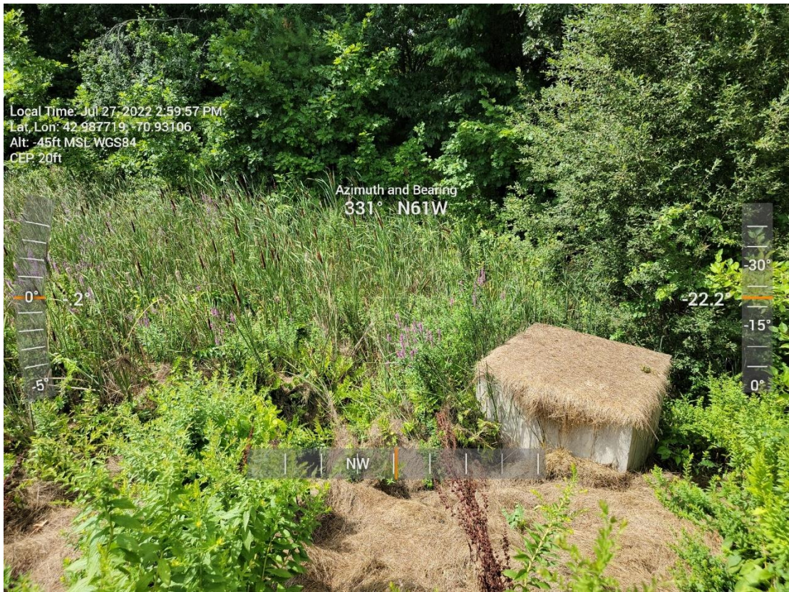
Photo: 5 – Detention-pond and outflow structure
