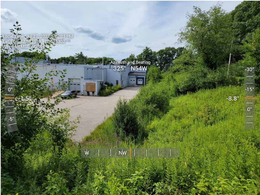
Photo: 3 – Low functioning, low value ditched area at toe of slope with invasive species.
