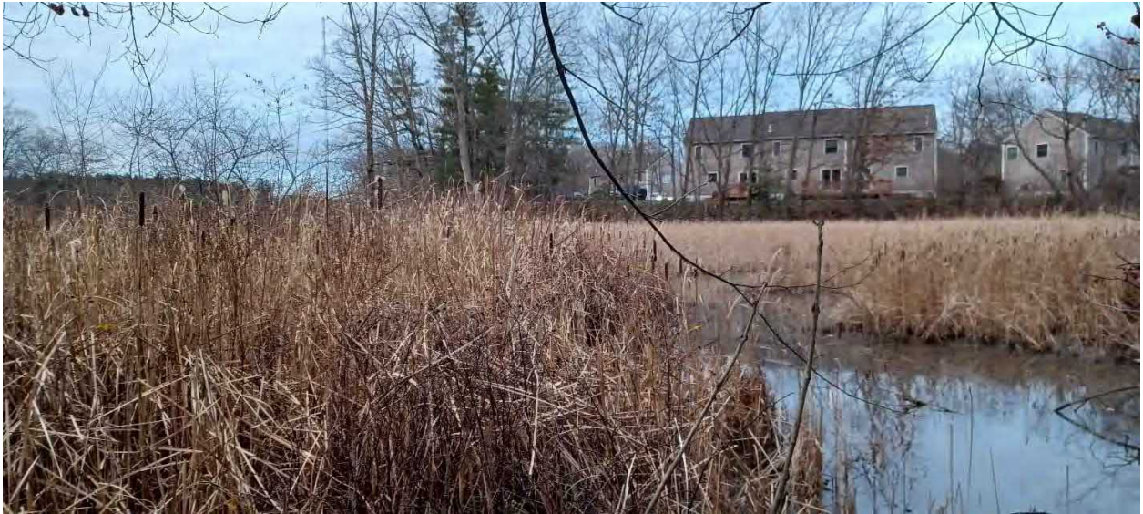
Photo 3: Taken facing northerly at the downstream side of the culvert under Webster Avenue. Note the residential buildings in the background.
