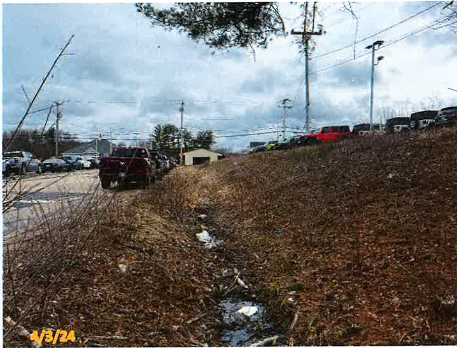
Photo 1-- Swale at beginning of GTE Road that will need to be crossed to provide access from adj. Foss Motors Site (Wetland B1)
