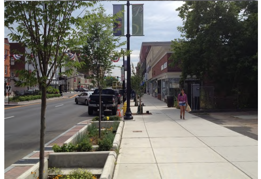
North Street before (top) and after (bottom) rain garden retrofits.
