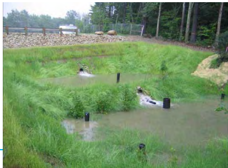
Figure 3. Gravel Wetland (Credit: UNH Stormwater Center)
