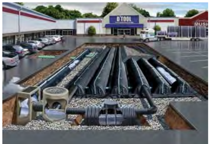
Figure 7. Subsurface infiltration at a commercial parking lot. (Credit: www.waterworld.com)
