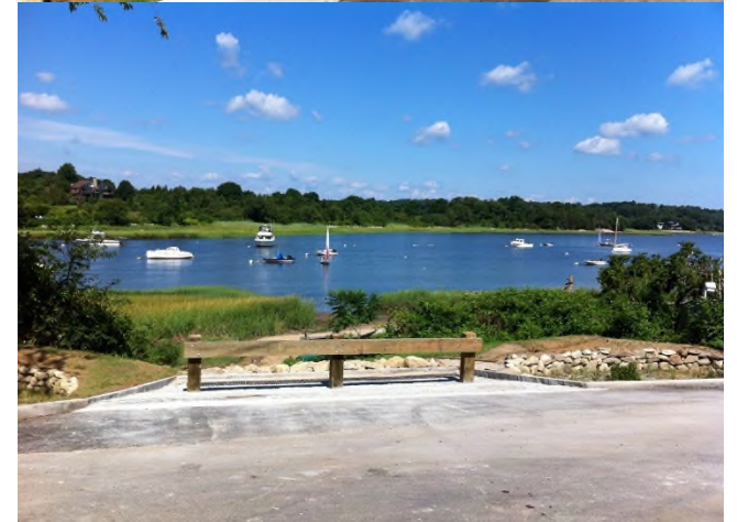
Rain garden off of Delano Avenue in Kingston, MA.
