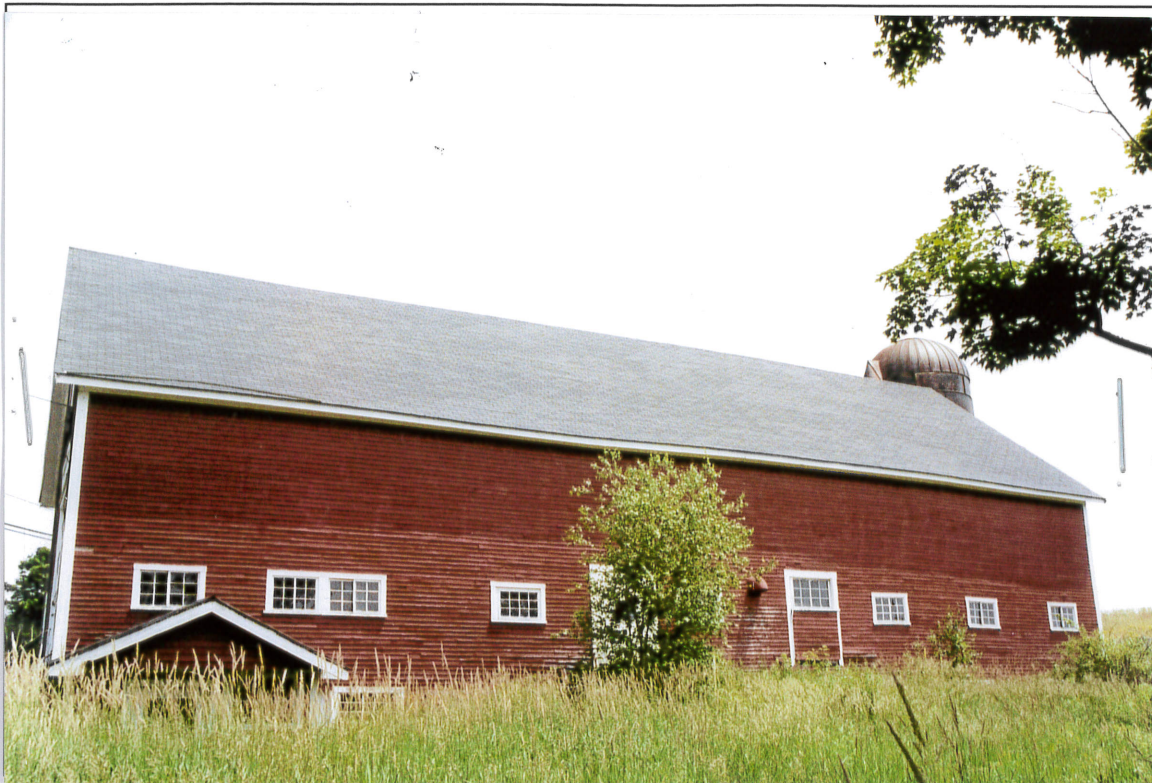
Photo # 9 Description: Milk Room Addition Removal (Before) Photo 9, Baseline 6:
