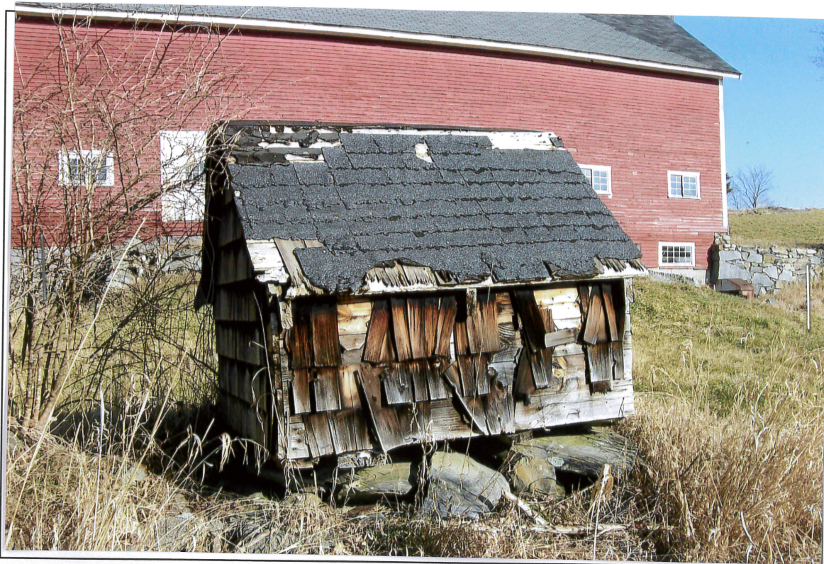
Photo # 11 Description: Well House (Before) Photo 11 Former Well House
