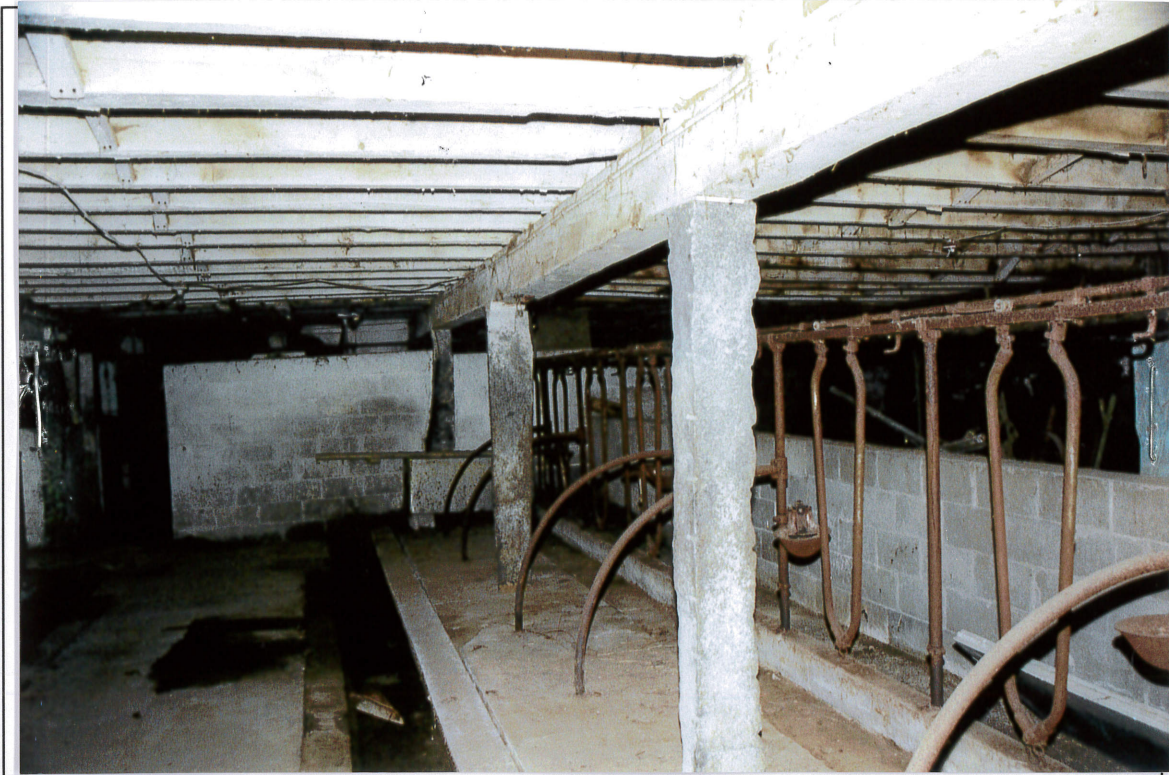
Photo # 7 Description: Replaced Columns (Before) Photo 7 Baseline 100
