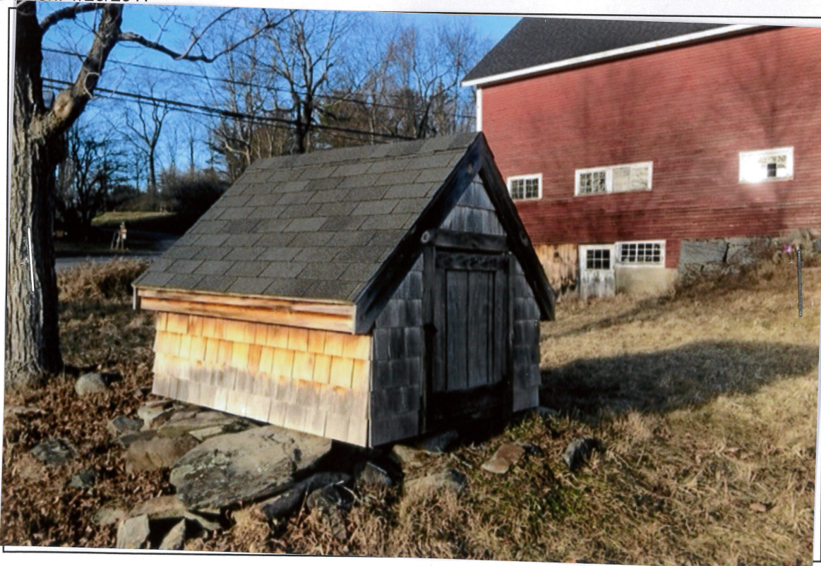
Photo # 12 Description: Well House (After) Photo 12 Replacement Well House:
