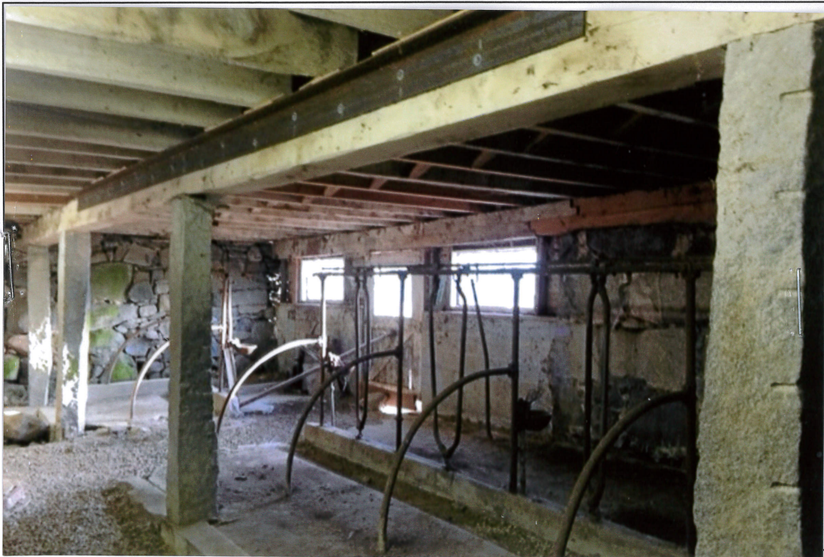
Photo # 8 Description: Replaced Columns (After) Photo 8 Replaced Columns:
