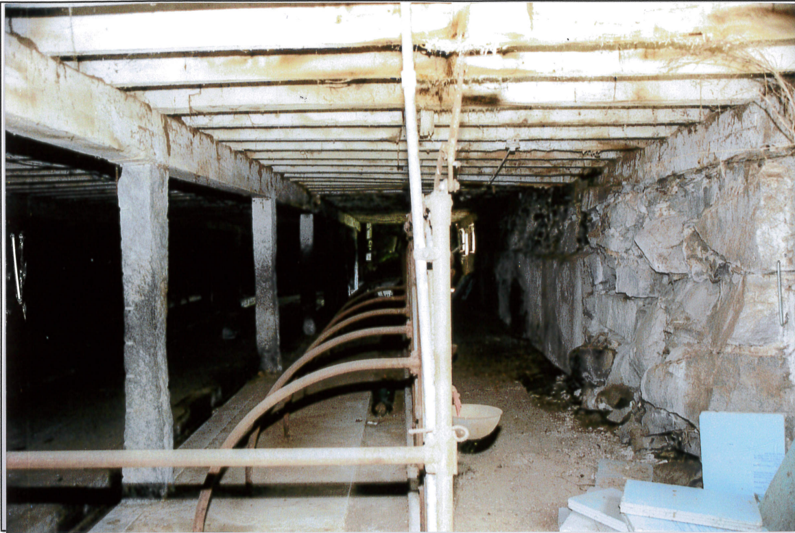
Photo # 5 Description: Sill Replacement (Before) Reference Photo 5 Baseline 99:
