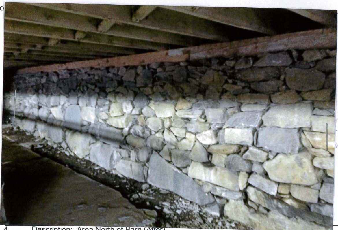
Photo # 4 Description: Area North of Barn (After) Photo 4 NW Foundation Repair:
