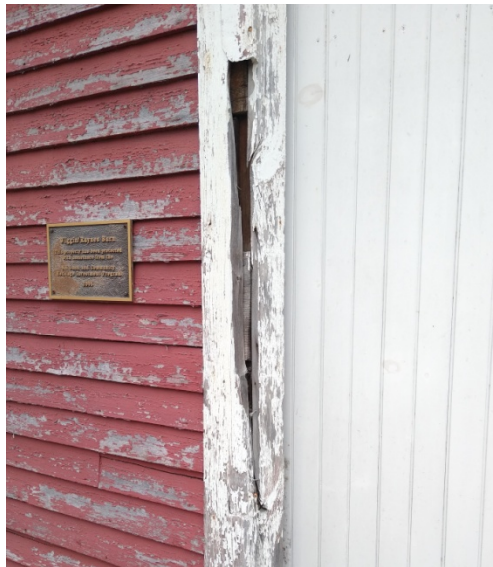
West Façade, trim on left side of barn door opening
