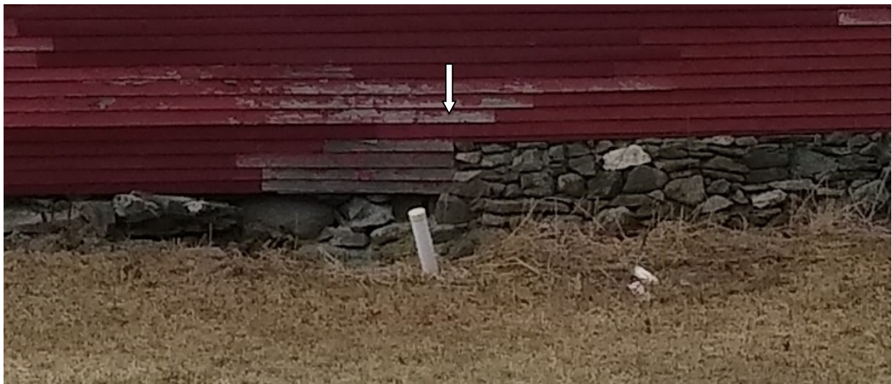
North foundation, sub-sill area about half way along north wall
