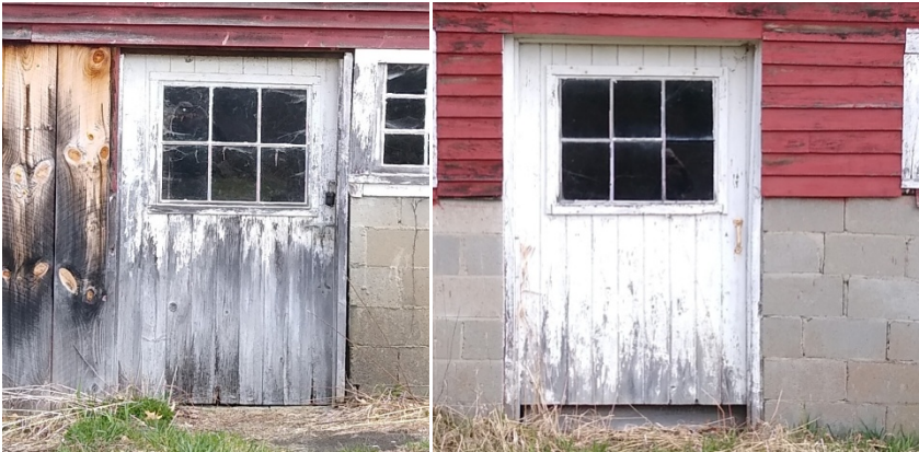
South side, westerly door
