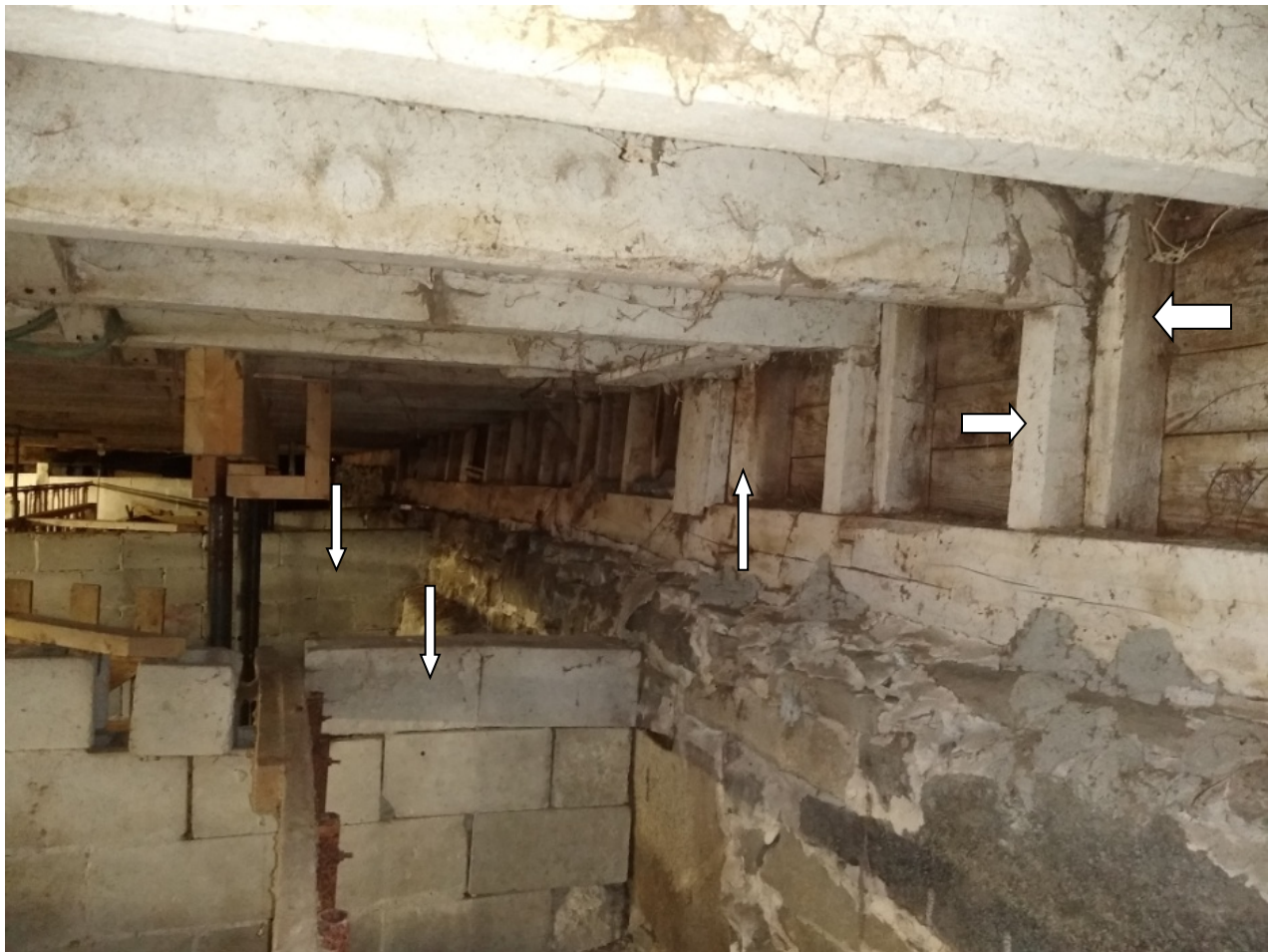
North sill and foundation wall (with “arrow” explanation below)
