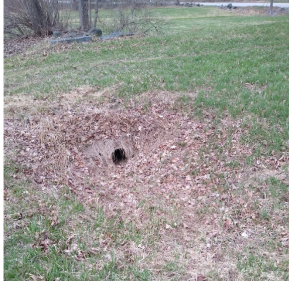
Culvert under east gable end earthen ramp.
