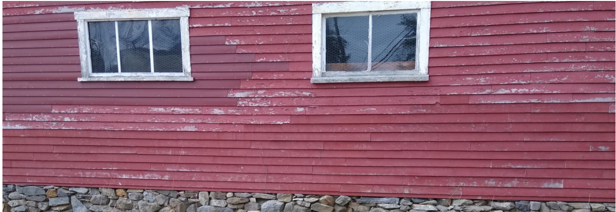
North side, easterly section showing clapboard replacement
