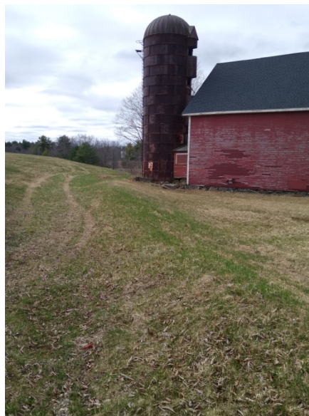
Grading along the north side, to help eliminate the slope/water pressure coming down the hill towards the barn
