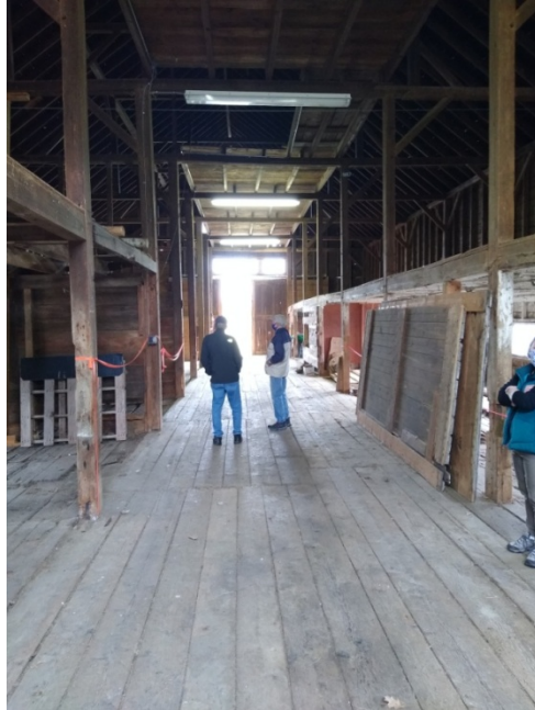
Barn center aisle looking east
