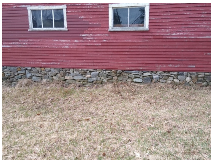
Westerly section of north foundation
