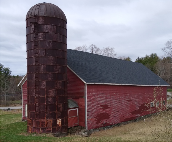
East side, connector and silo
