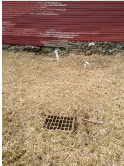
Catch basin and drainage along the north side of the barn
