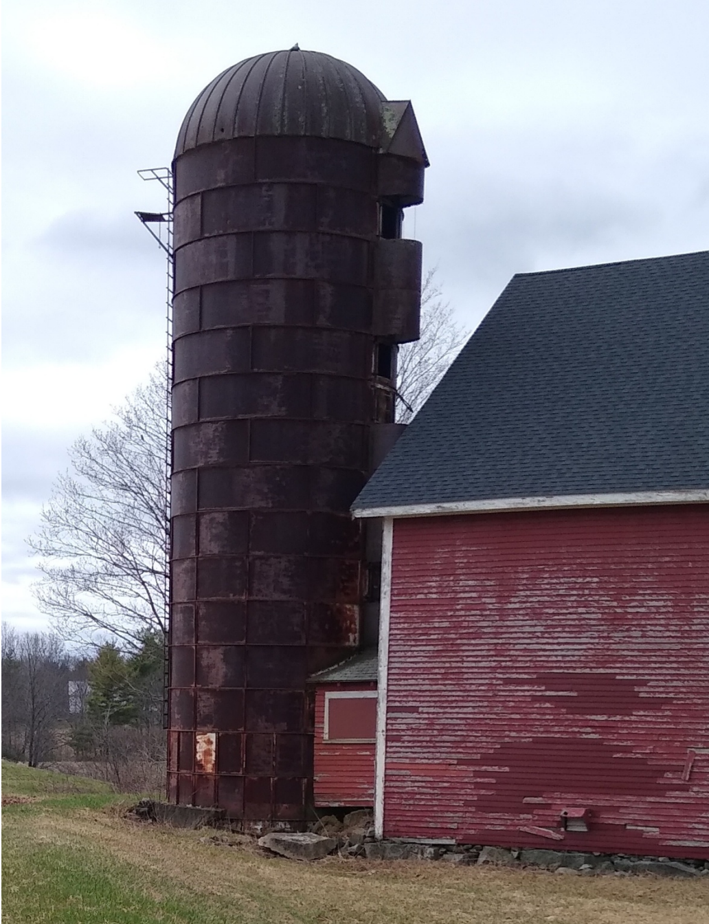
Left to right, south easterly view of silo, connector and barn
