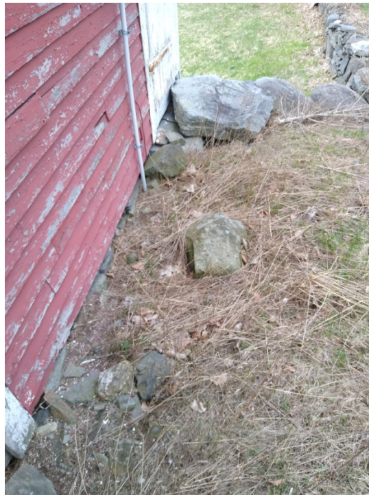
West façade looking southeast
