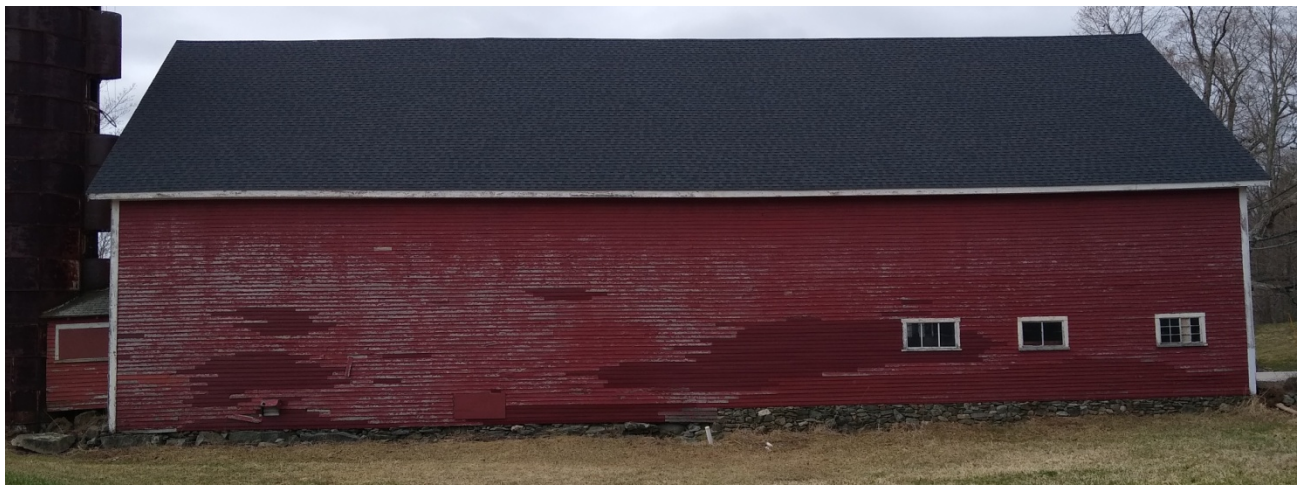
Foundation on north side
