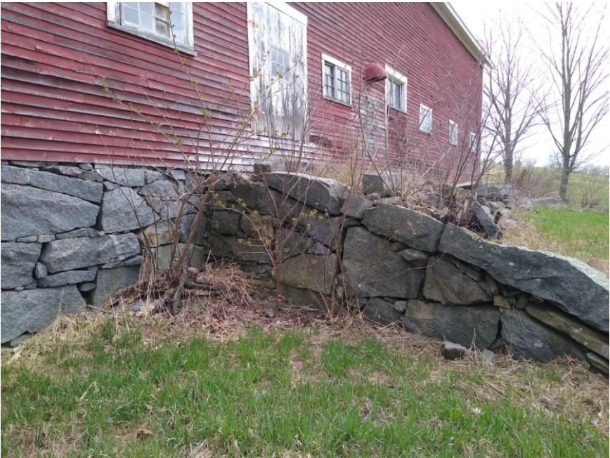
Western side of south side ramp with brush
