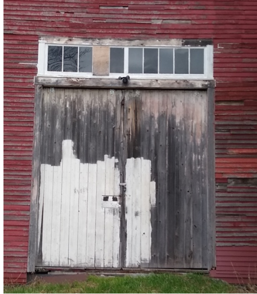
East side, large sliding doors
