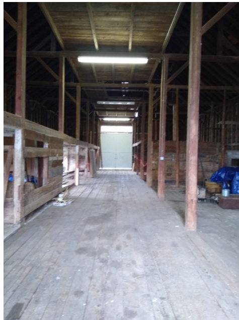
Barn center aisle looking west
