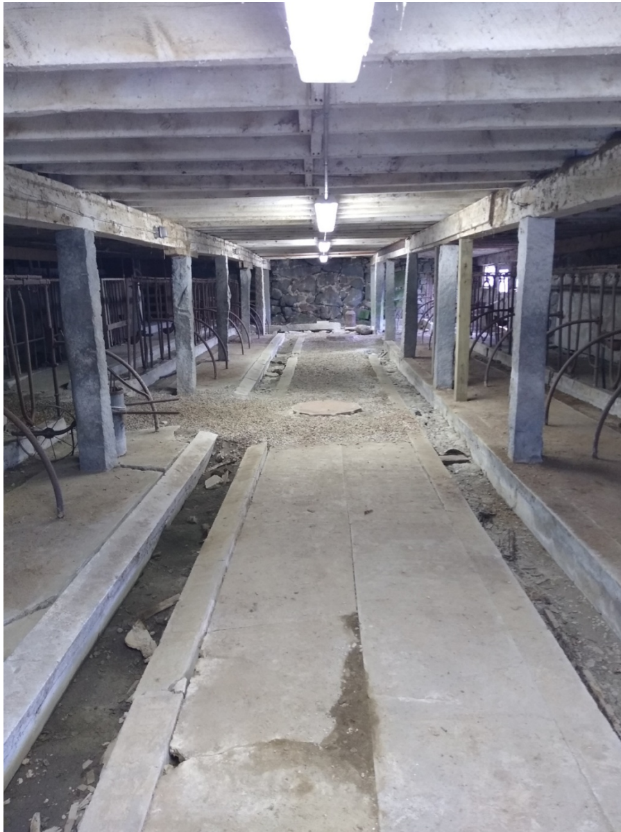
Looking east, lower level milking parlor remnants Please note the original granite posts that support the first floor main carriers
