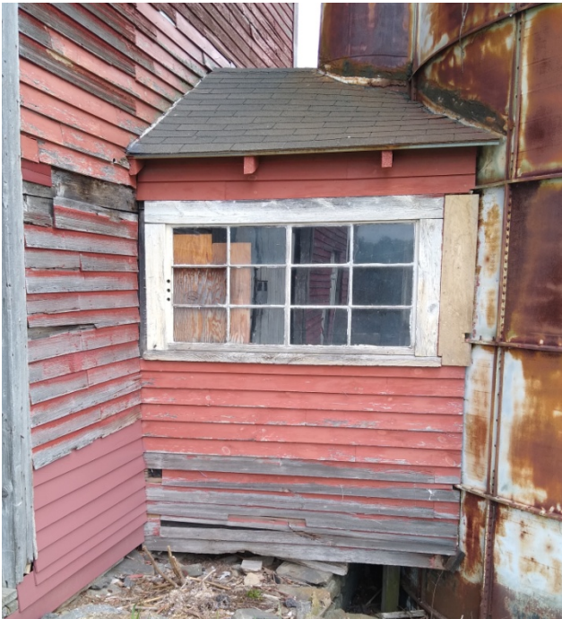
East side, southerly connector side
