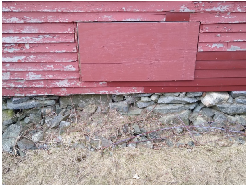
Easterly section of north foundation
