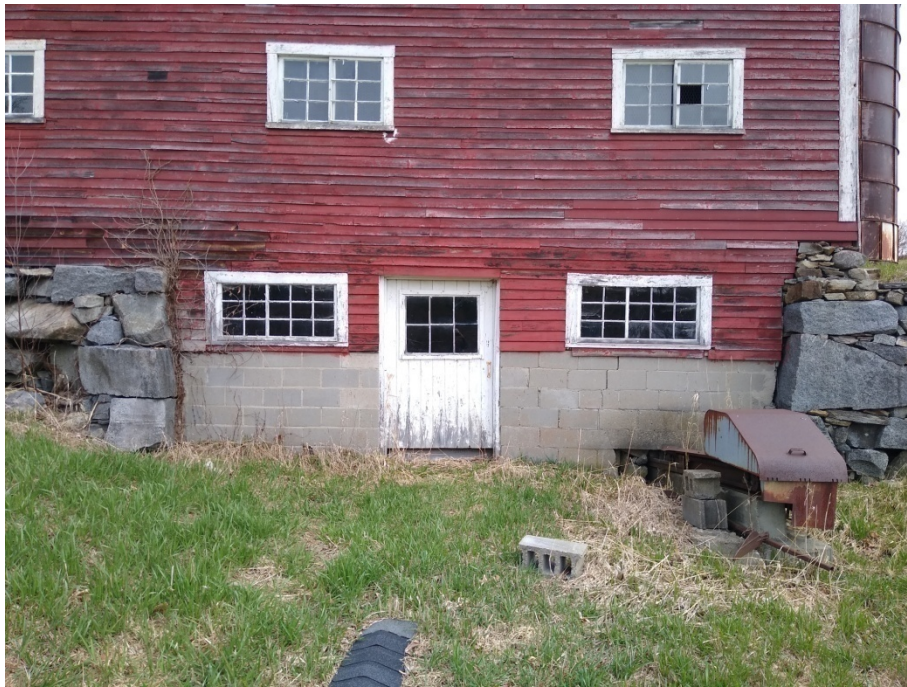
Easterly entrance into the lower level area on the south side
