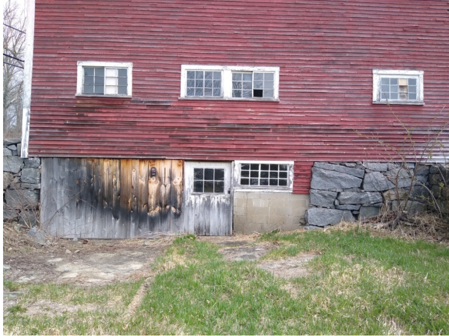
Westerly entrance into the lower level area on the south side
