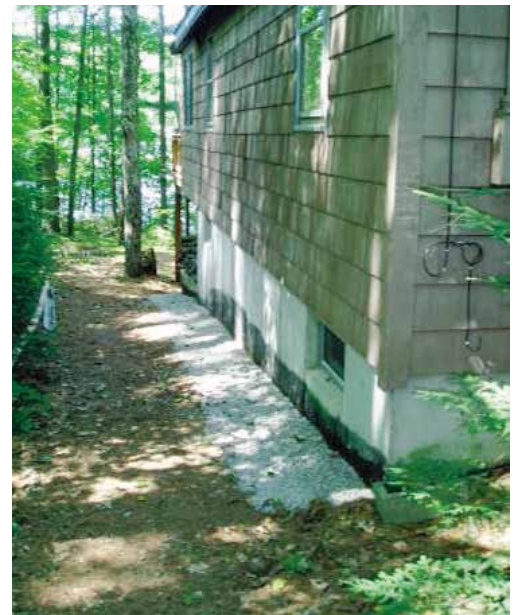
An infiltration trench was constructed to catch roof runoff at this lakeside home.
