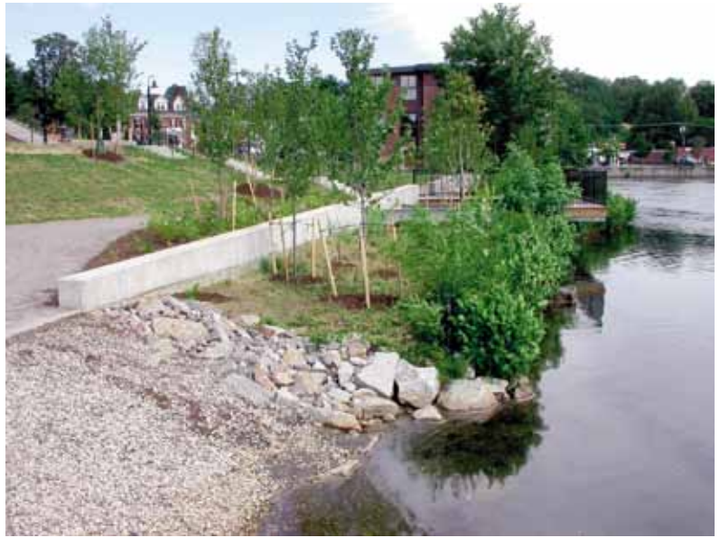
This 12-foot wide buffer is not adequate for the steeply-sloped property above it. The paved pathways provide a direct route for runoff water to enter the river.
