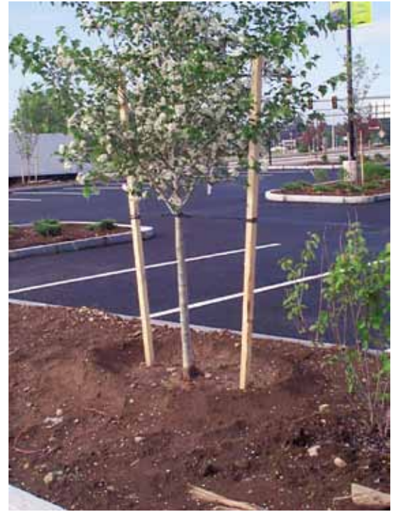
This tree on a commercial site has been properly planted and staked with flexible ties. The next step is to add mulch 2-3 inches deep over the entire bed, but keeping it away from the trunk.
