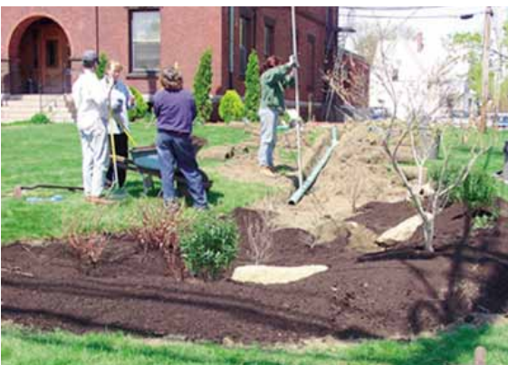
Demonstration rain garden being installed in Kingston, Rhode Island. At right, puddles remain in the road after a heavy rain but the runoff from the landscape has already infiltrated the soil in the rain garden.
