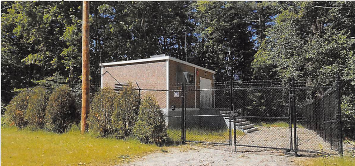
Stadium Well pumping station
