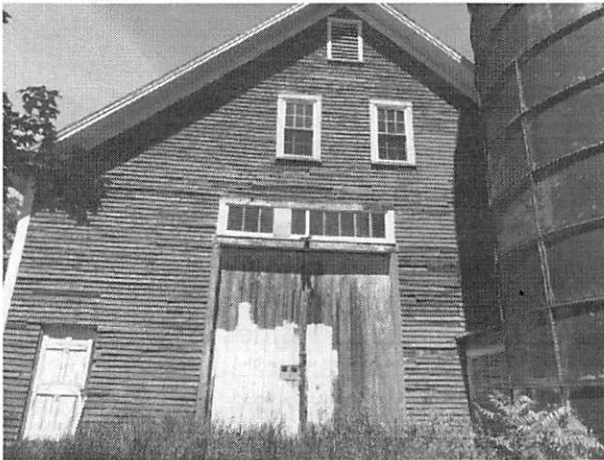
Windows, Doors, Clapboards
