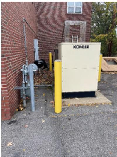
**Figure 16 – Unsecured utilities and backup generator**
