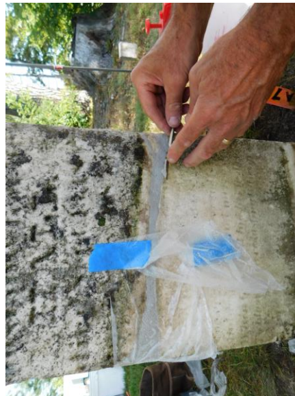
7. EWSC. A71. DT. Filling losses along break-line with Jahn M120.
