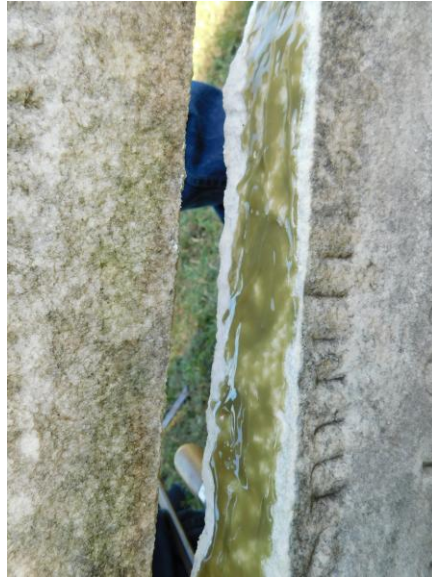
4. EWSC. A104. DT. Detail of mating surfaces with epoxy.
