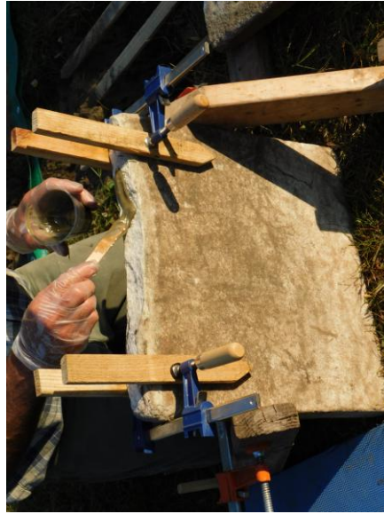
4. EWSC. A126. DT. Application of epoxy for repair.
