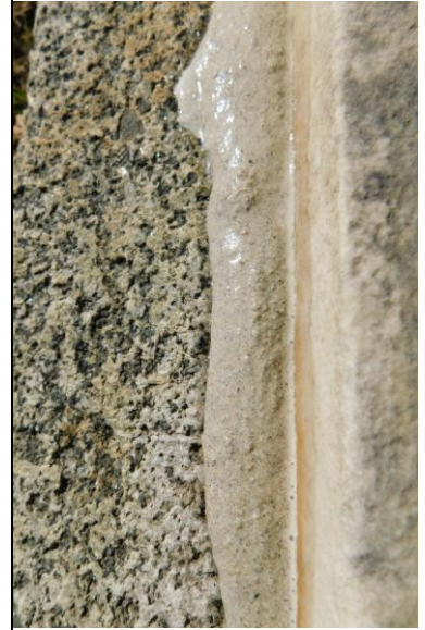
12. EWSC. A109. DT. Detail of mortar extruding from below marble.
