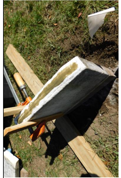
5. EWSC. A71. DT. Epoxy application on bottom stone.
