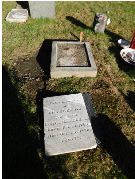
10. Marble prior to setting in mortar bed on granite base.
