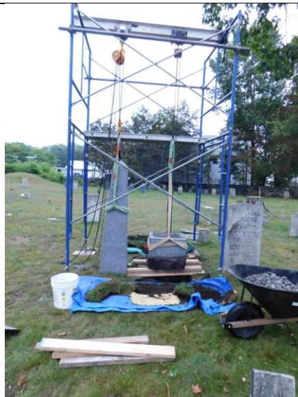
EWSC D53 3. During Reset. Detail of base set in concrete.
