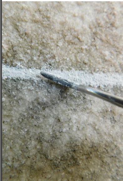
12. EWSC. A104. DT. Detail of break-line during fills.
