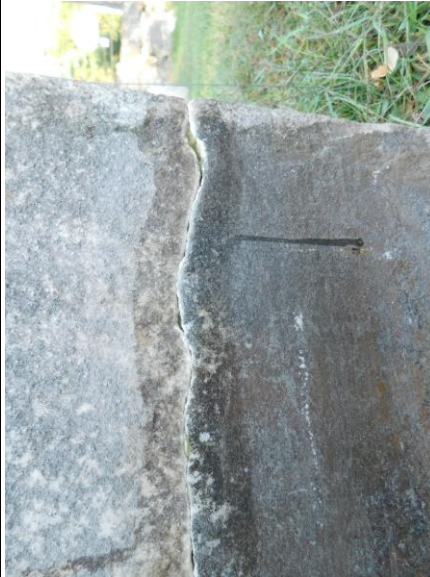
7. EWSC. A104. DT. Release on marble faces and epoxy filling crack.
