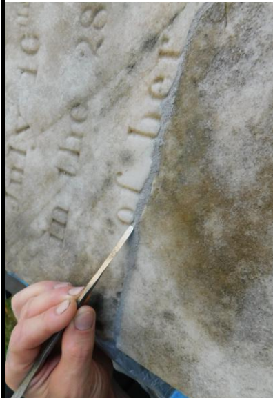
12. EWSC. A108. DT. Mortar fill along break-line.
