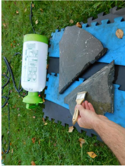
4. EWSC. A145 FS. DT. Cleaning slate with ReVive.
