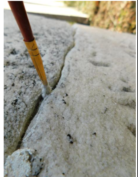
8. EWSC. A76. DT. Wetting break-line with Jahn mortar slurry.
