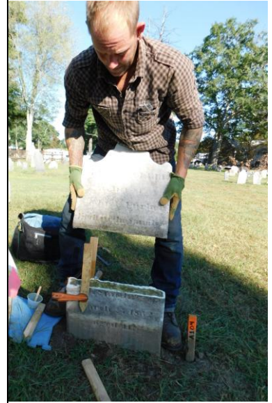
5. EWSC. A104. DT. Joining stones with epoxy.
