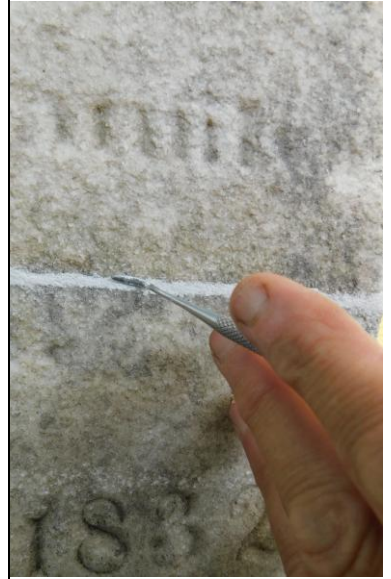
11. EWSC. A104. DT. Break-line during fills.
