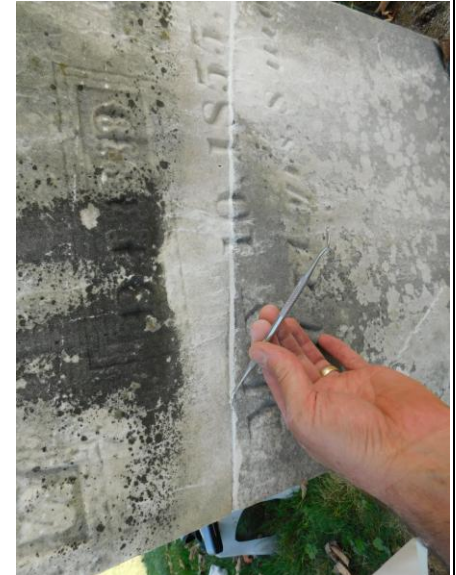
14. EWSC. B71. DT. Application of Jahn mortar in break-line mend.
