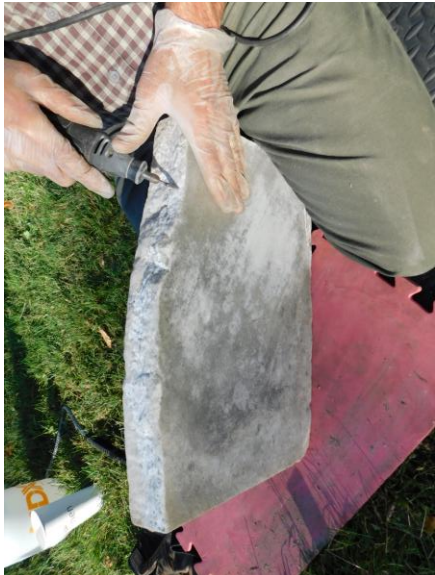
12. EWSC. B71. DT. Removal of failed adhesive on break-line with Dremel.
