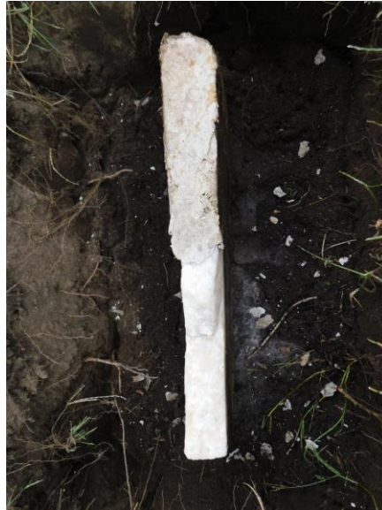
4. EWSC. A76. DT. Removal of failed adhesive.
