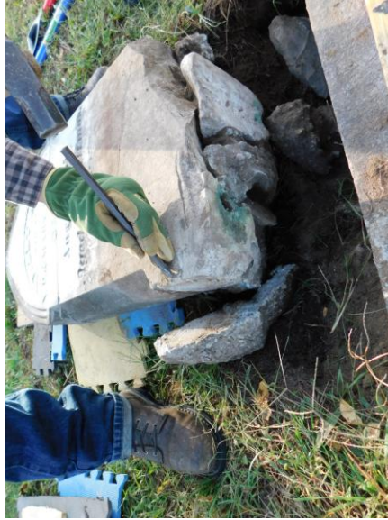
5. EWSC. A30. DT. Removing concrete and marble fragments around marble.
