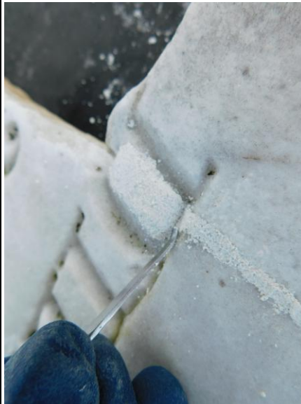
7. EWSC. A93. DT. Detail of filling losses with Jahn mortar.
