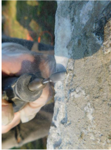
5. EWSC. A29. DT. Removing failed adhesive mortar at break-line.
