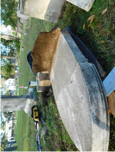
4. EWSC. A30. DT. Concrete poured around marble.
