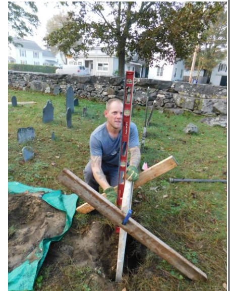
8. EWSC. A126. DT. Setting marker plumb.
