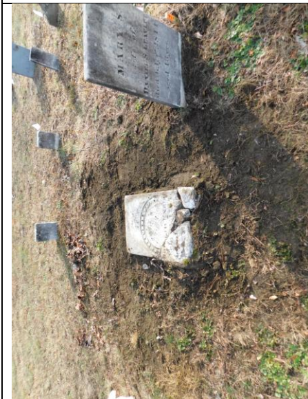
EWSC A39 7. During Reset. Braced marble in concrete base.
