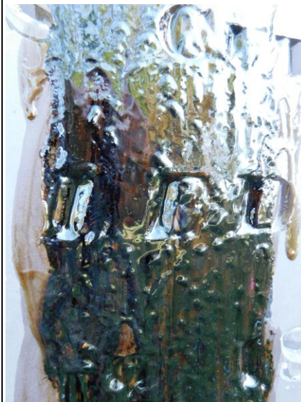
20. EWSC. F80. DT. Application of stripper after scrapping, detail.
