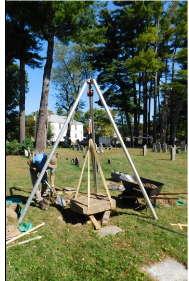
6. EWSC. A109. DT. Removal of base for crushed stone bed.
