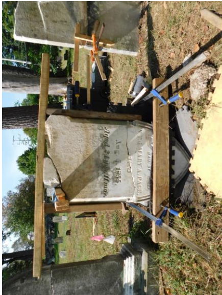
7. EWSC. A30. DT. Aligning fragment for coring pins.
