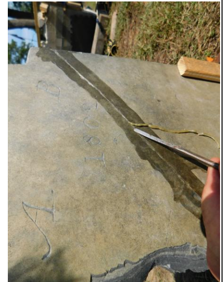
9. EWSC. A145 FS. DT. Removal of excess epoxy prior to full gel.
