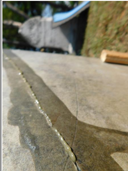
8. EWSC. A145 FS. DT. Detail of excess epoxy and resist.
