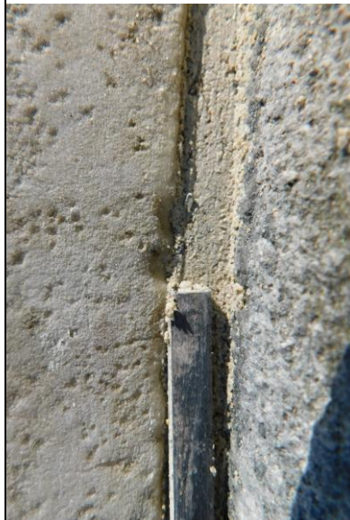
13. EWSC. A93. DT. Detail, pointing the edges of the mortar joint.
