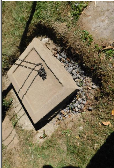
7. EWSC. A109. DT. Setting granite base on crush stone.
