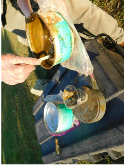
3. EWSC. A126. DT. Mixing epoxy for repair.
