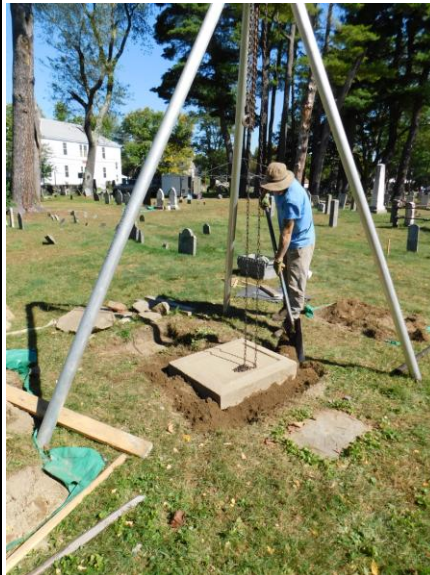
8. EWSC. A109. DT. Packing earth around the granite.
