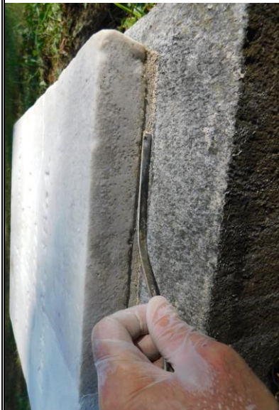
12. EWSC. A93. DT. Pointing the edges of the mortar joint.
