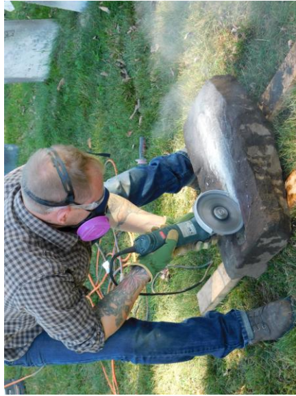
4. EWSC. B71. DT. Removing marble in mortise.
