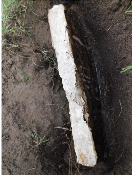
3. EWSC. A76. DT. View of lower portion with failed adhesive.
