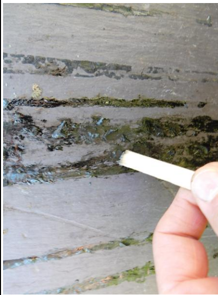
8. EWSC. F80. DT. Detail of scraping tar on back removal test.
