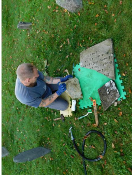
3. EWSC. A82. DT. Cleaning the marble sections with ReVive.
