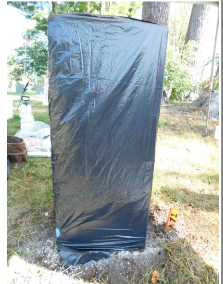
8. EWSC. A71. DT. Marker covered with plastic for mortar cure.
