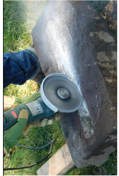
5. EWSC. B71. DT. Removing marble in mortise with diamond wheel.
