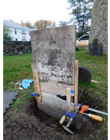
6. EWSC A22. DT Mending stone with epoxy.
