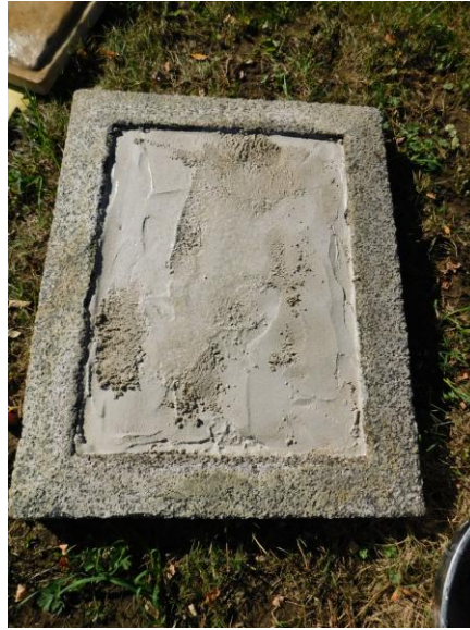
11. EWSC. A109. DT. Overview of granite ready for setting in mortar.
