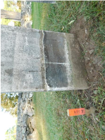
6. EWSC. A104. DT. Stone mended. Note release on marble faces.
