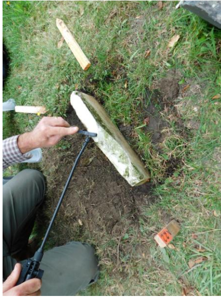
5. EWSC A22. DT Cleaning mating sections.
