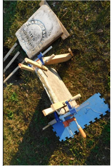
5. EWSC. A126. DT. .Epoxy applied to lower stone.
