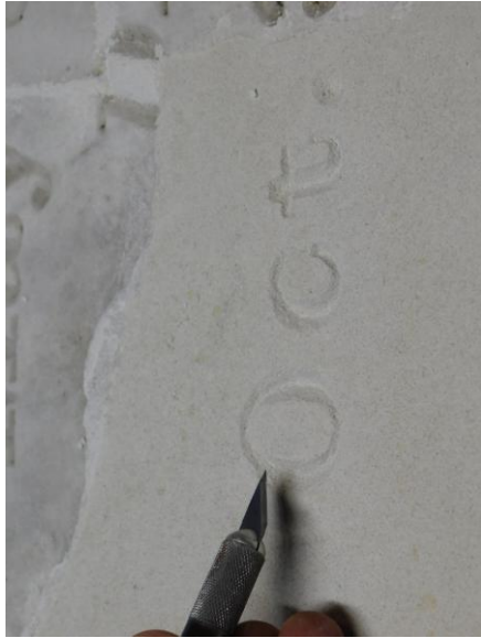
9. EWSC. A93. DT. Carving text in replacement element.
