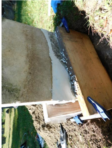
8. EWSC A22. DT Loss replacement with Jahn 120.
