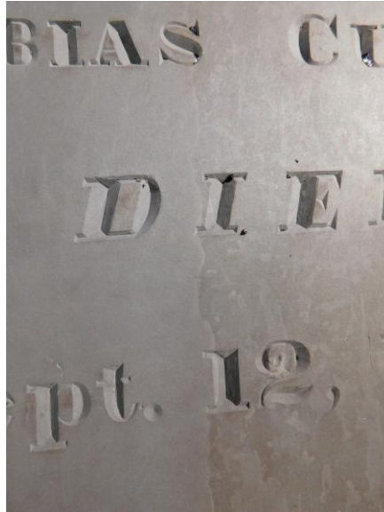
23. EWSC. F80. DT. Small tar accumulations in carving detail.
