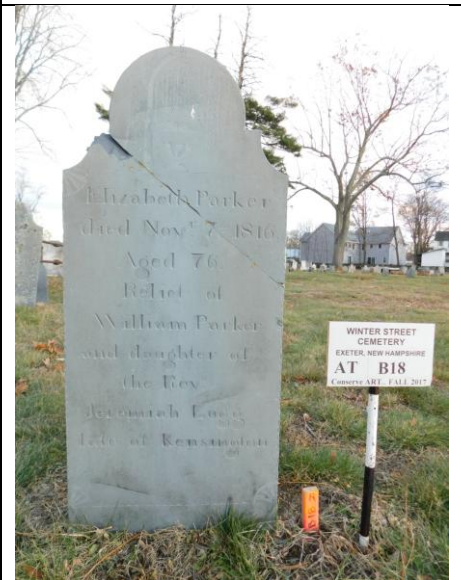
EWSC A135 1. During Reset. Compromised marble set on gravel for better drainage.
