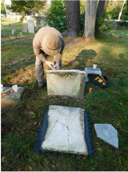
4. EWSC. A29. DT. Removing failed adhesive mortar at break-line.
