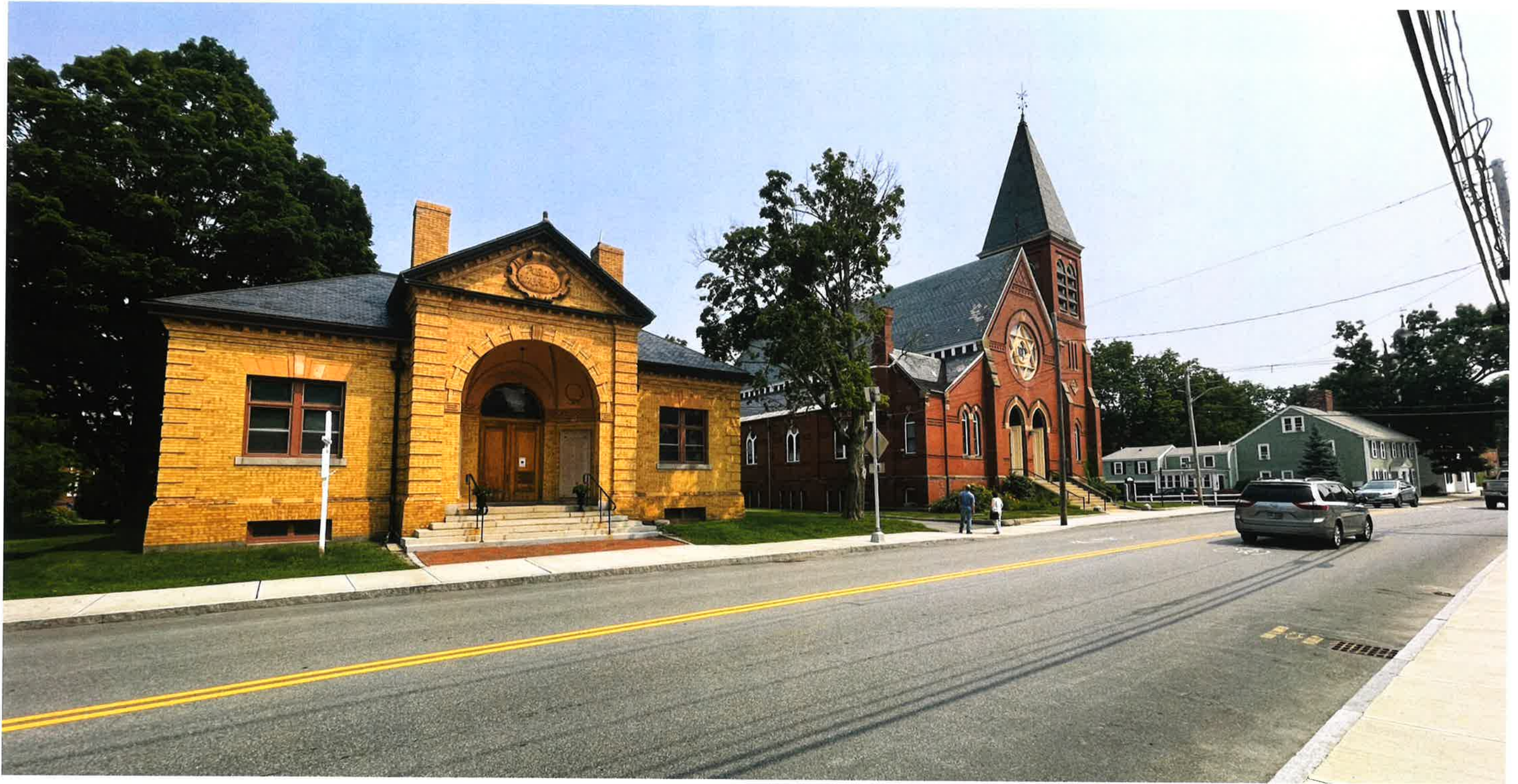
Existing Photo From Northwest Corner
