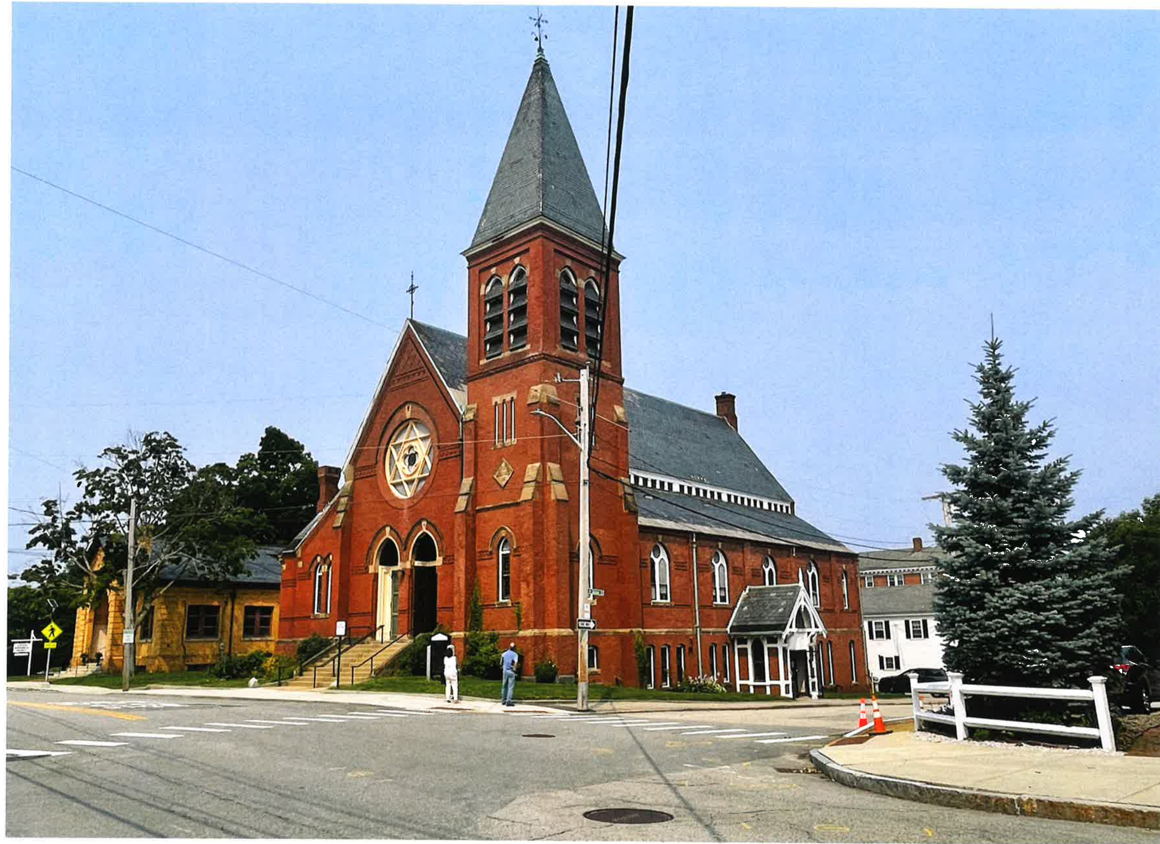
Existing Photo From Southwest Corner
