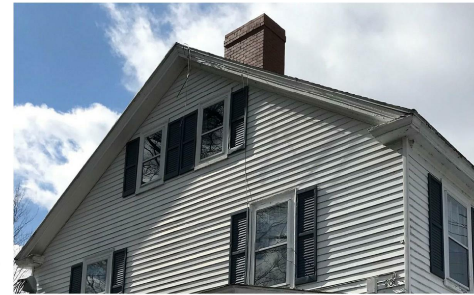
EXISTING GABLE END @ 55 HIGH STREET
