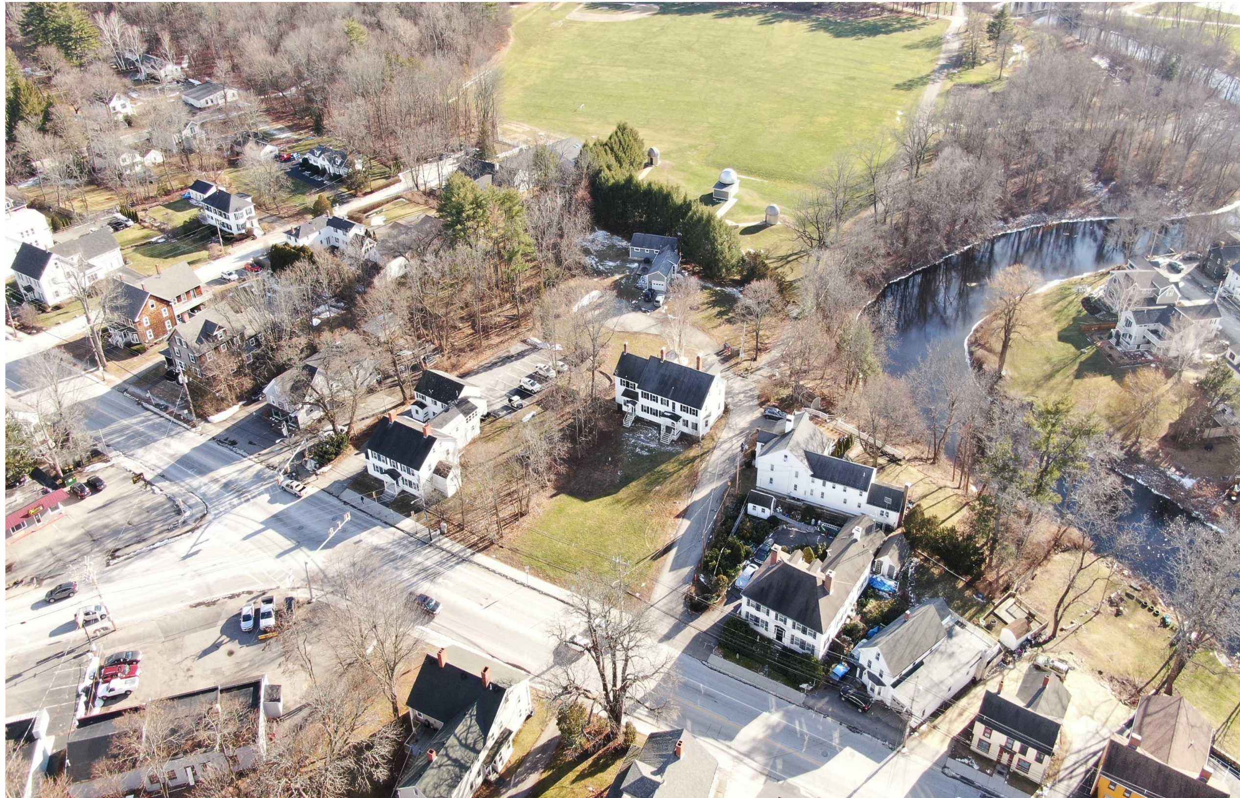
Existing Condition - View looking southeast
