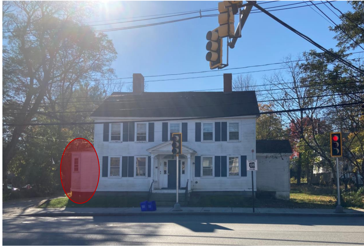
35 High Street – Partial Demolition
